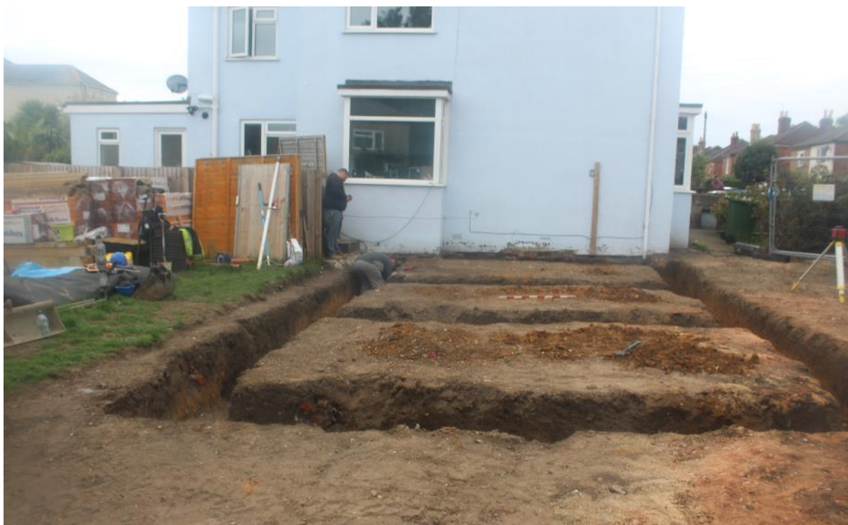
Plate 1. Overview of the Site. Taken looking south with a 1m scale.
