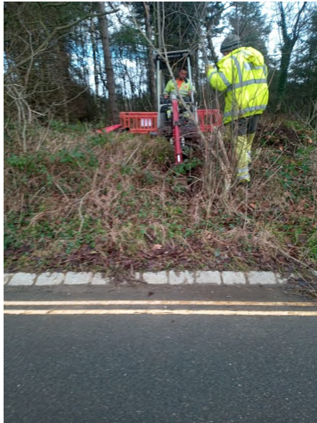
Plate 1- Watching brief area, view NE. View north-east.
