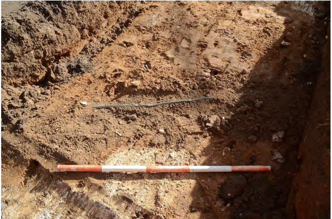
Plate 7: Trench 2, service pipe, view South
