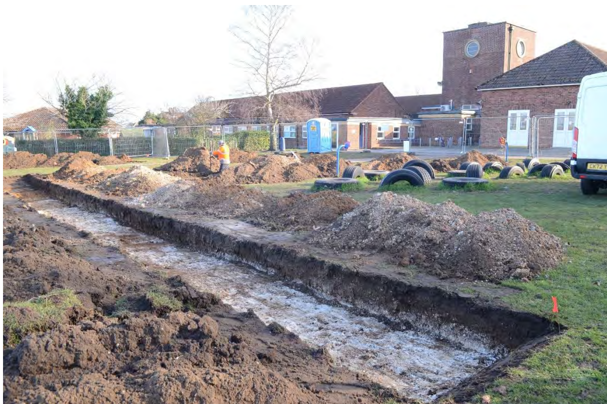
Plate 2: Excavation of trenches in progress, view SSE (Trench 1 in foreground)
