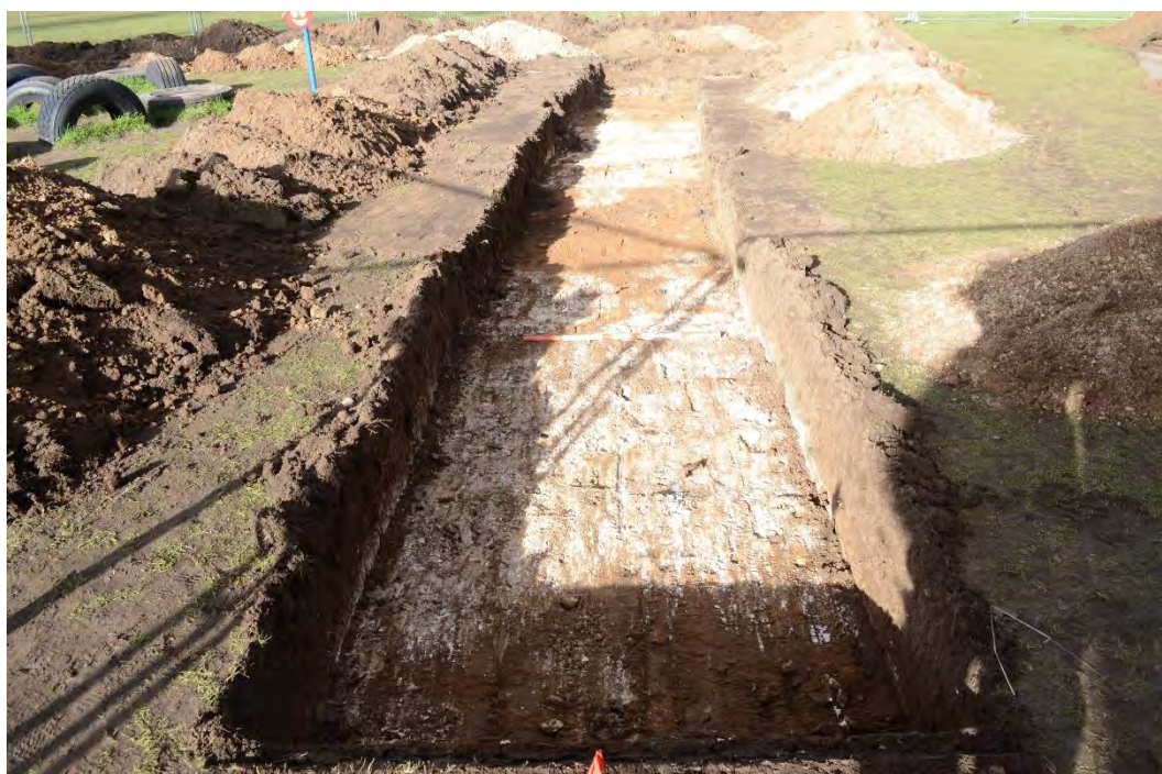
Plate 4: Trench 2, view North
