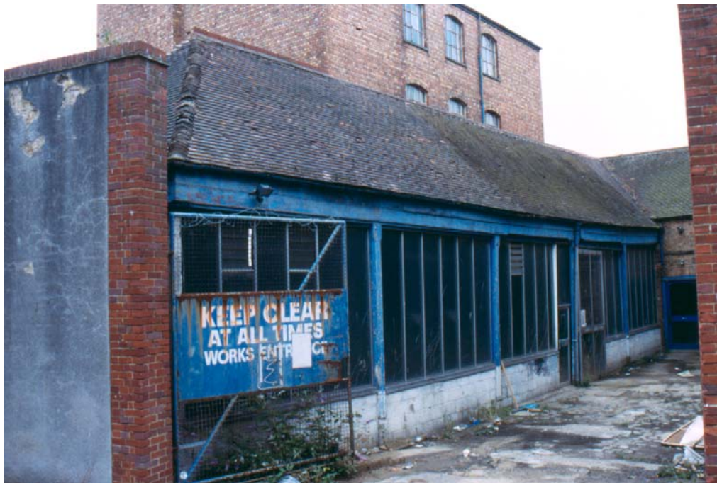
Plate 6: Building 4, West Facing Elevation
