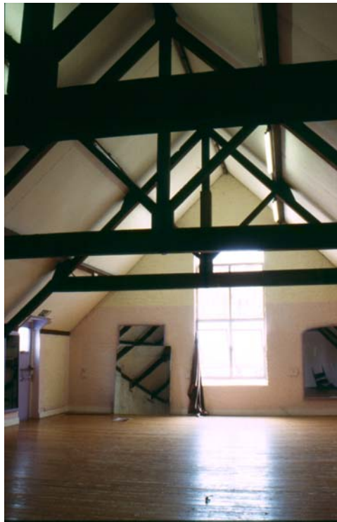
Plate 5: Building 3: Third Floor
