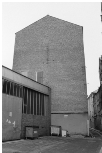
Plate 1: Building 2, South Facing Elevation
