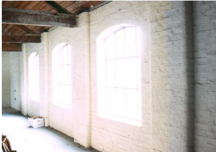
Plate 3: Building 2, Fourth Floor
