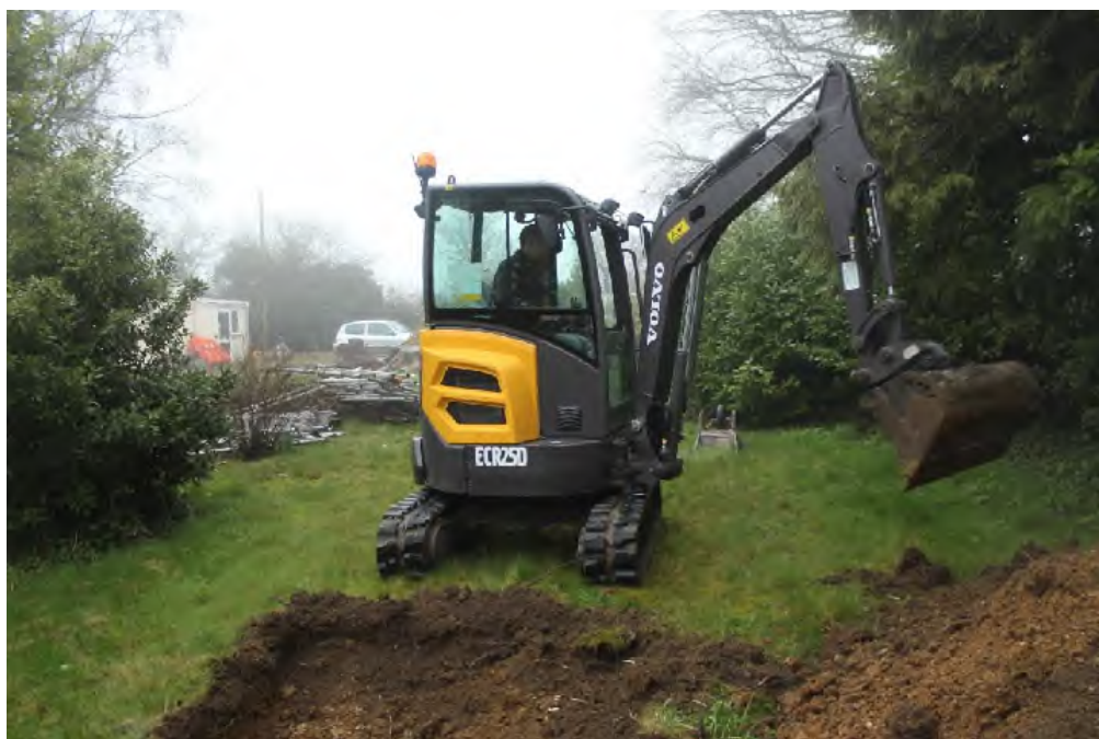
Plate 1: Trench 1, machining, view north
