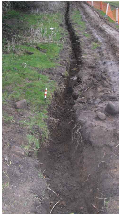
Plate 12: Cable trench continuing north-eastwards from Trench 2, looking north-east ( scale 0.5m )
