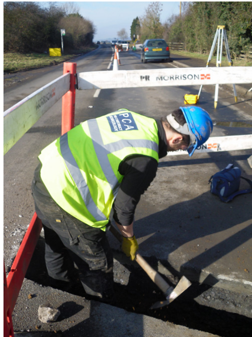
Plate 5: Trench 1a working shot, looking north-west
