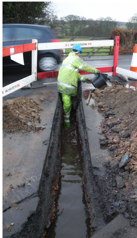
Plate 6: Trench 1b working shot, looking north-east
