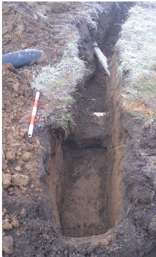
Plate 14: Trench 3 and cable trench continuing, south-westwards, looking south-west ( scale 0.5m )
