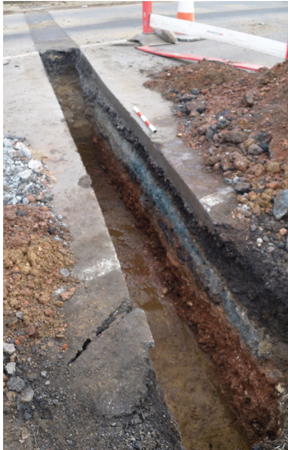
Plate 10: Trench 1b, modern intrusion [36] in Section 1b, looking east ( scale 0.5m )
