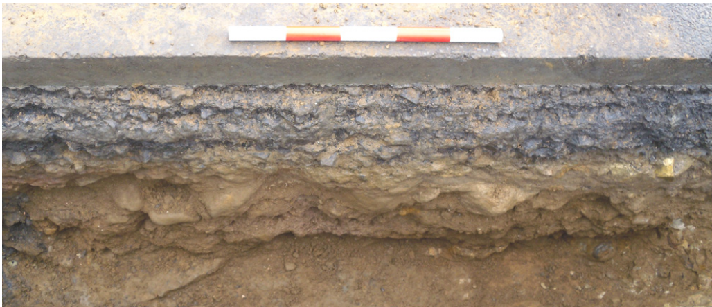
Plate 4: Trench 1a, south-western extent of Section 1a, looking south-east ( scale 0.5m )
