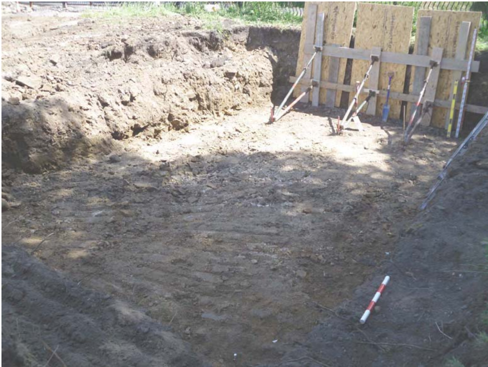
Plate 8: Overview of Sub-station footprint, looking north-east ( scale 0.5m )
