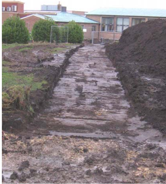
Plate 3: Overview of MUGA footpath during topsoil strip, looking south-west
