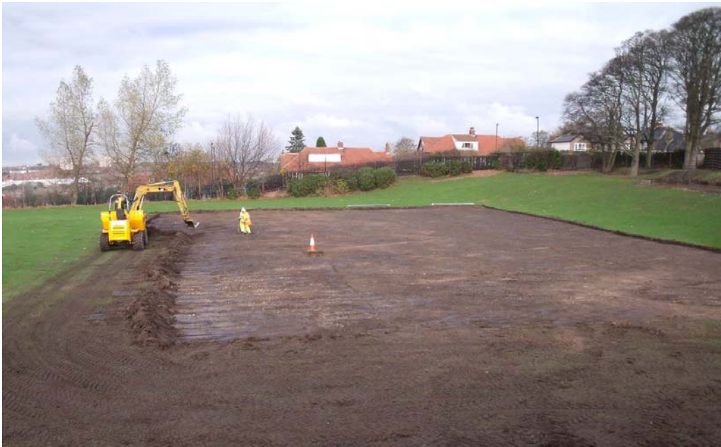
Plate 2: Overview of MUGA during topsoil strip, looking north
