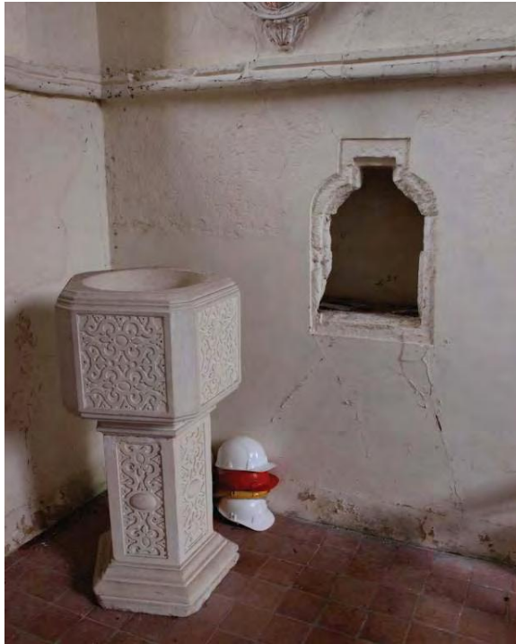
Plate 31. South east corner of the chancel showing string course, piscina and 20 th century font.
