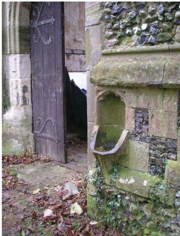
Plate 24. Detail of the stone stoup on the south side of the entrance in the west elevation.
