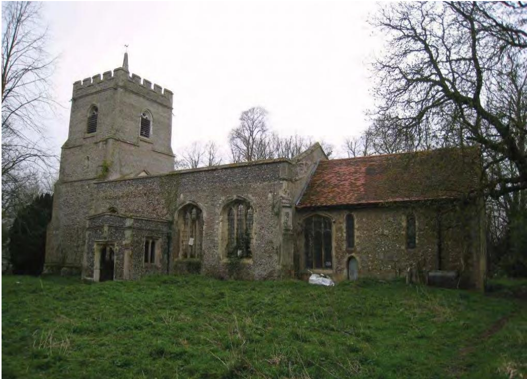
Plate 15. South elevation of St. Bartholomew's church.
