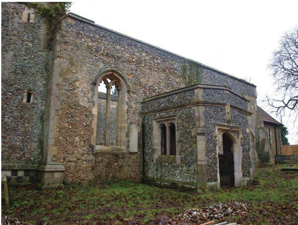
Plate 16. Porch and south side of nave.
