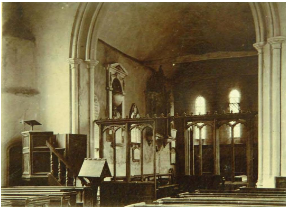
Plate 2. View of the chancel with timber screen and previous roof structure (pre 1904).
