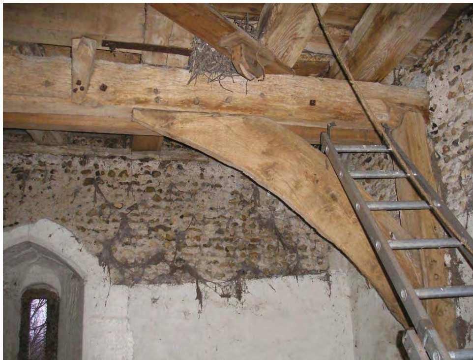
Plate 44. First floor tower room showing window and beams supporting belfry above.
