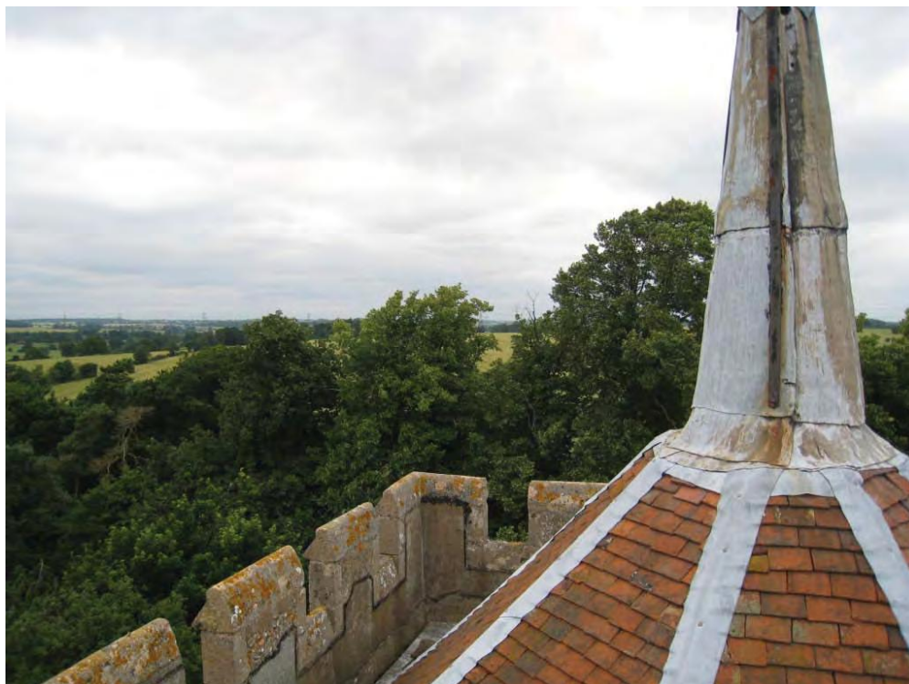
Plate 28. Octagonal roof with lead covered spike.
