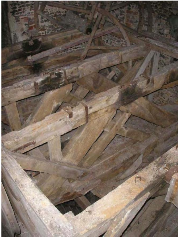
Plate 47. Bell frames after the bells had been removed.
