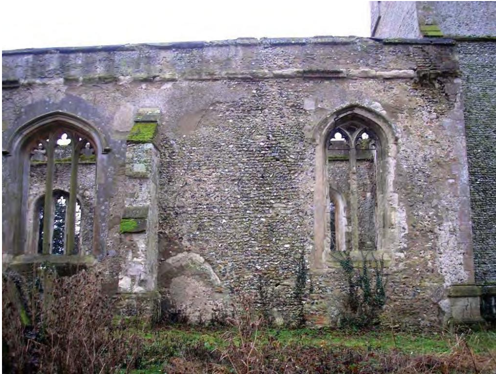
Plate 17. North elevation of the nave with parapet string course not seen on south elevation.
