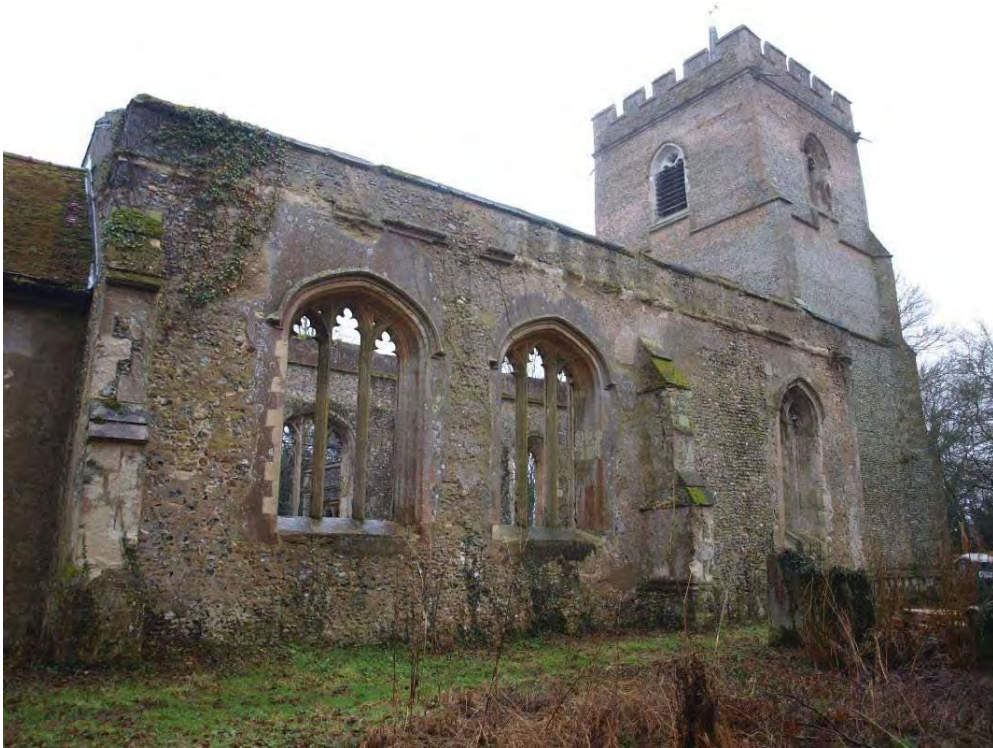
Plate 17. North elevation of the nave with parapet string course not seen on south elevation.
