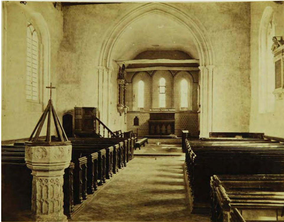
Plate 1. Nave and chancel with previous roof structure and timber tie beams. The end wall also shows evidence of painted decoration (pre 1904).
