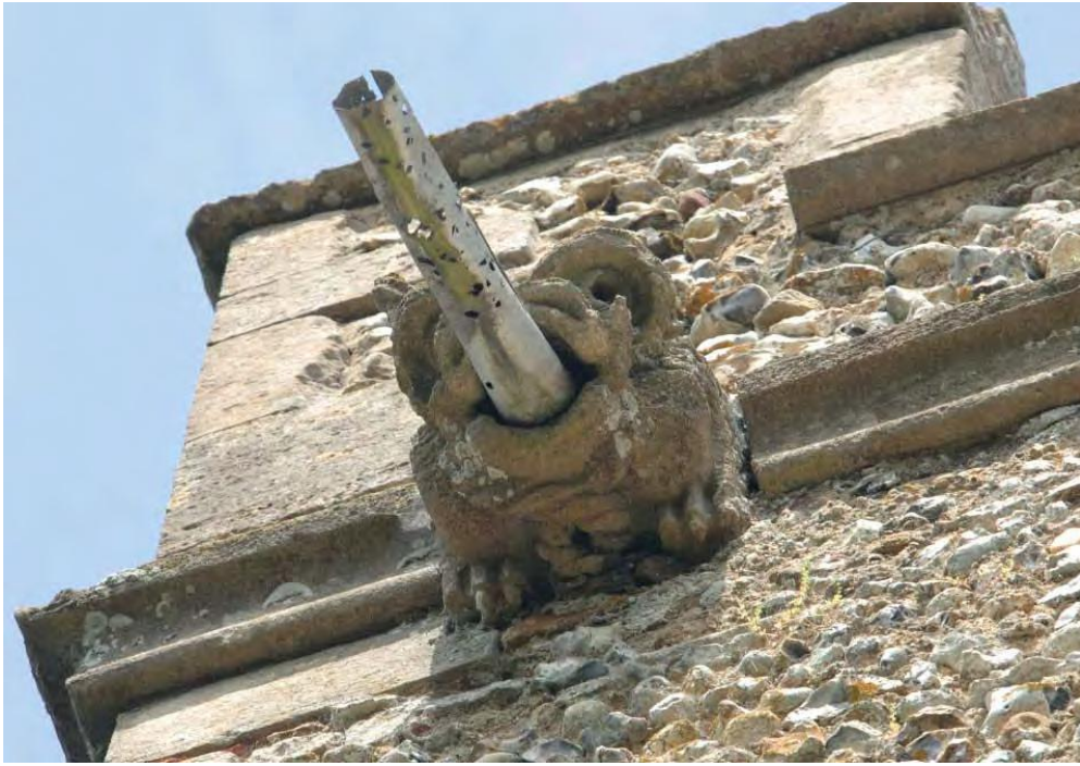
Plate 21. Carved stone gargoyle with water spout from tower roof.
