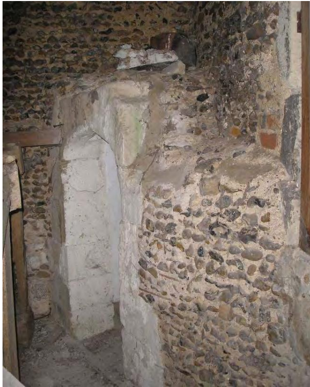
Plate 45. Entrance doorway to belfry from spiral staircase.
