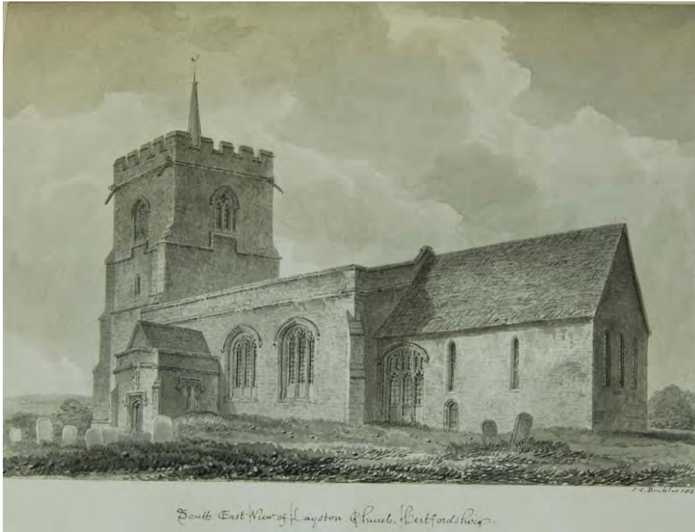
Figure 11 J.C. Buckler's illustration of south and east elevations of St Bartholomew's church 1831, showing previous porch, chancel roof and nave parapet.
