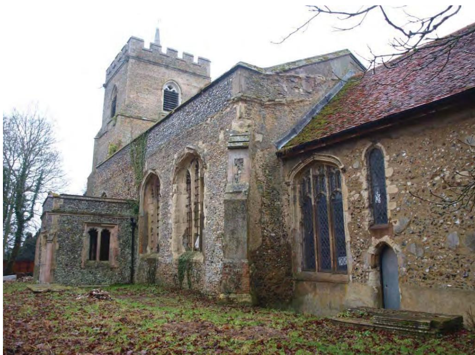
Plate 14. South elevation of the chancel and nave.
