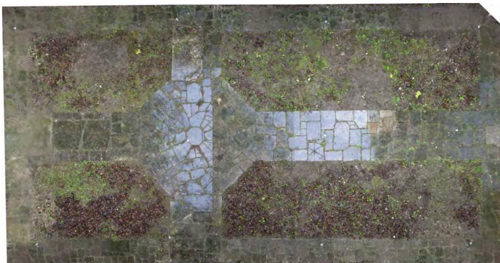
Plate 39. A mosaic of rectified photographs combined to make an accurate record of the post 1954 paving in the interior of the nave.
