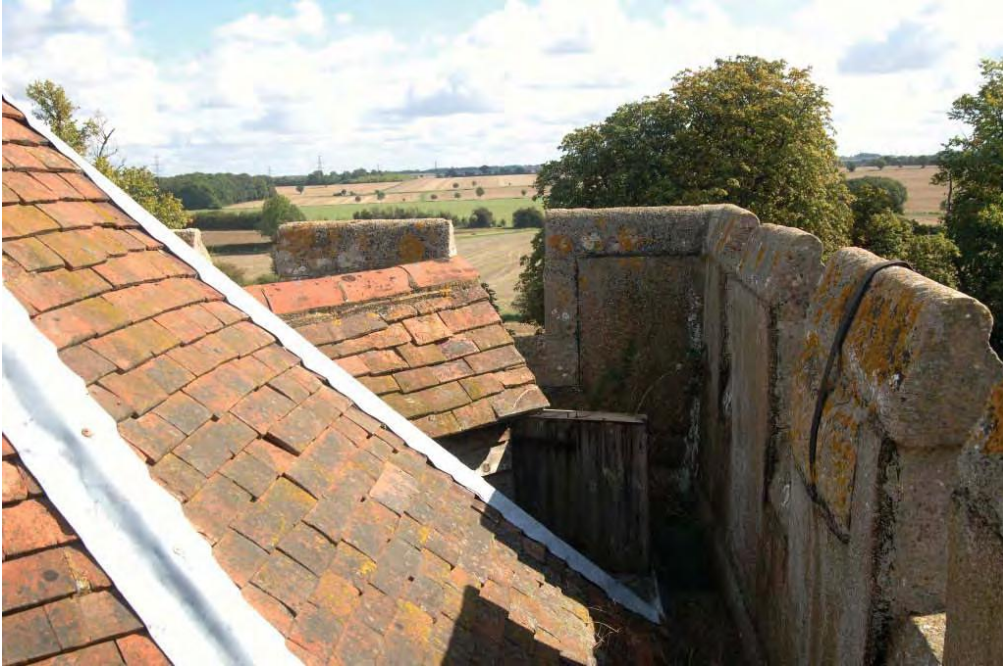
Plate 29. Octagonal roof, parapet crenellations and access from belfry.
