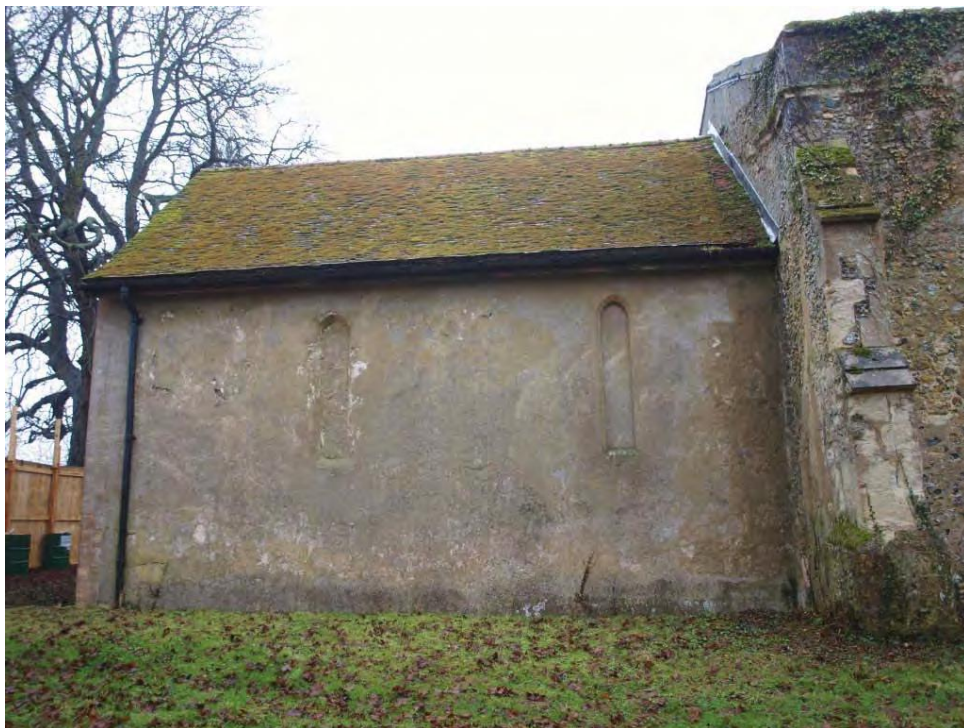
Plate 10. North elevation of the chancel with two blocked original lancet windows.
