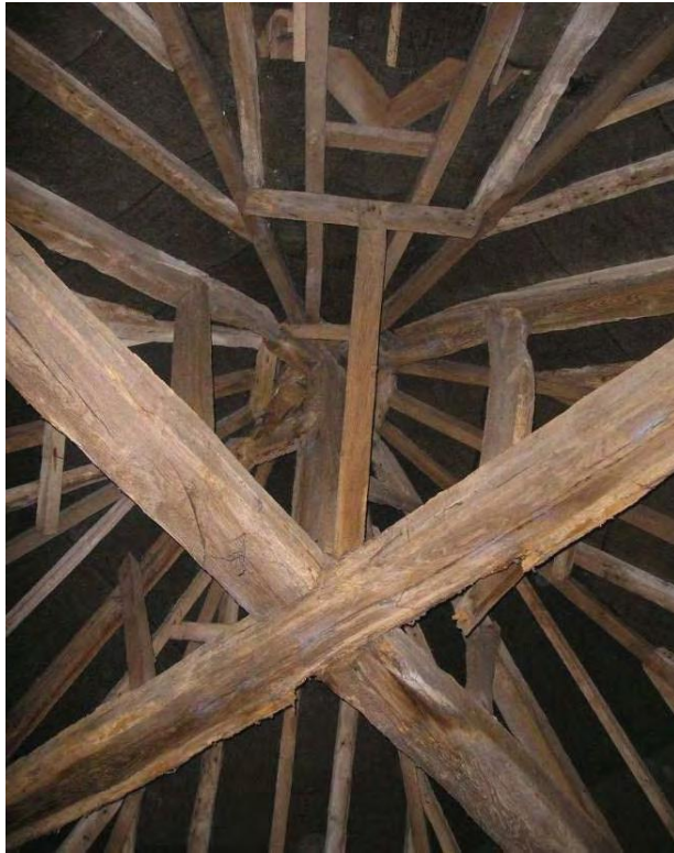
Plate 27. Octagonal timber roof structure.
