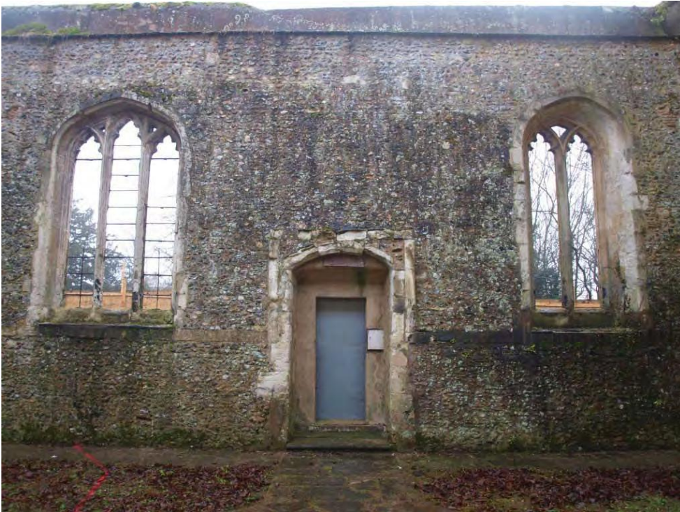
Plate 38. Interior south elevation of the nave.
