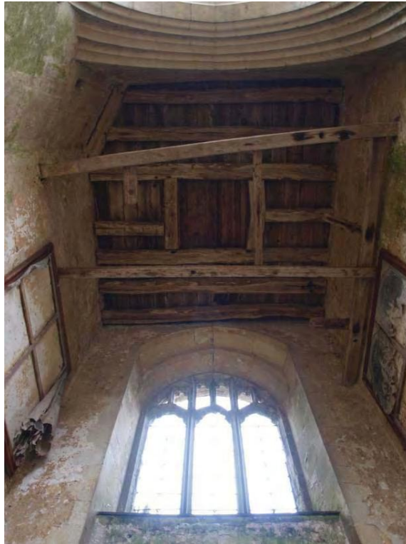
Plate 43. Interior of the tower showing the window in the west wall, bell rope guide wheels against the north wall and the timber joists of the first floor.
