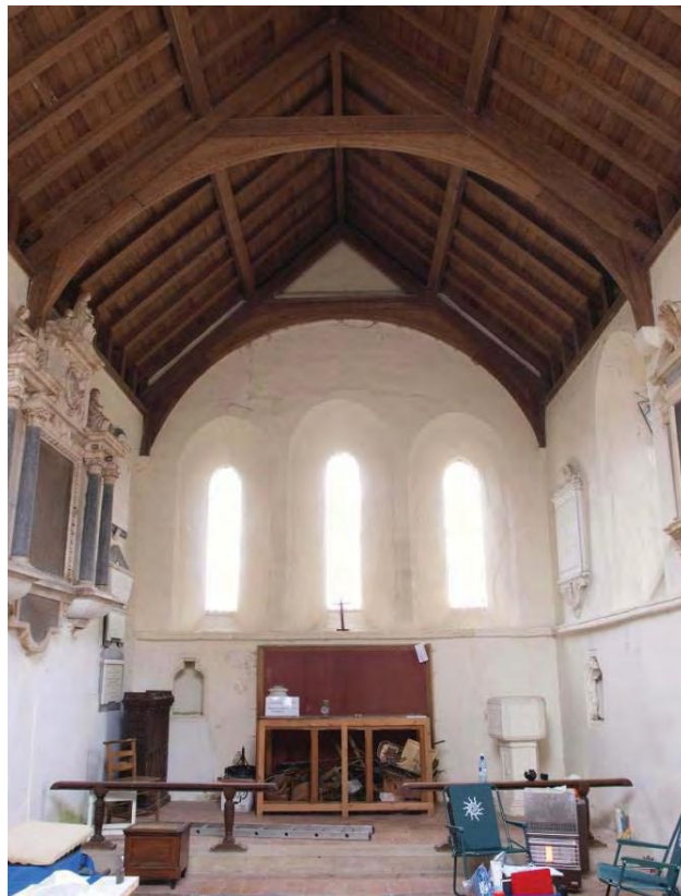
Plate 30. Interior view of the chancel with replacement timber roof.
