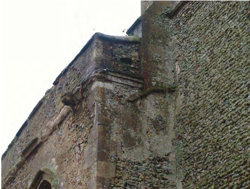
Plate 19. North-west corner of nave showing tower buttress.
