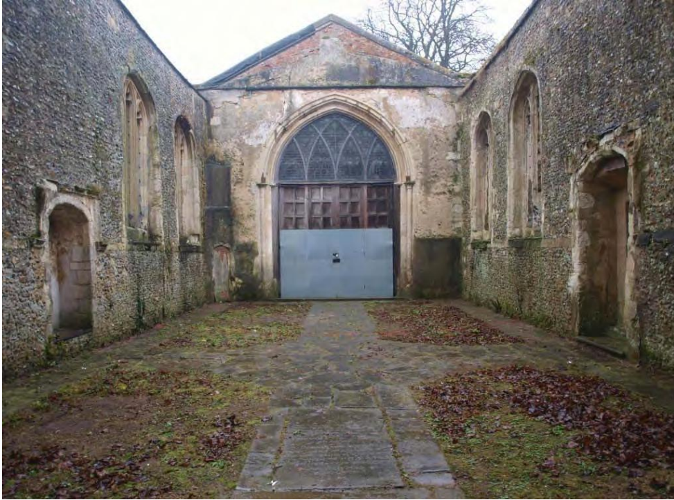
Plate 37. Nave with inserted doors in chancel arch.
