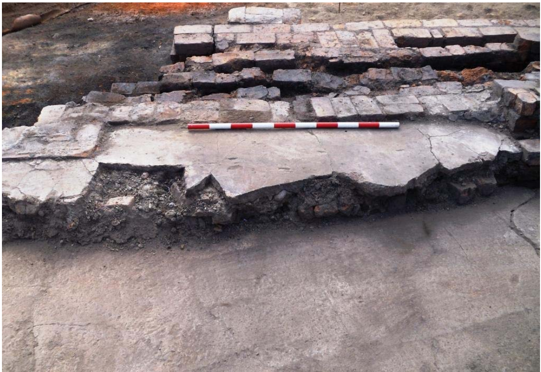
Plate 14. Area A, Phase 4d successive concrete surfaces [1071] and [1075], detail, looking south (1m scale)
