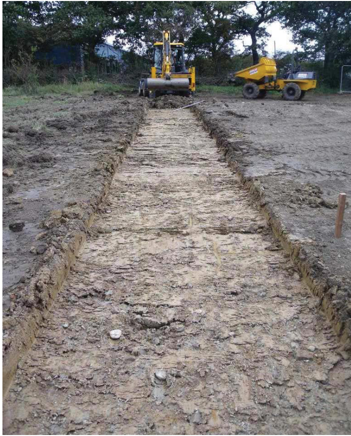
Figure 3. Bulk ground reduction exposing natural clay, looking ENE
