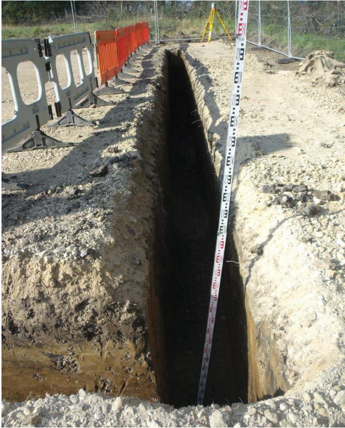
Figure 4. NE wall foundation trench, looking NNW
