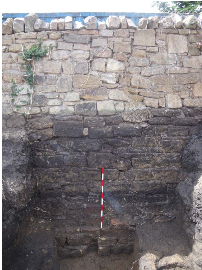
Plate 54: Boundary wall [1006], full height exposed (Section 6), looking south-west ( scale 1m )
