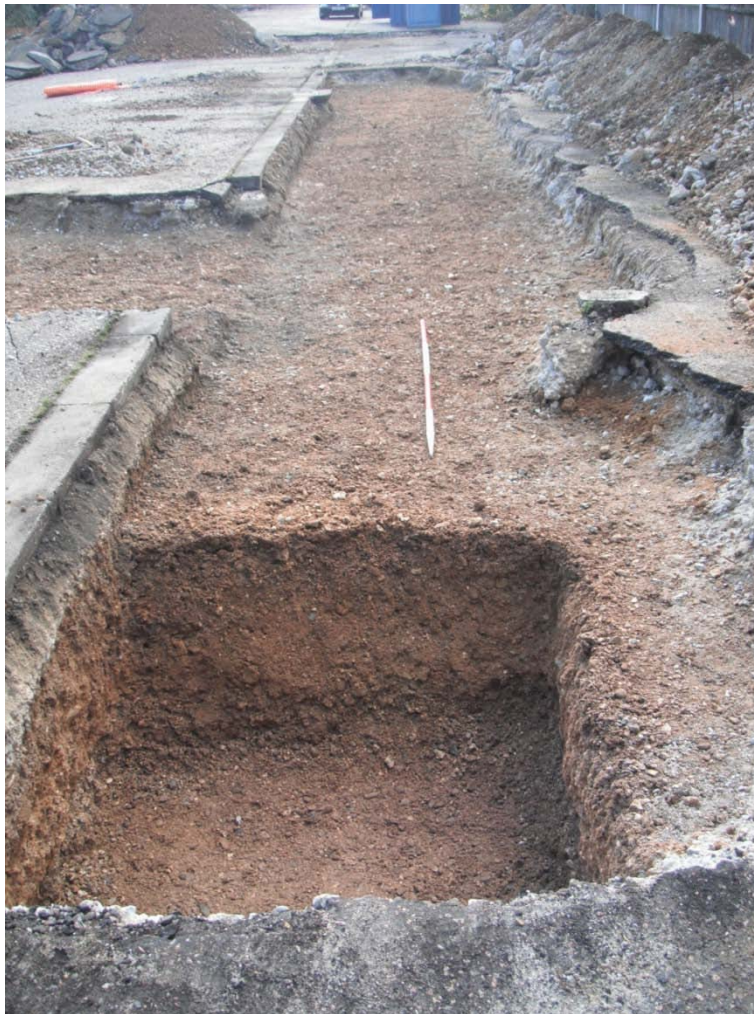
Plate 1: View of Trench 1, looking south with 2m scale
