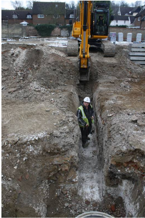
Plate 8: Storm drain looking west
