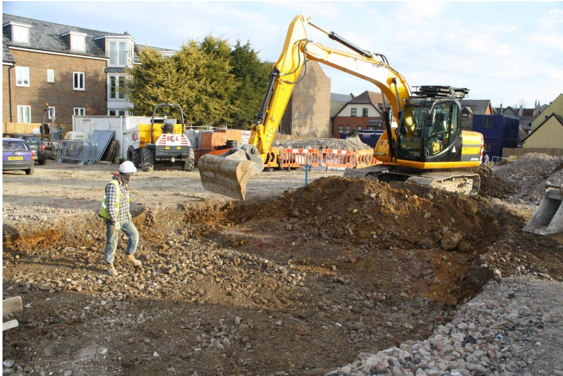
Plate 6: Ground reduction for new road onto the site
