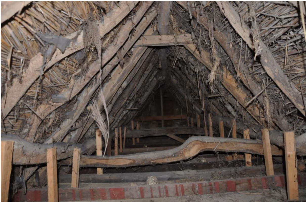
10. Cottage 21 roof showing replaced brace to rear and modern suspended ceiling.
