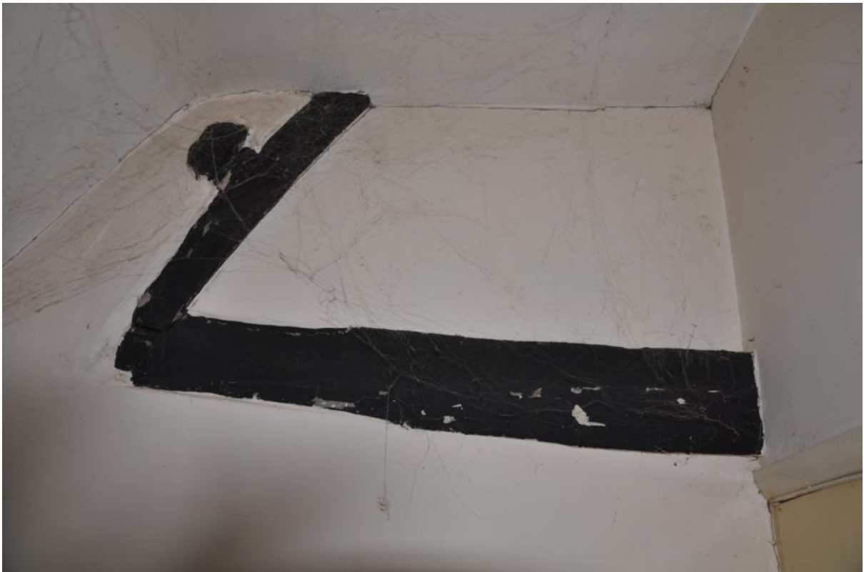
20. Detail of truss in bedroom 1 showing truss with sawn off purlin.
