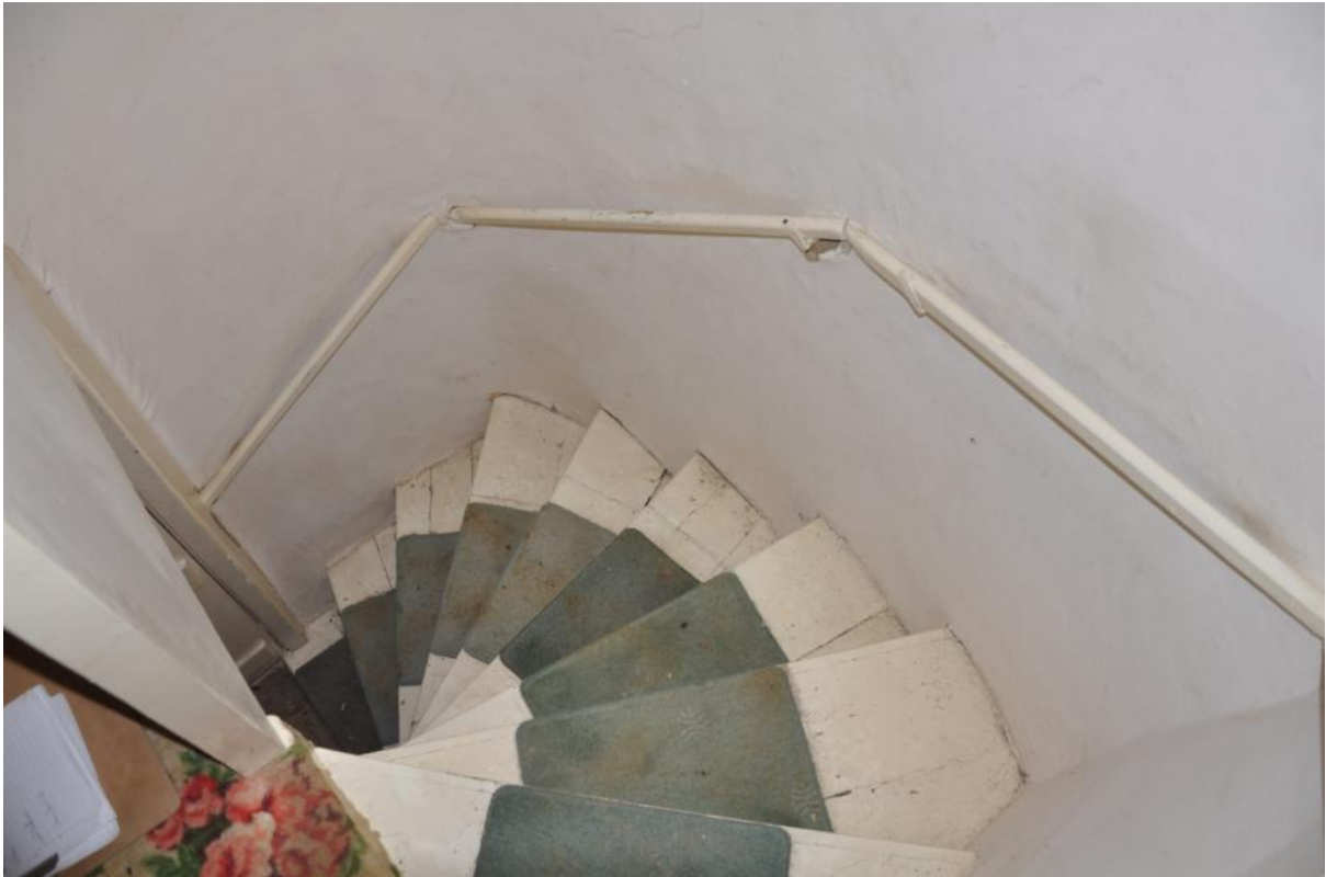
17. Staircase between ground floor and attic.
