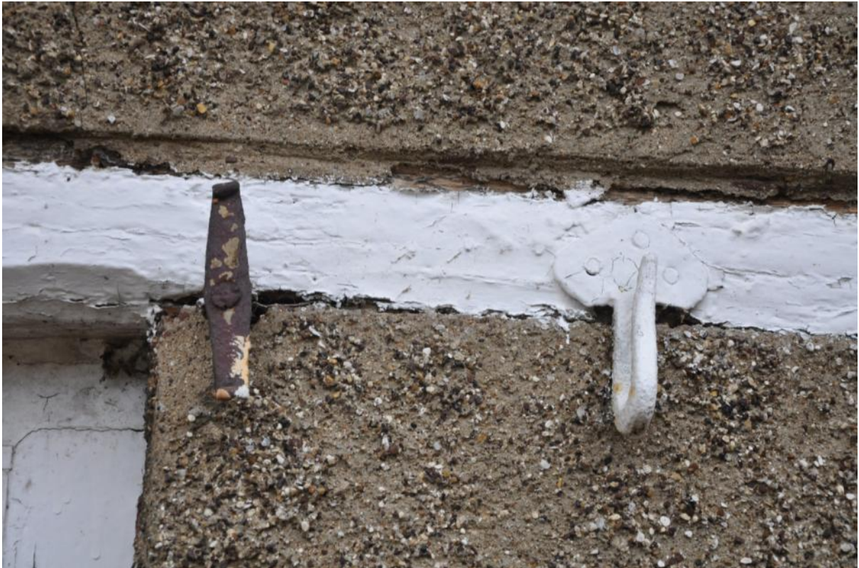
11. Pheasant hook over cottage 23 door lintel.
