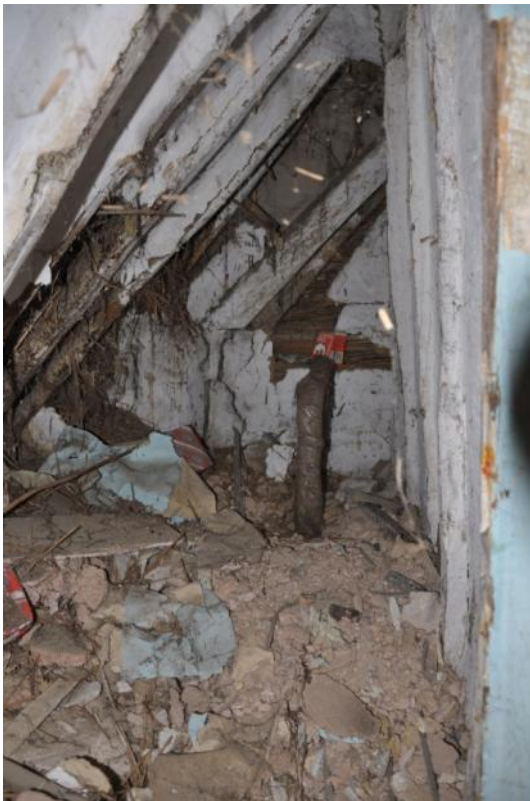
22. Rafters and braces in partitioned roof space in bedroom 2.
