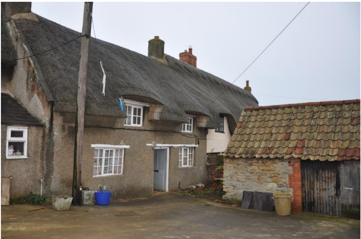
12. Cottage 23 showing dormer windows, lintels and ashlar parapet.
