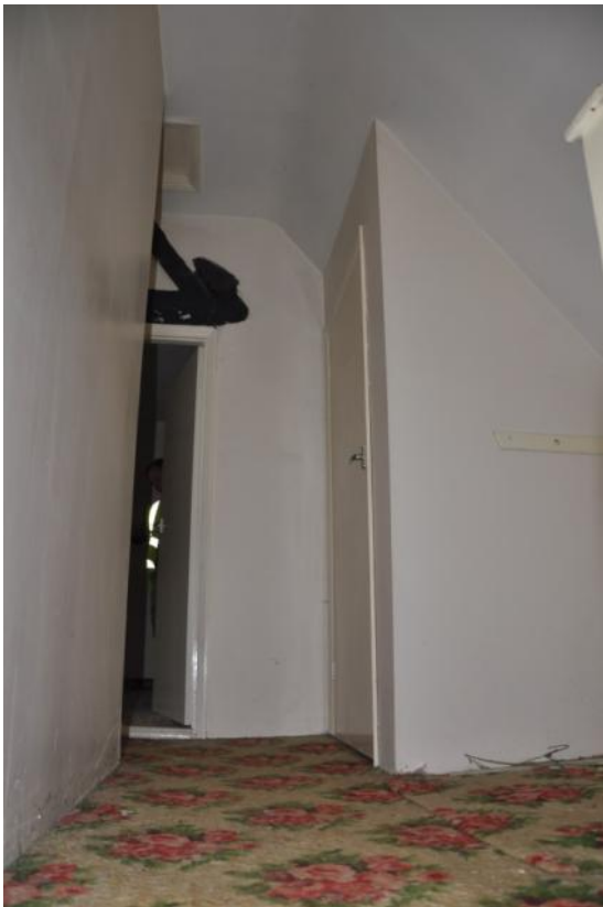
18. Landing showing revealed truss.
