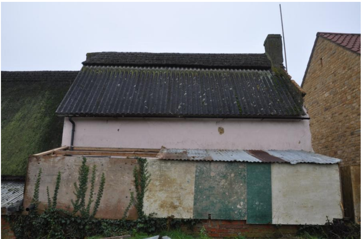
2. Cottage 21 northern rear exterior showing lean to and low brick wall.
