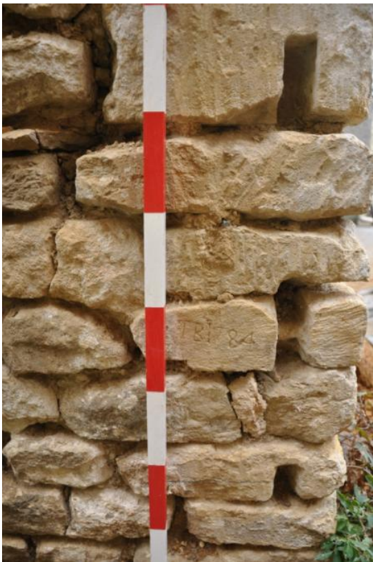
4. Northern quoins on western gable wall showing vertical and diagonal tooling, fence or gate sockets and graffiti dated 1784.
