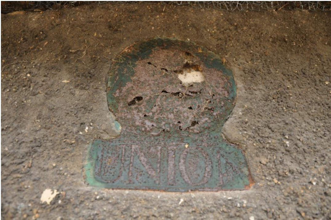
3. Fire insurance plate below eaves on the southern exterior wall.
