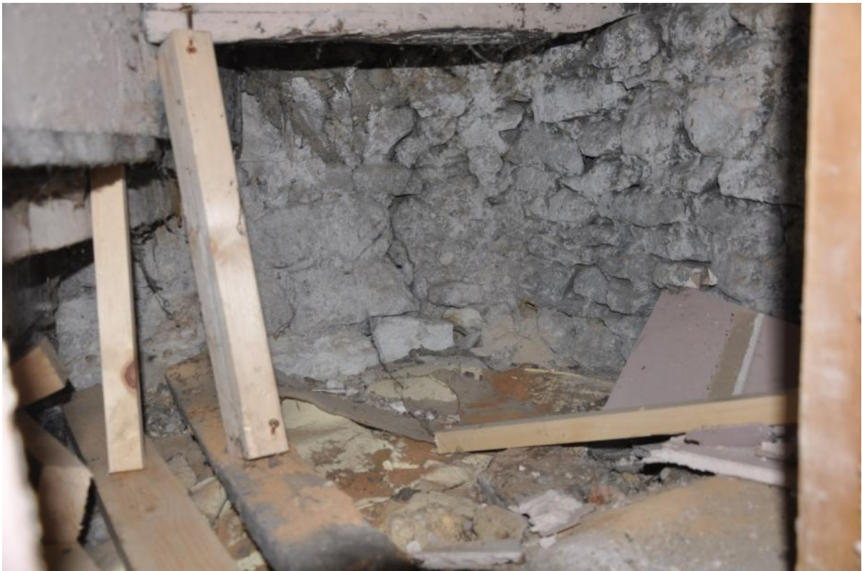
14. Propped stairs and original coursed rubble exterior wall of cottage 23.
