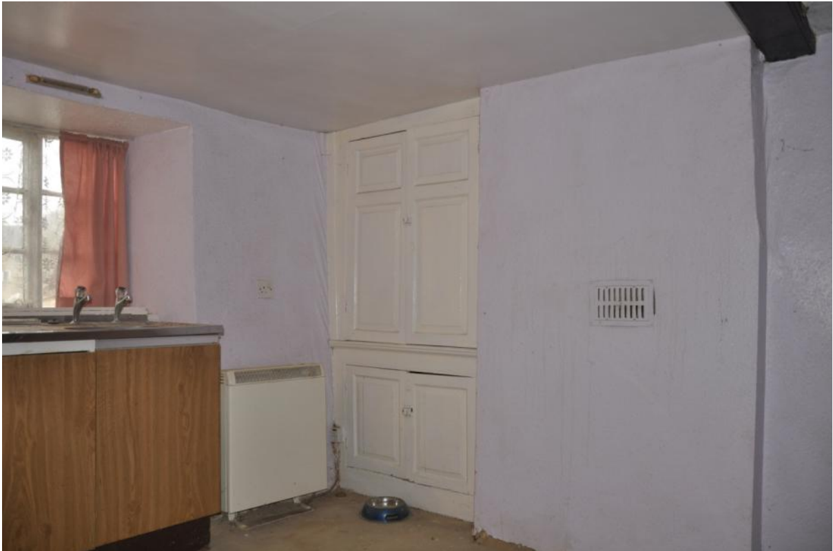
15. Kitchen showing early or original cupboards and blocked chimney breast.
