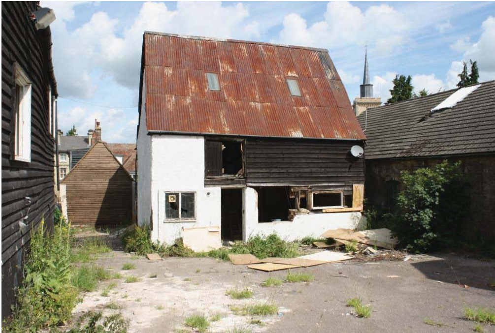
Plate 17. South elevation of the Cottage (Building 4), looking north.
