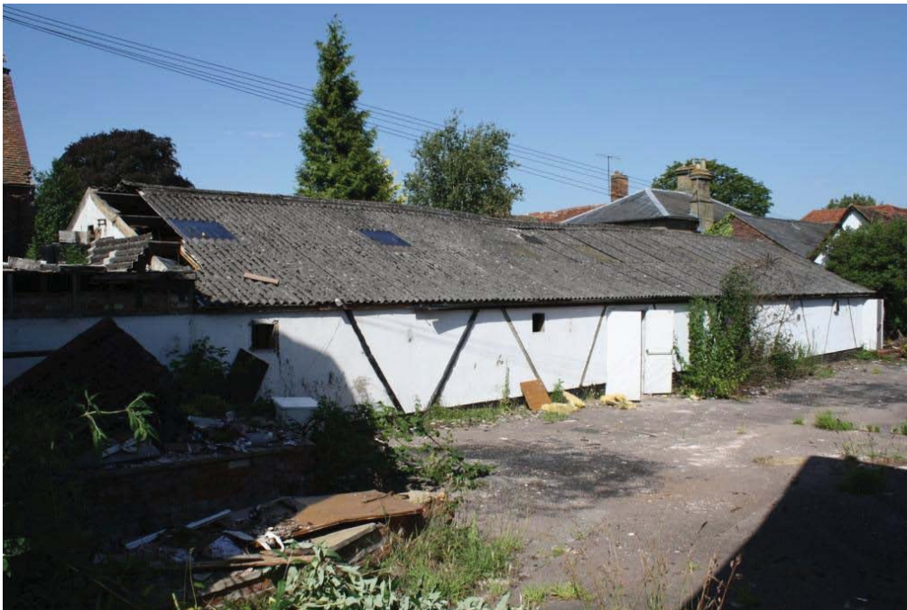
Plate 14. Link Building (Building 3) and yard area, looking north-west.
