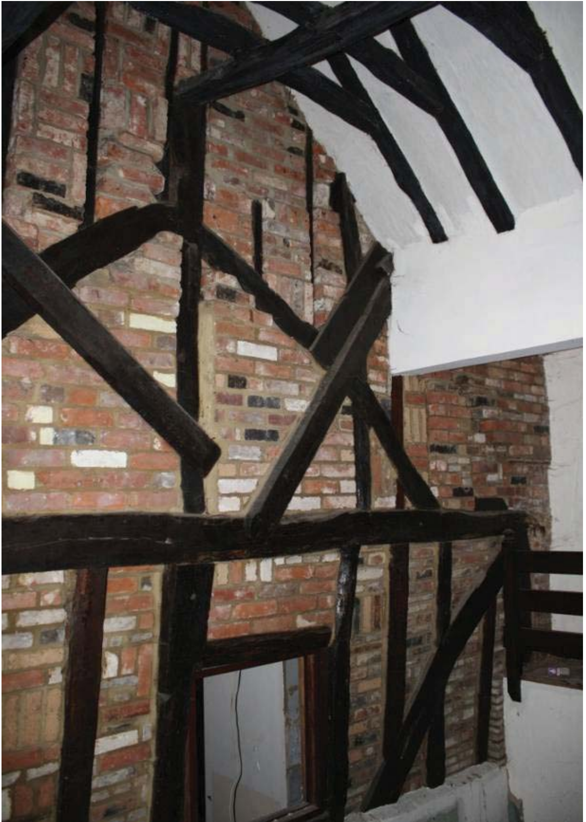
Plate 12. East-west dividing wall in Building 2, looking south-west.
