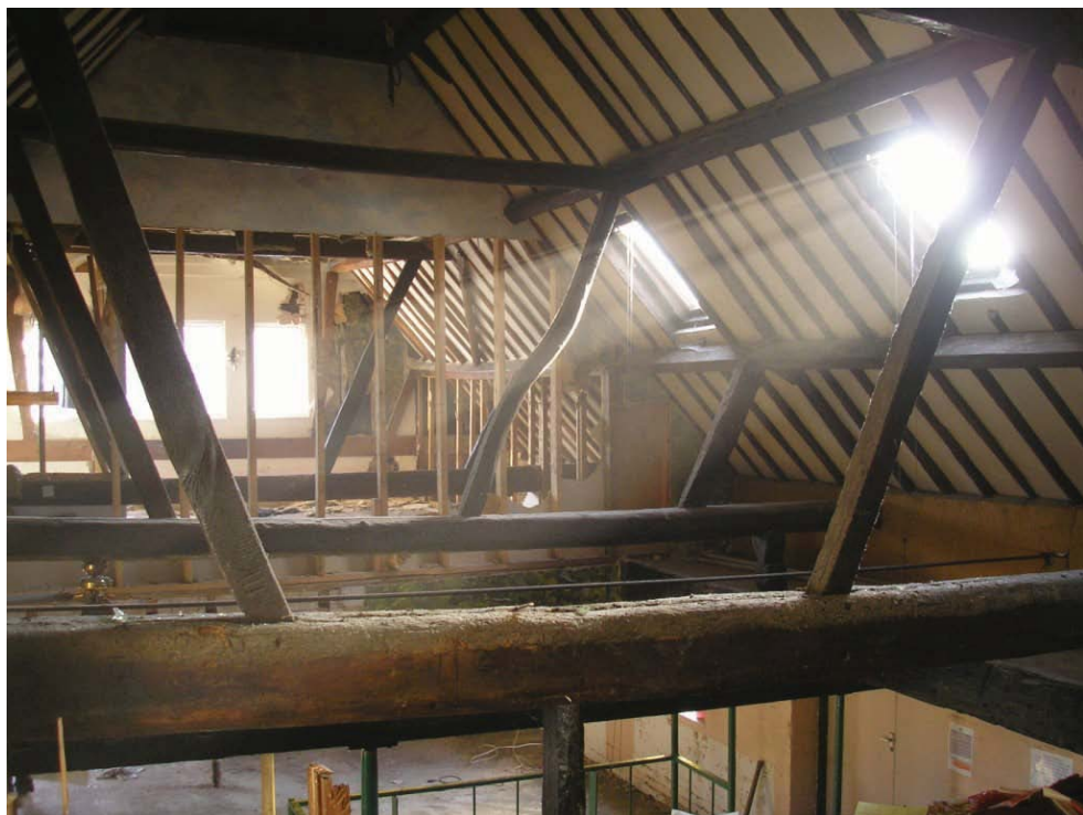
Plate 35. Roof trusses in the east-west block of Maltings Building 5, looking south-east.
