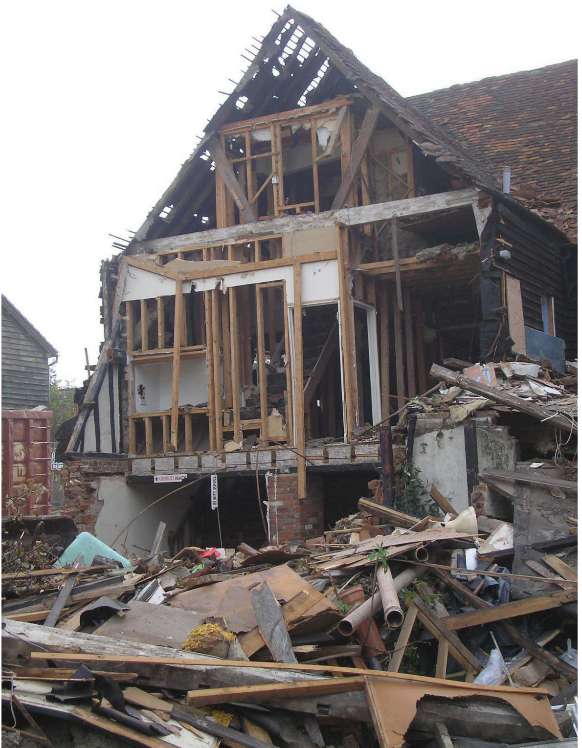
Plate 26a. East wing, Maltings Building 5 during demolition, looking south.
