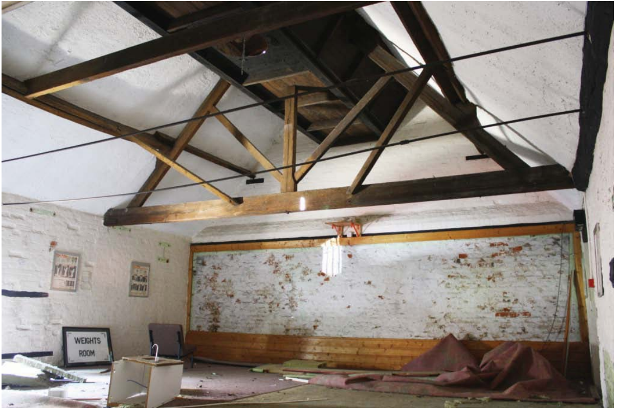
Plate 44. North end of first floor of Building 7, looking north.
