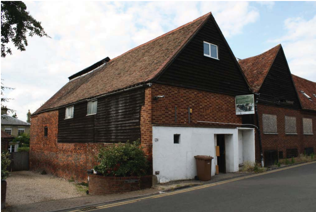
Plate 39. West and south elevations of Building 7, looking north-east.
