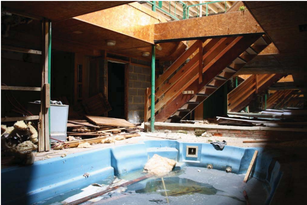
Plate 26. Ground floor, central east-west part of Maltings Building 5, showing spa pool, inserted stairs to the first floor and spa sauna cabins on the left, looking north-east.
