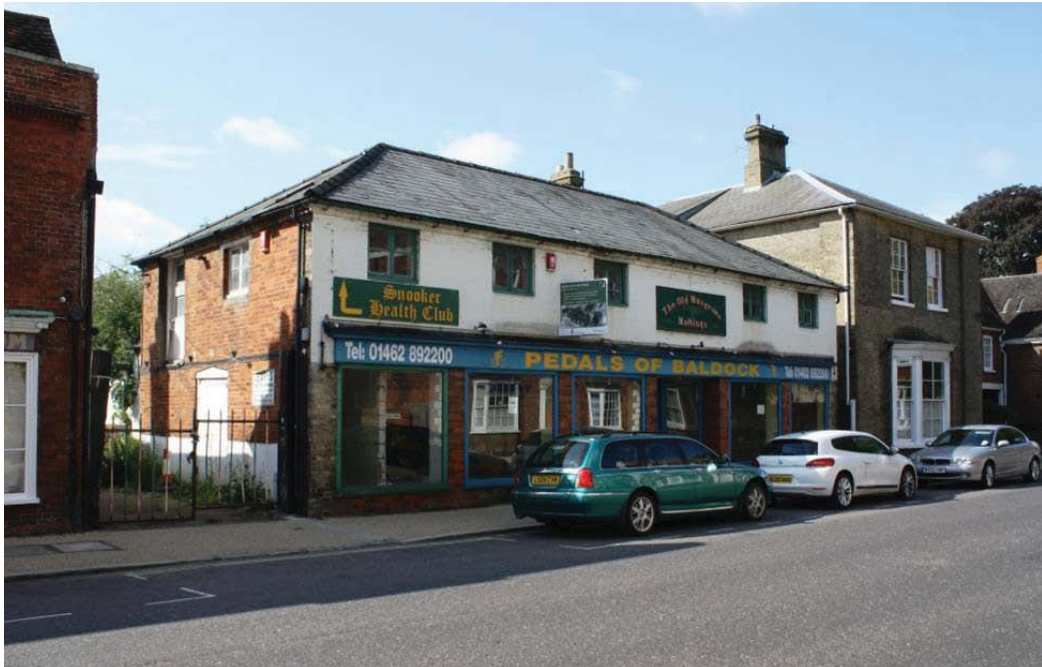
Plate 2. Front (north) elevation of no. 31a Hitchin Street (Building 1).
