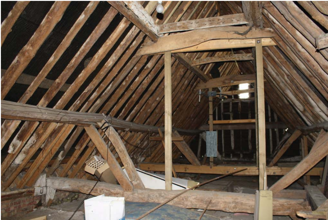
Plate 37. Roof structure of north-south block of Maltings Building 5, looking north.
