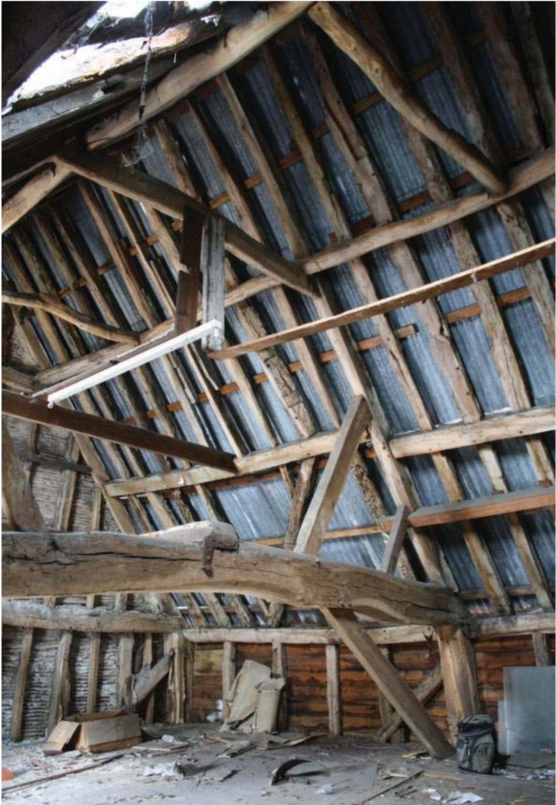
Plate 20. First floor and roof structure of Cottage (Building 4), looking north-west.
