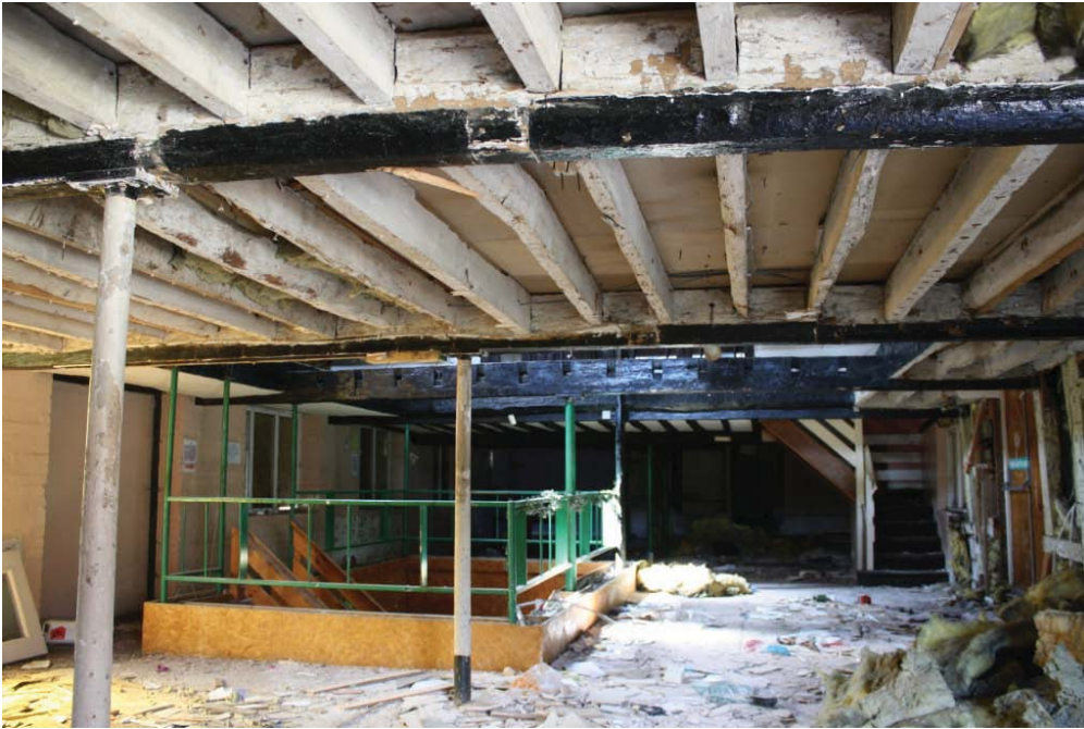
Plate 32. First floor of east-west block of Maltings Building 5, looking west.
