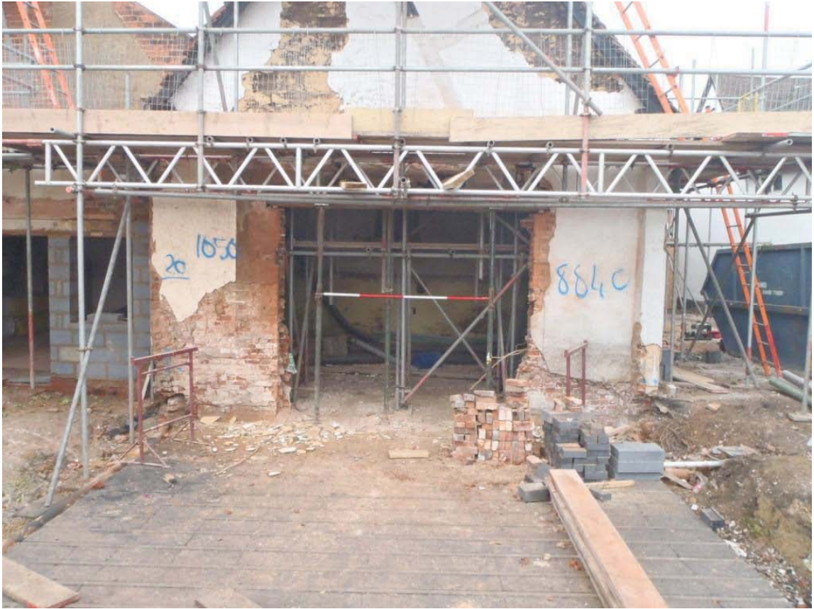
Plate 51. View of south elevation of Building 2 with new opening.
