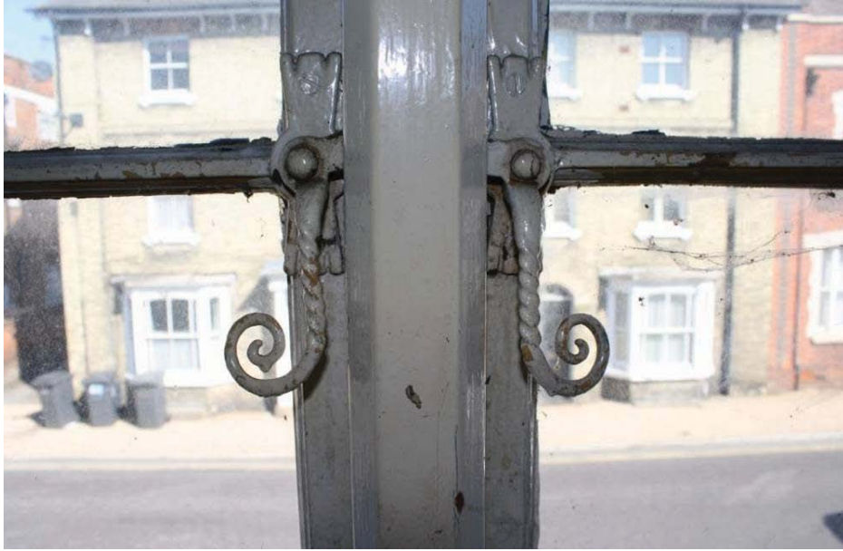
Plate 9. Detail of original decorative catch on timber-framed casement window, first floor of Building 1, overlooking Hitchin Street.
