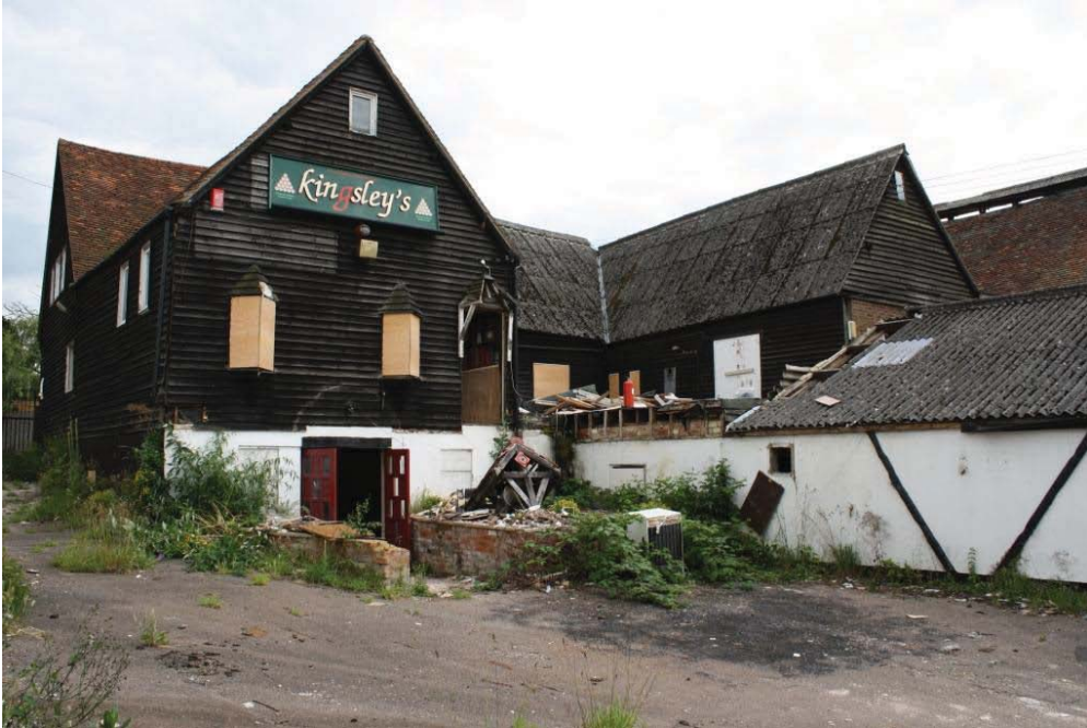
Plate 21. North elevations of Maltings Building 5, with Link Building 3 on the right and flat roofed Building 6 between the two wings of Building 5.
