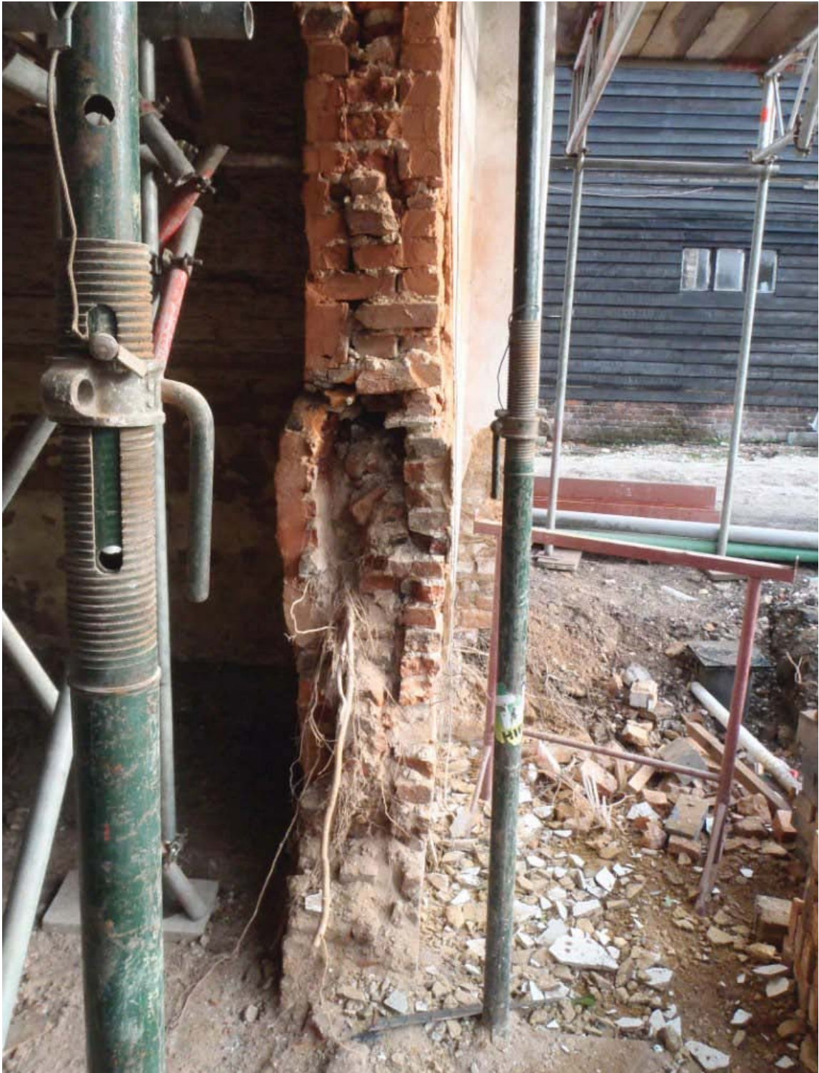
Plate 52. South gable end of Building 2 seen in cross section looking north-east, with a noticeable change in brickwork.
