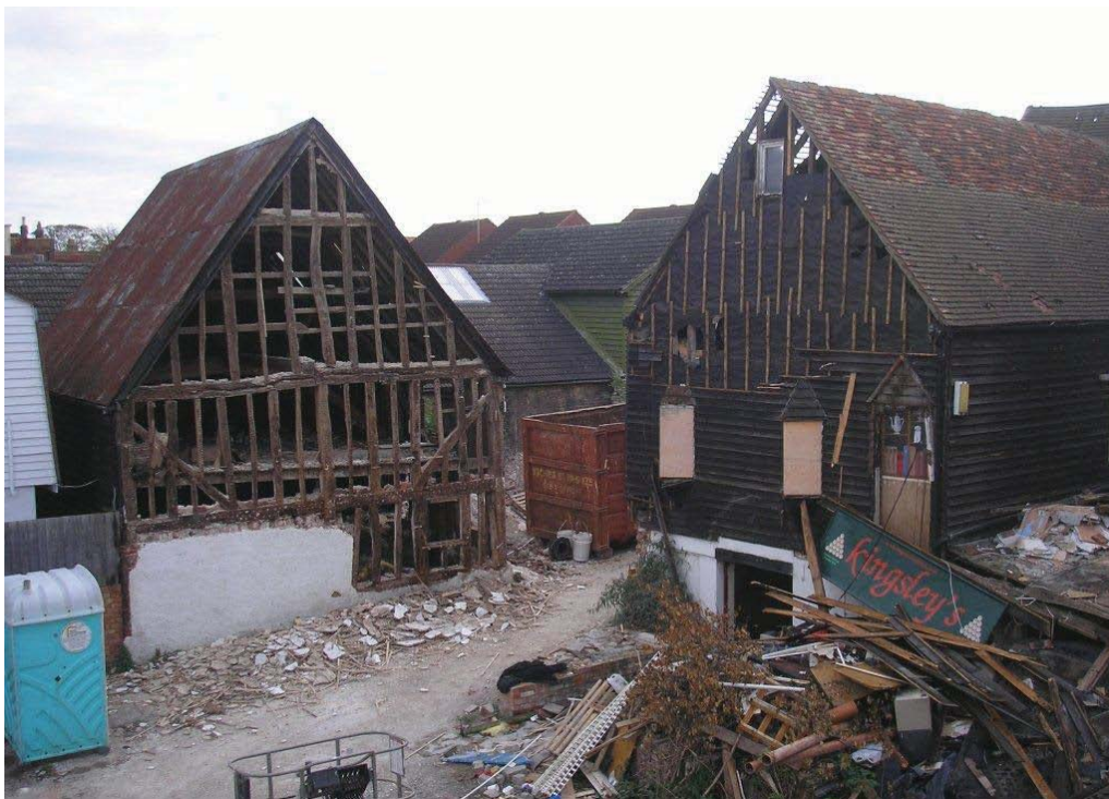
Plate 18. Exposed timber-frame of west elevation of the Cottage (Building 4), looking south-east.
