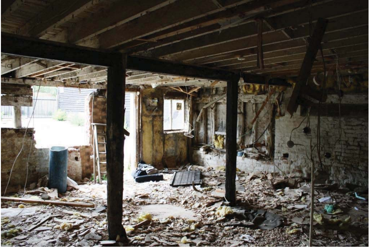
Plate 19. Ground floor of Cottage (Building 4), looking south-west.
