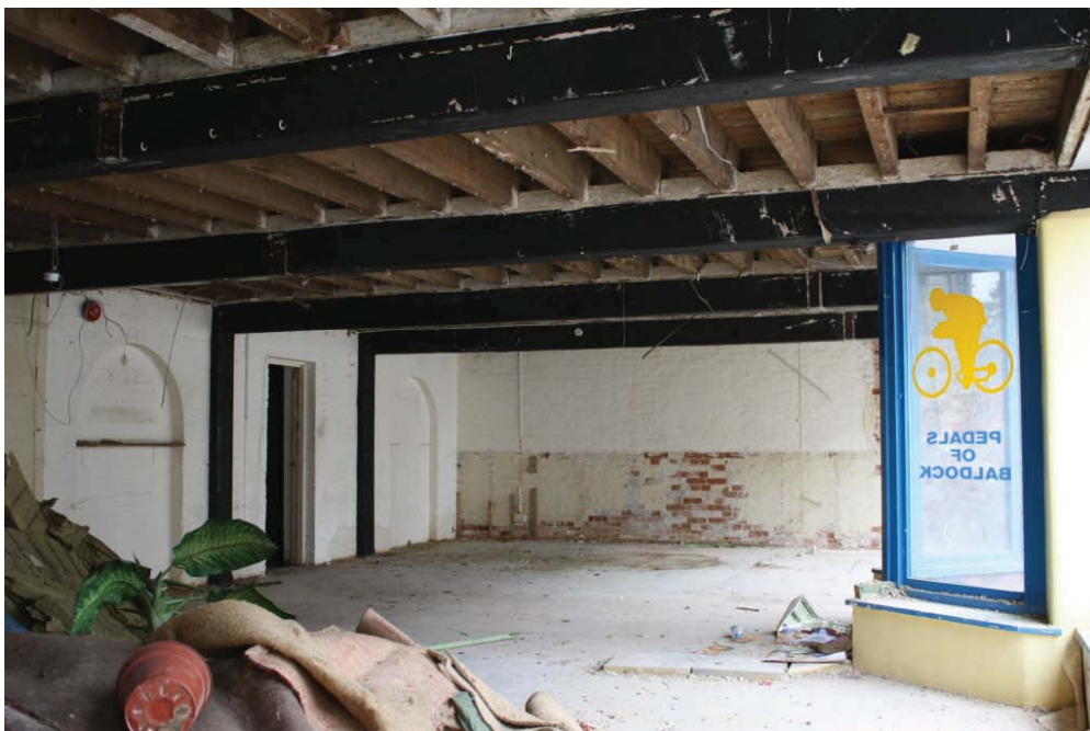
Plate 4. Ground floor shop of 31a Hitchin Street (Building 1) looking south-west.
