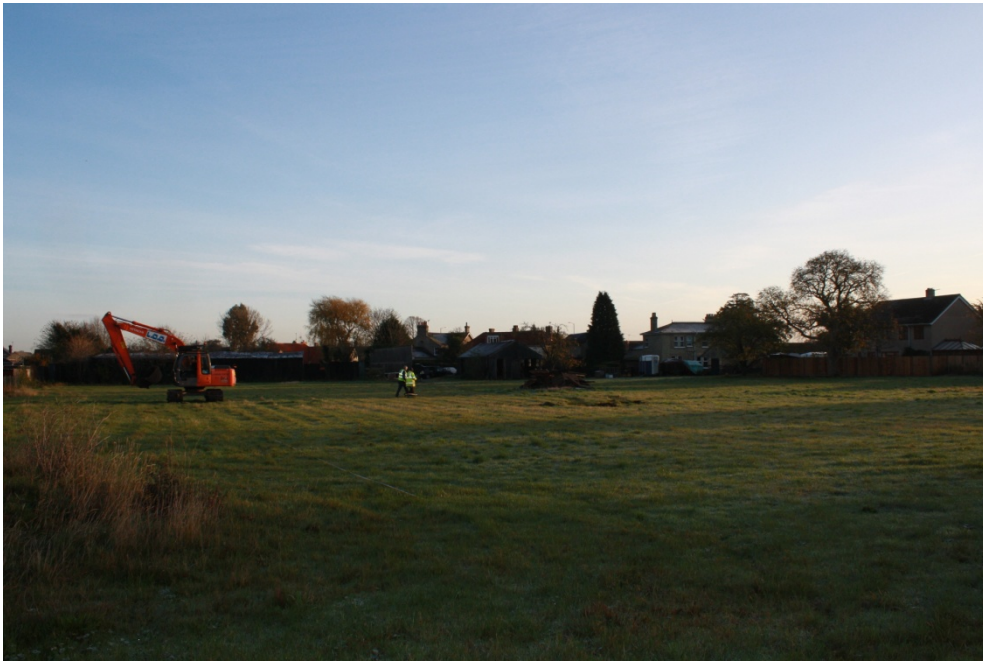
Plate 1. Site prior to machine stripping. Facing northwest
