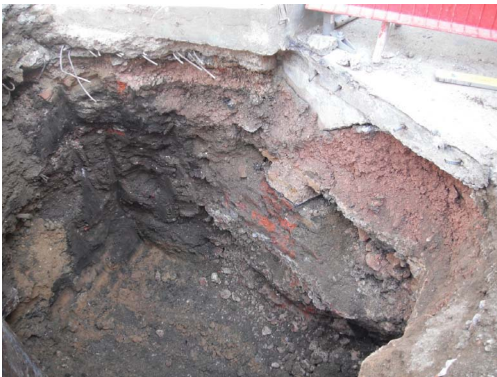
Plate 2: Truncated natural sands exposed beneath basement slab; view NNW at NW corner of site.
