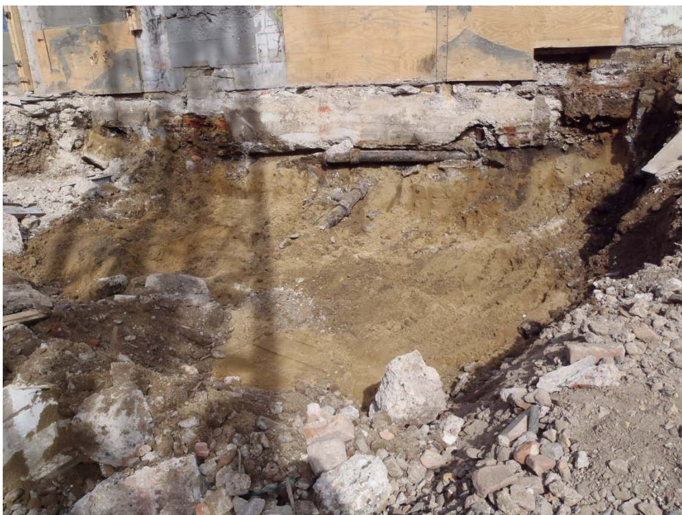
Plate 2: Truncated natural sands exposed beneath basement slab; view NNW at NW corner of site.
