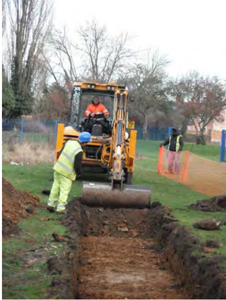
Trench 6 being excavated
