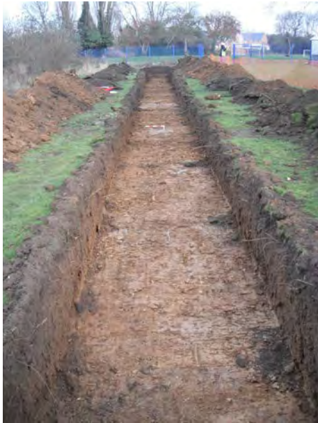
Trench 6 view east
