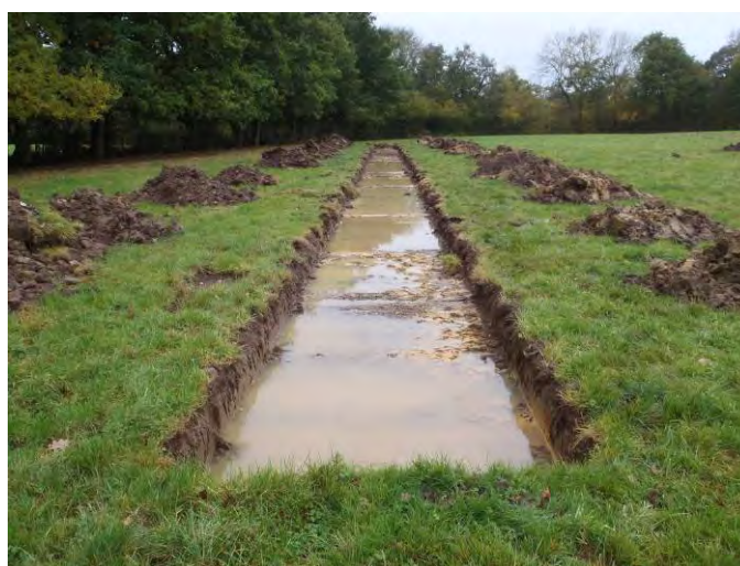
Plate 7: Trench 31. View looking west to show flooding
