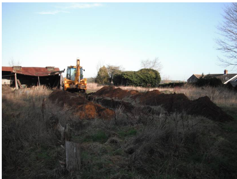
Trench 2 being excavated – view north
