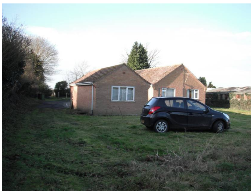
Current buildings occupying the site looking west
