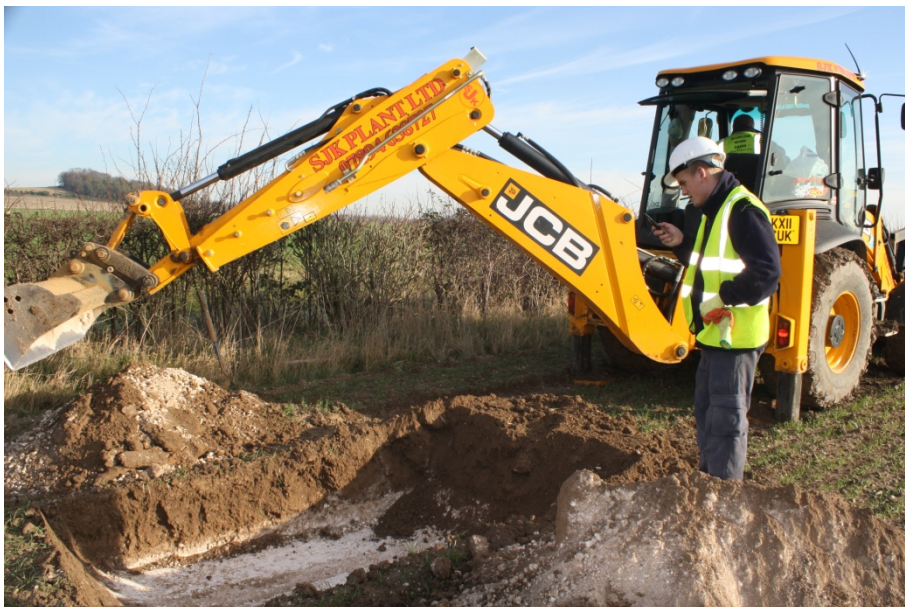
Excavation of Test Pit
