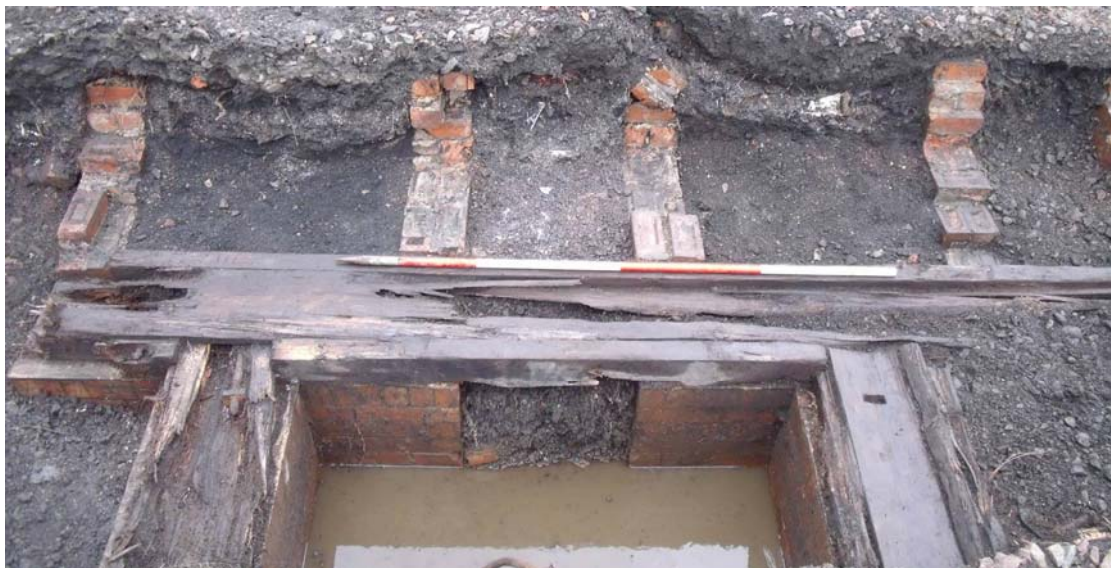
Figure 15 Trench 3, Structure [400], timber [371] detail, looking north-west ( scale 2m )
