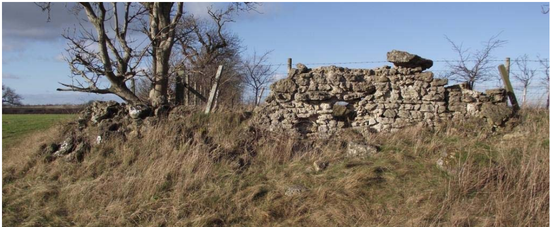
Plate 12. Phases 2 & 3 area, detail of northern field boundary wall, looking north
