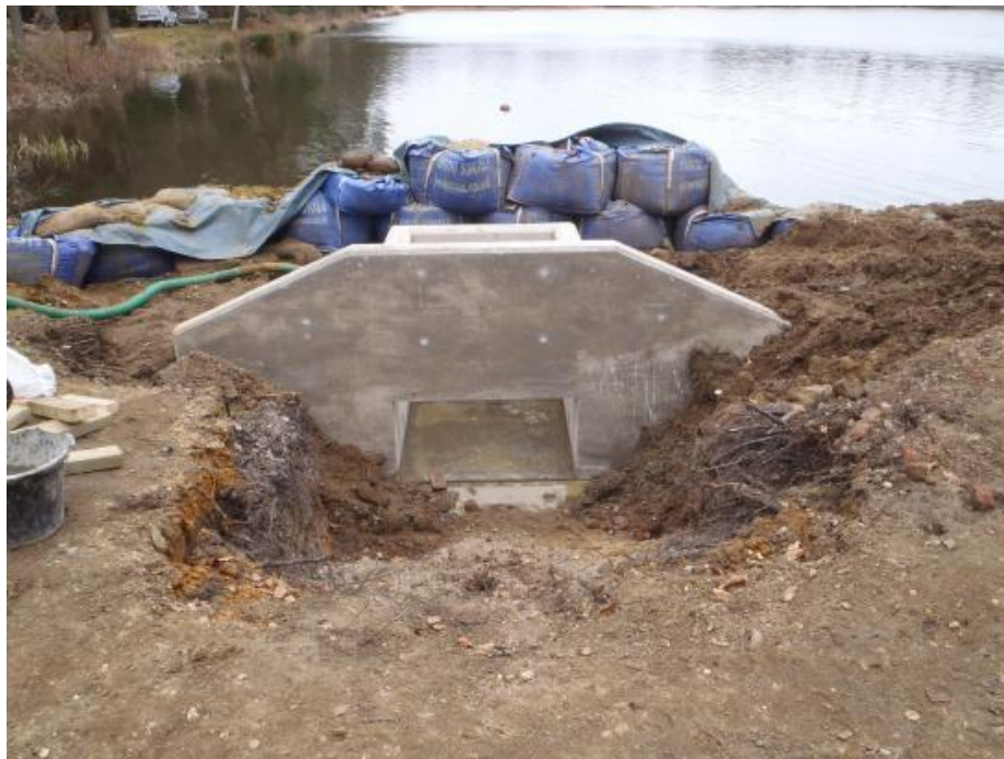
Plate 5: View looking east of cofferdam and newly constructed culvert head.
