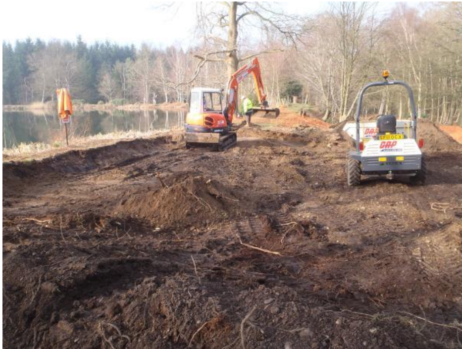
Plate 1: View looking north during excavation of auxiliary spillway
