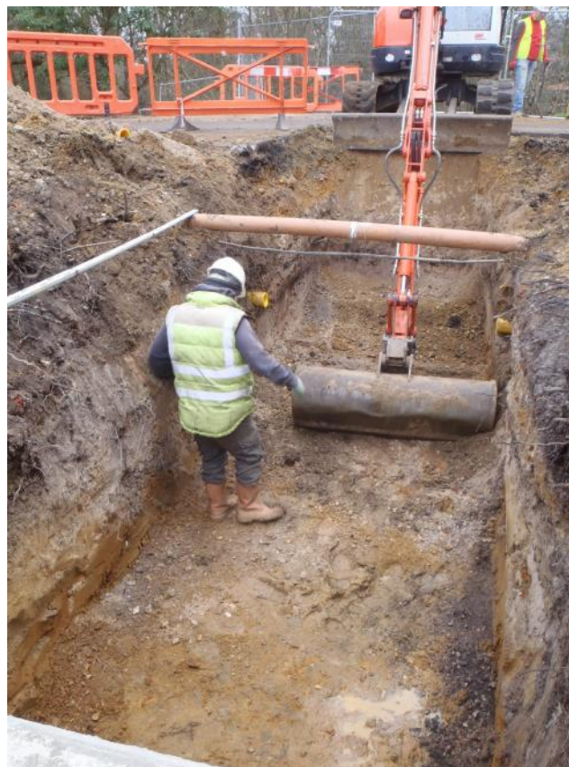
Plate 6: View looking east of main spillway area on eastern side of rear access road
