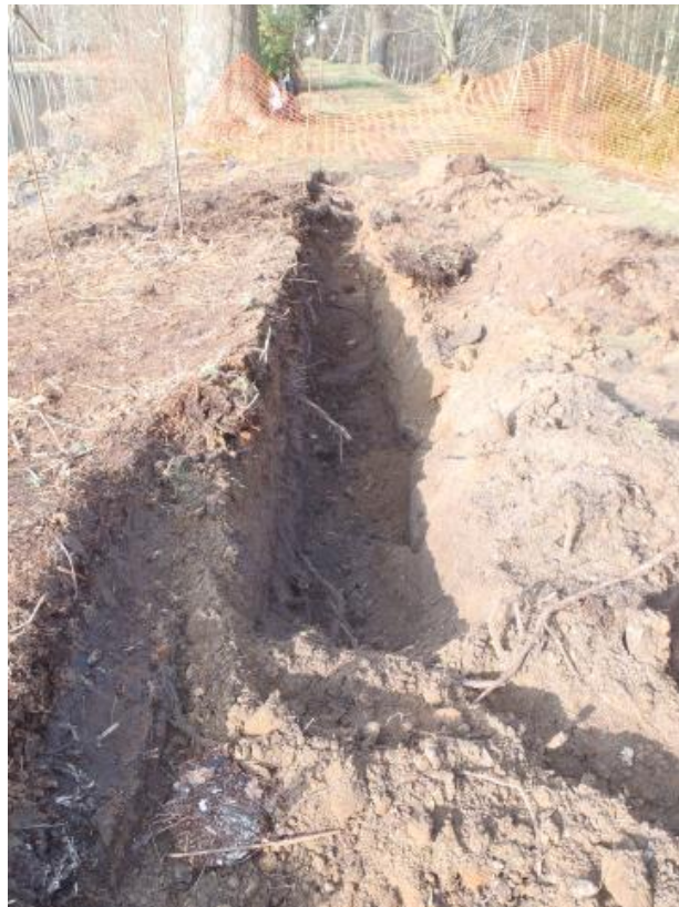
Plate 2: View looking north of slot for concrete beam
