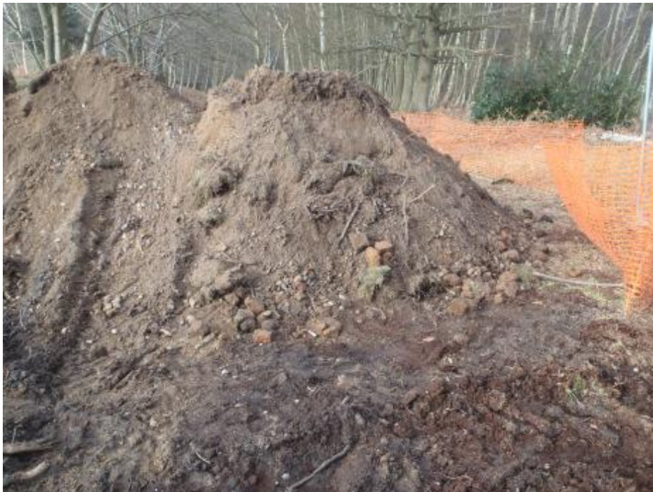
Plate 4: Excavated material from auxiliary spillway containing brick and tile rubble
