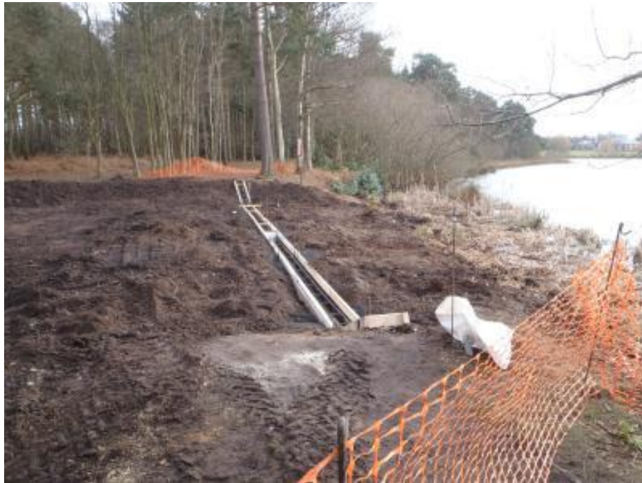
Plate 3: View looking south of completed slot for concrete beam
