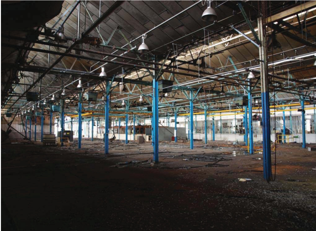
Plate 81. Interior of Building 32 looking northeast.
