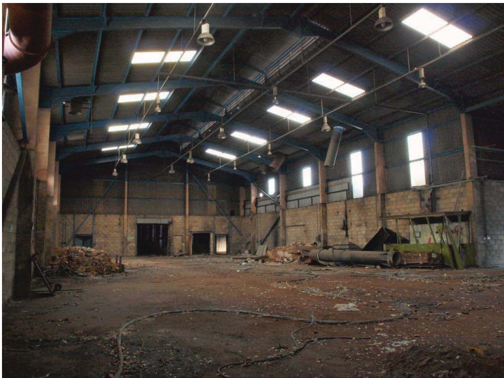
Plate 42. Interior of the Shotblast Building (12) looking northeast.
