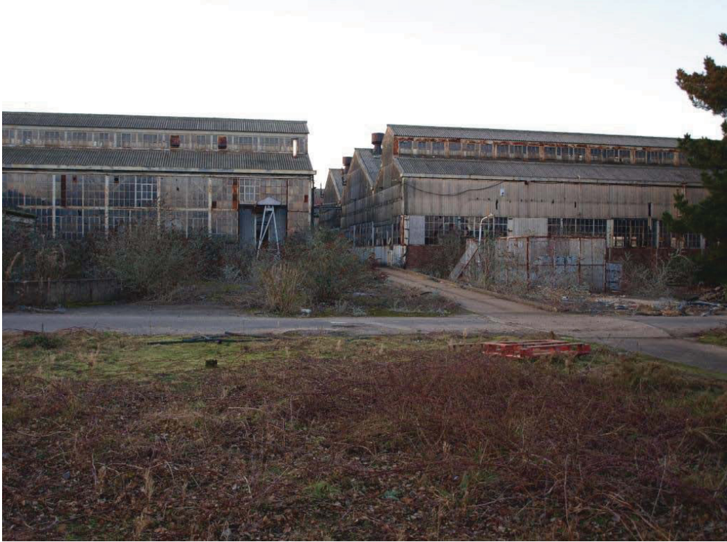
Plate 51. East elevations of Building 17 (right) and Building 24 (left), looking west.
