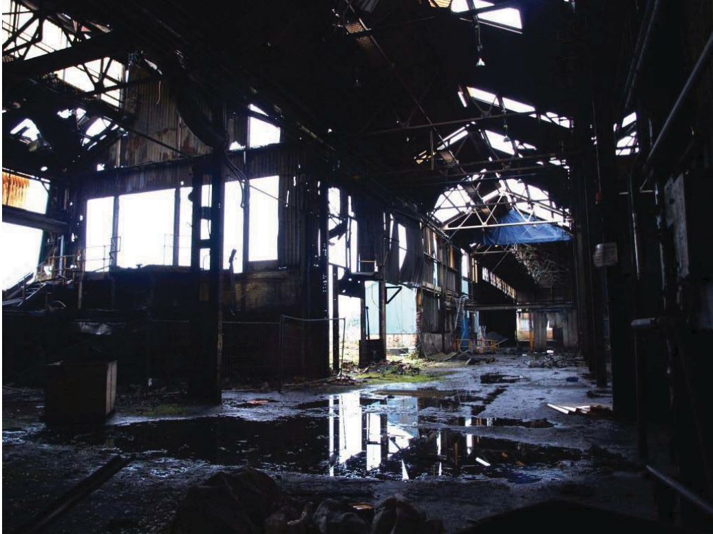
Plate 85. Interior of Old Grey Iron Foundry Building 35 looking north.
