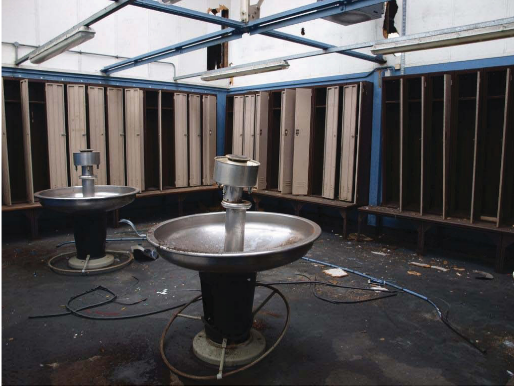
Plate 35. Mezzanine changing room in northwest corner of Building 7.
