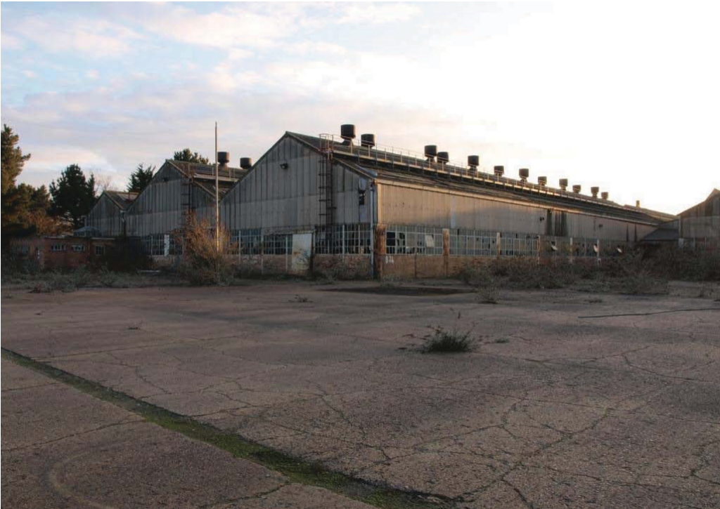
Plate 50. North and west elevations of Building 17, looking southeast.
