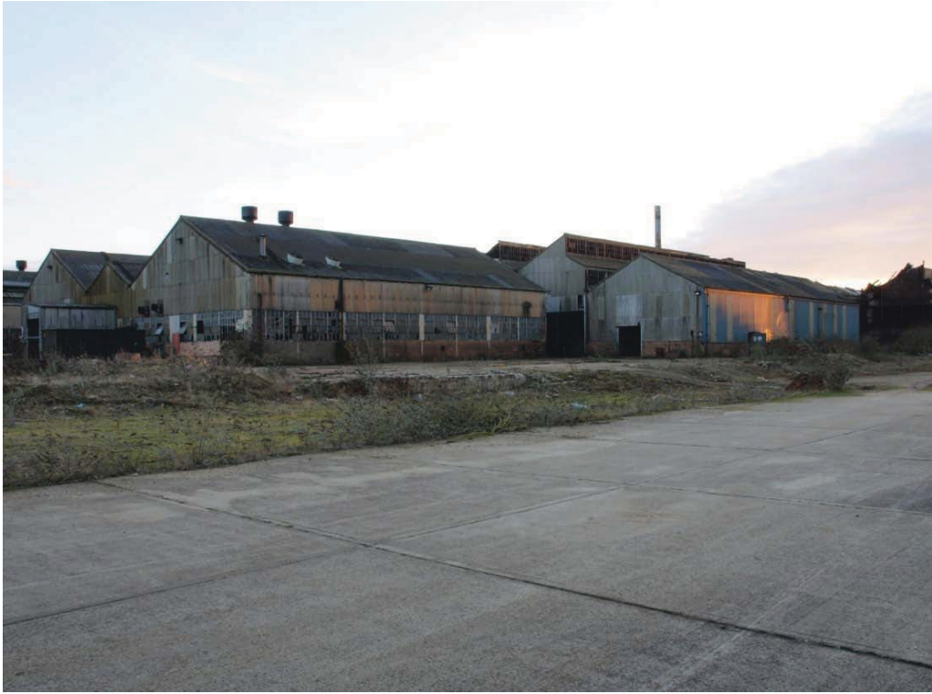
Plate 47. West and north elevations of Buildings 15 (right) and 16 (left), looking southeast.
