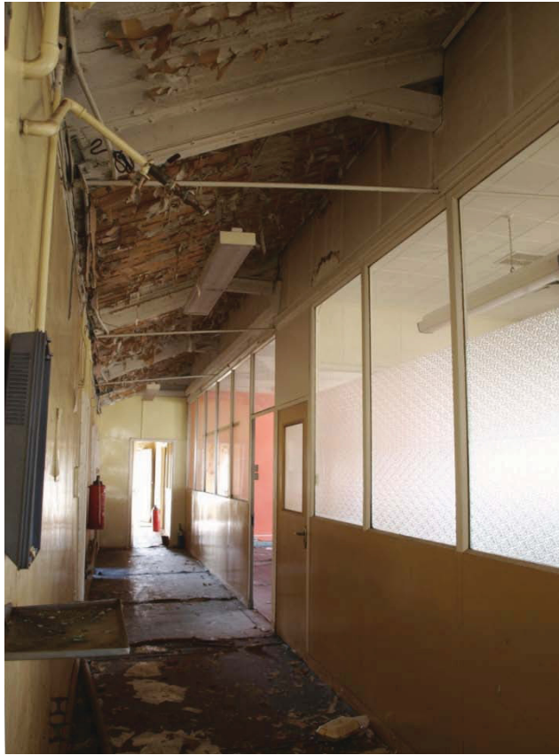
Plate 39. Interior corridor of Works Pavilion (10) looking east.
