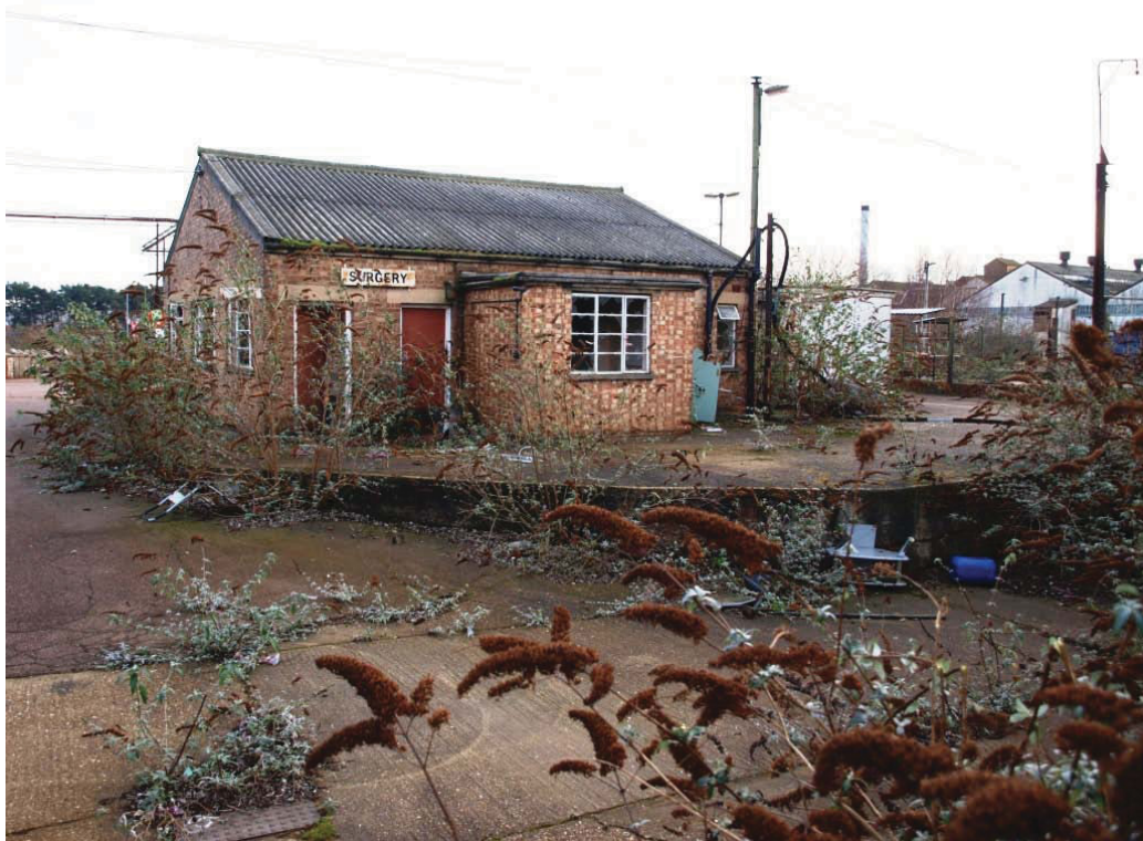
Plate 66. West elevation of the Surgery Building (23).
