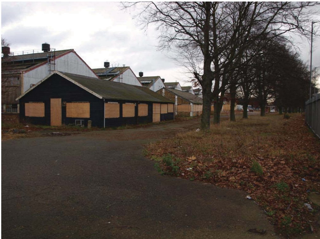
Plate 14. South elevation and west gable of Black Hut (4) with south gables of Union Machine and Assembly Building (7) beyond and on the right trees and boundary fence along Nacton Road.
