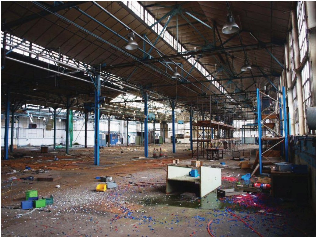
Plate 68. Interior of Building 24 looking north.
