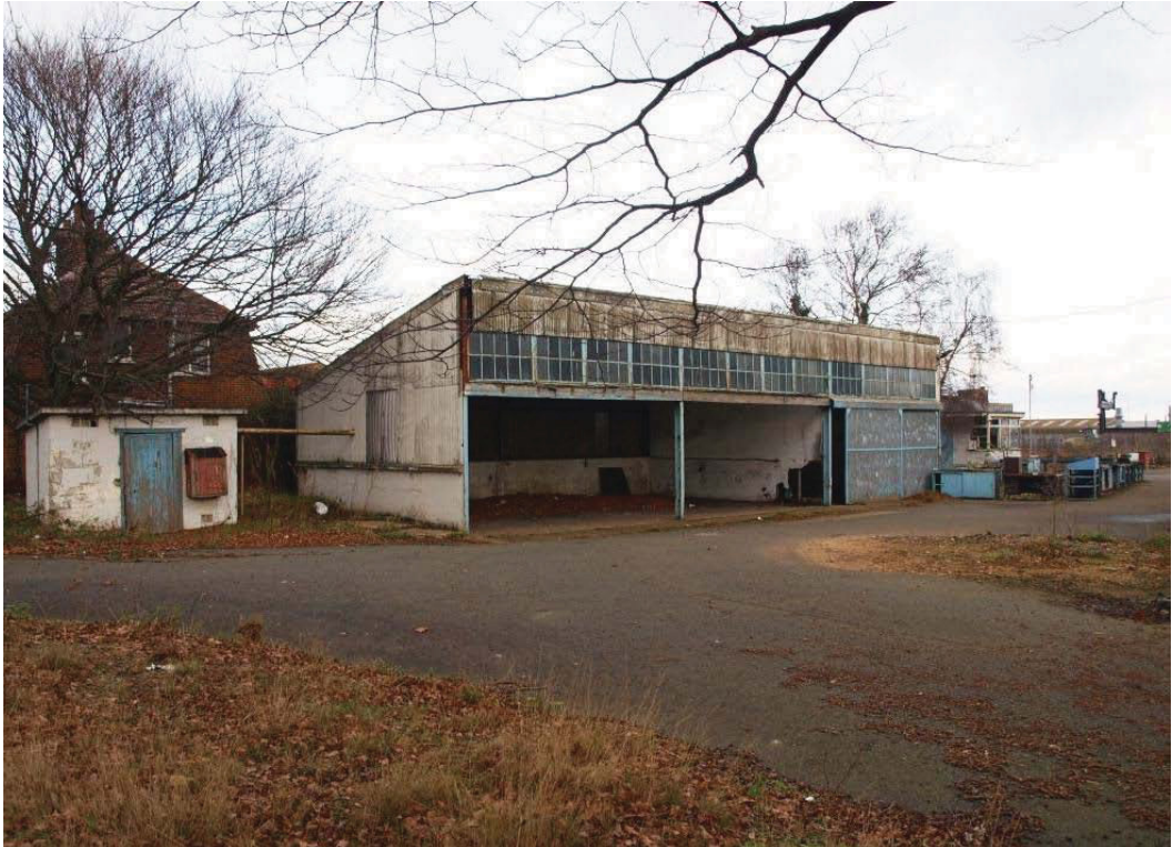
Plate 37. Garage (8) in the southwest corner of the site with the Weighbridge (9) seen on the right.
