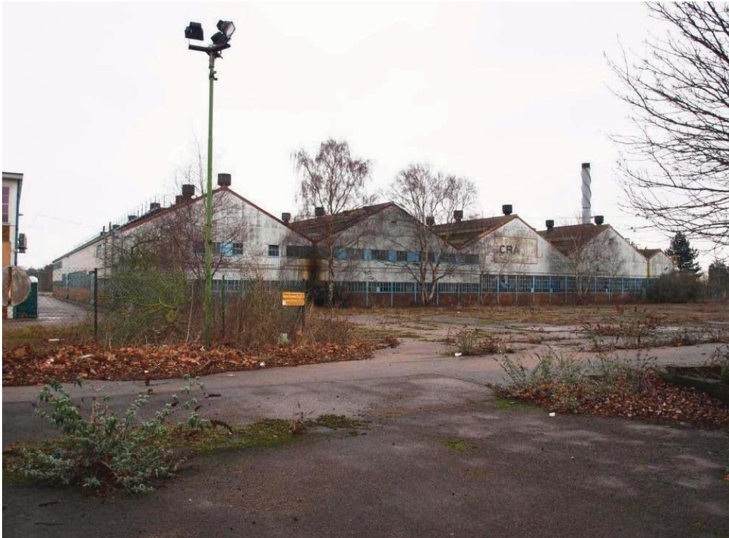
Plate 15. South and west elevations of Old Bronze Foundry (5).
