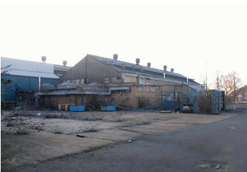
Plate 30. West and north elevations of Union Machine and Assembly Building (7).
