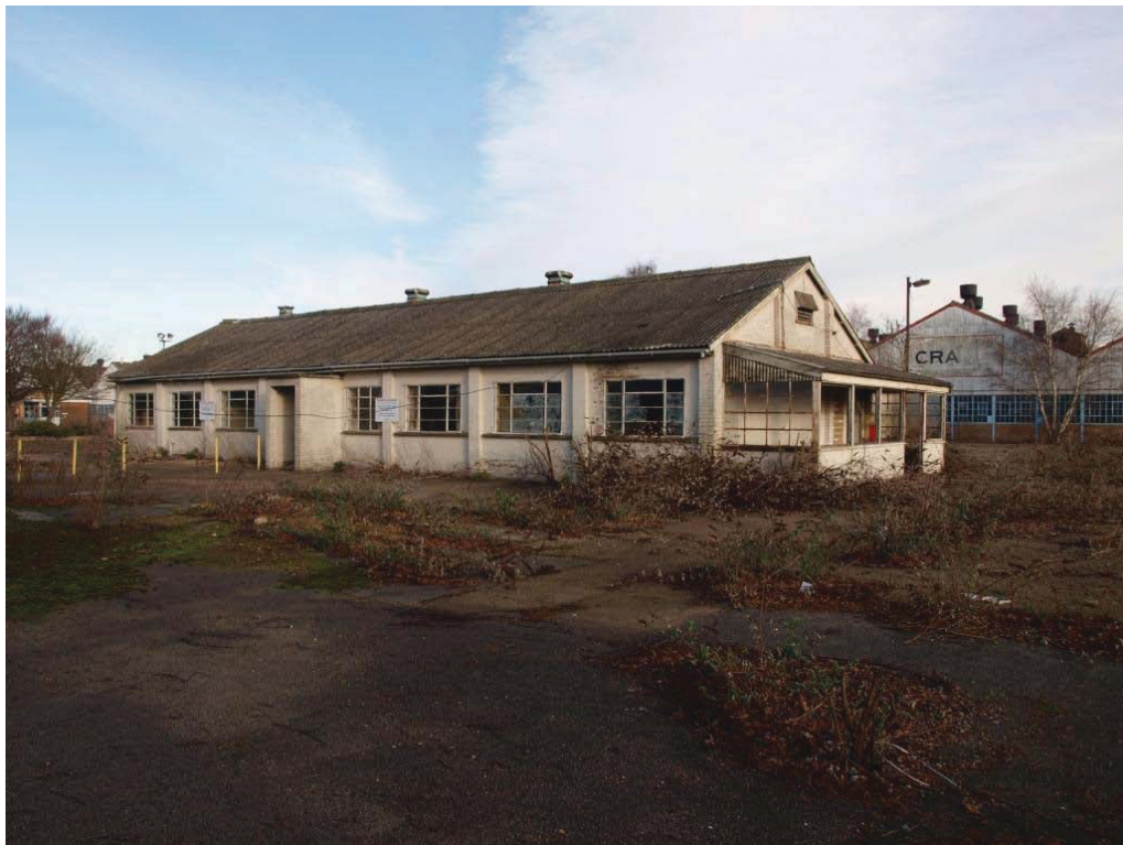
Plate 38. South elevation of Works Pavilion (10).
