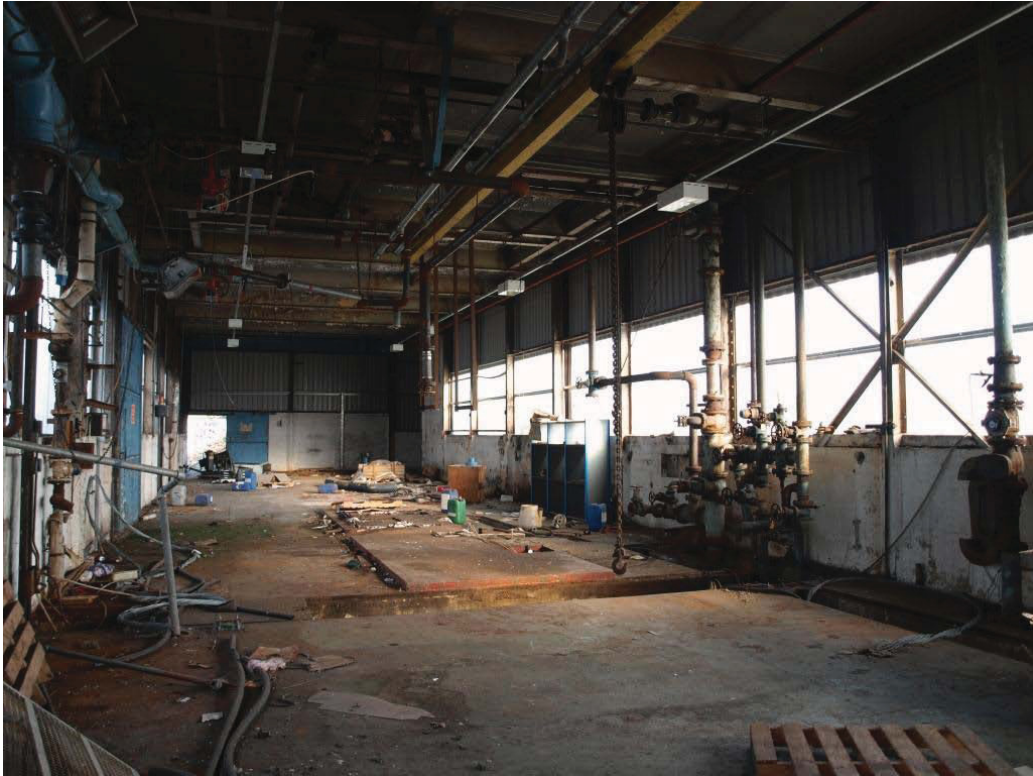
Plate 63. Interior of the Power House looking northeast.
