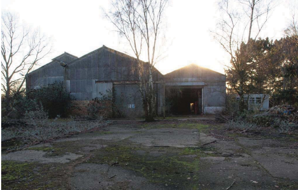
Plate 57. North elevation of Building 18 with office extension shown on the right.
