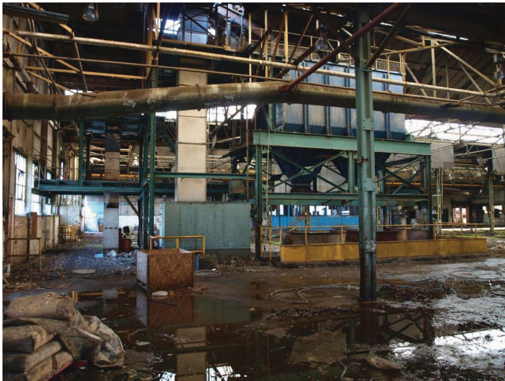
Plate 24. North end of eastern side of the Old Bronze Foundry (5).
