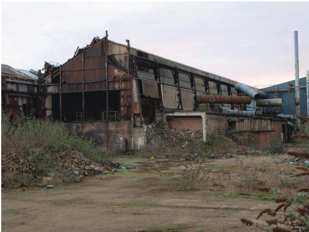
Plate 44. West elevation of Malleable Core Shop (14), looking southeast.
