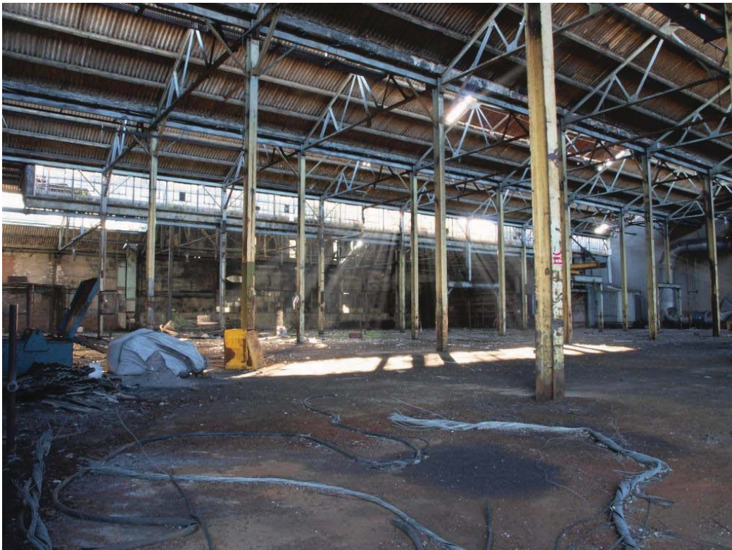
Plate 86. Interior of Old Grey Iron Foundry Building 35 looking southeast.
