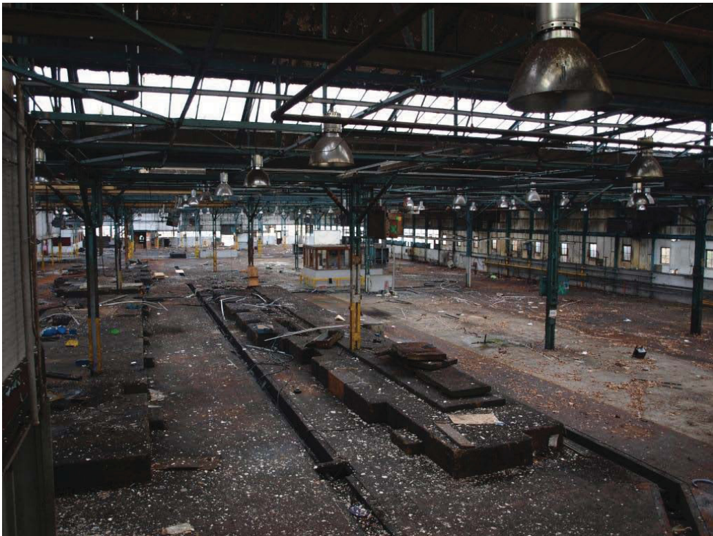
Plate 36. View of raised machine bases in the Union Machine and Assembly Building (7).
