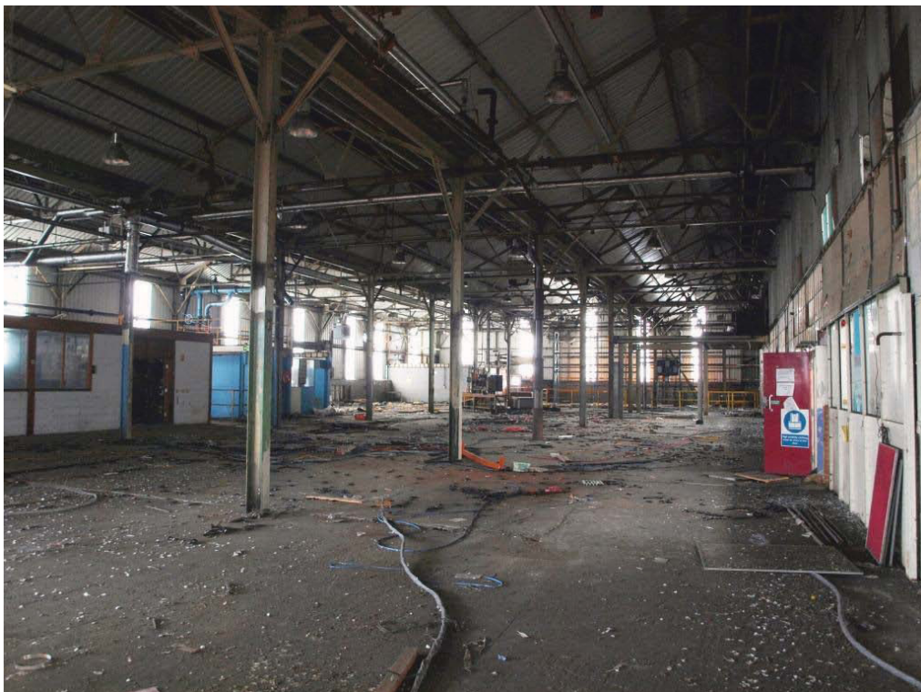
Plate 70. Interior of Building 25 looking south, with mess room on left.
