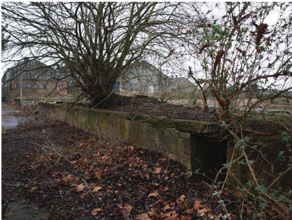
Plate 54. Entrance to Air Raid Shelter 2, looking southwest, two further collapsed air raid shelter entrances are just visible on the left. The vertical concrete face and hard standing above that constrict the shelter entrance were built sometime after the shelters.
