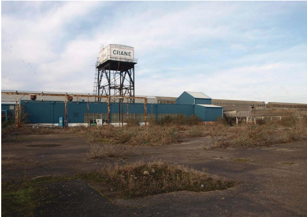
Plate 62. East elevation of the Power House and Water Tower (21). In the foreground is the concrete hard standing where a now demolished foundry building once stood.
