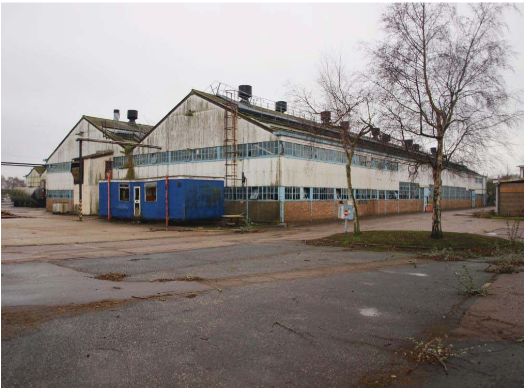
Plate 16. North gables and west elevation of Old Bronze Foundry (5).
