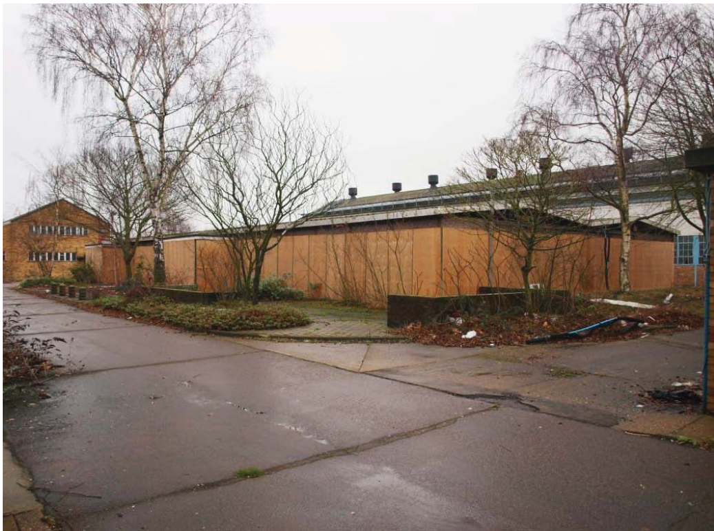
Plate 26. West and south elevations of I.T. Offices (6), formerly canteen buildings.
