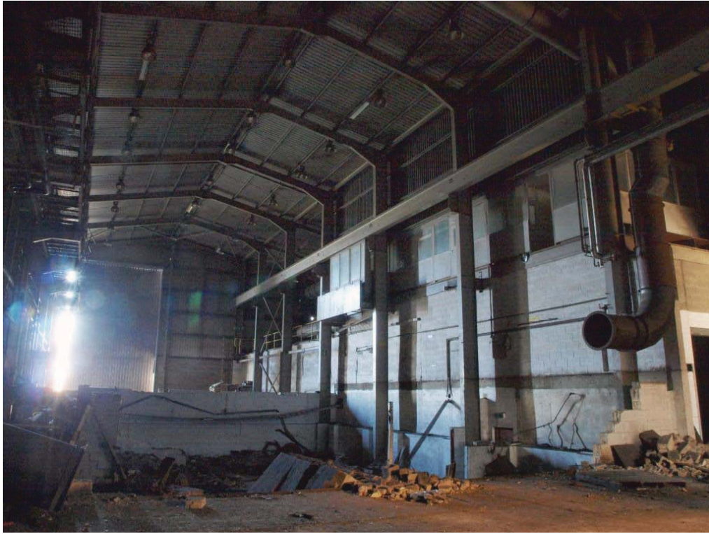
Plate 43. Electric Melt Building (13) looking northeast.
