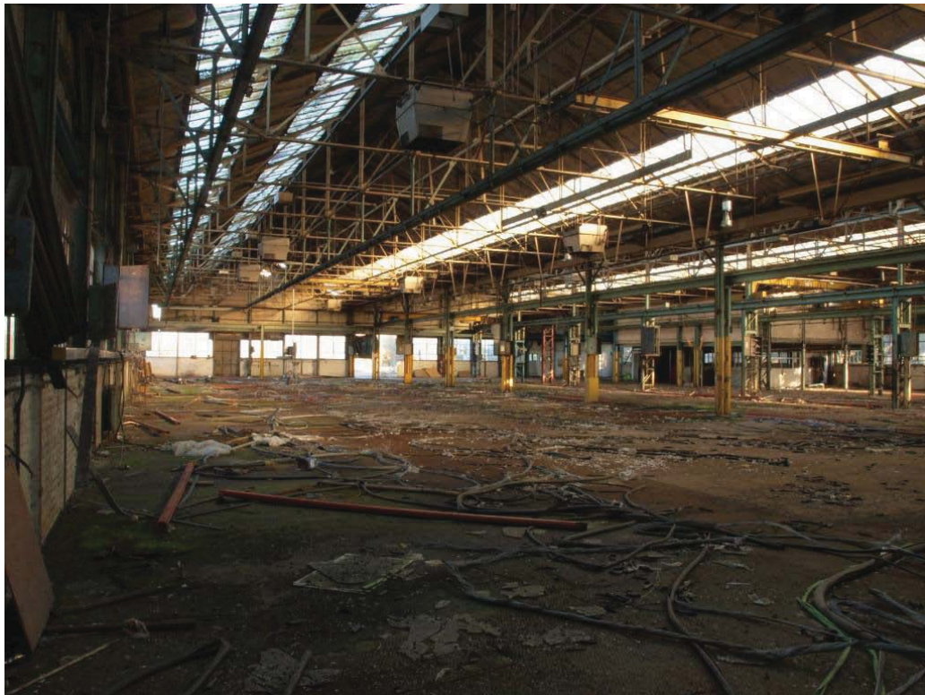
Plate 56. Interior view of Building 17, looking northeast.
