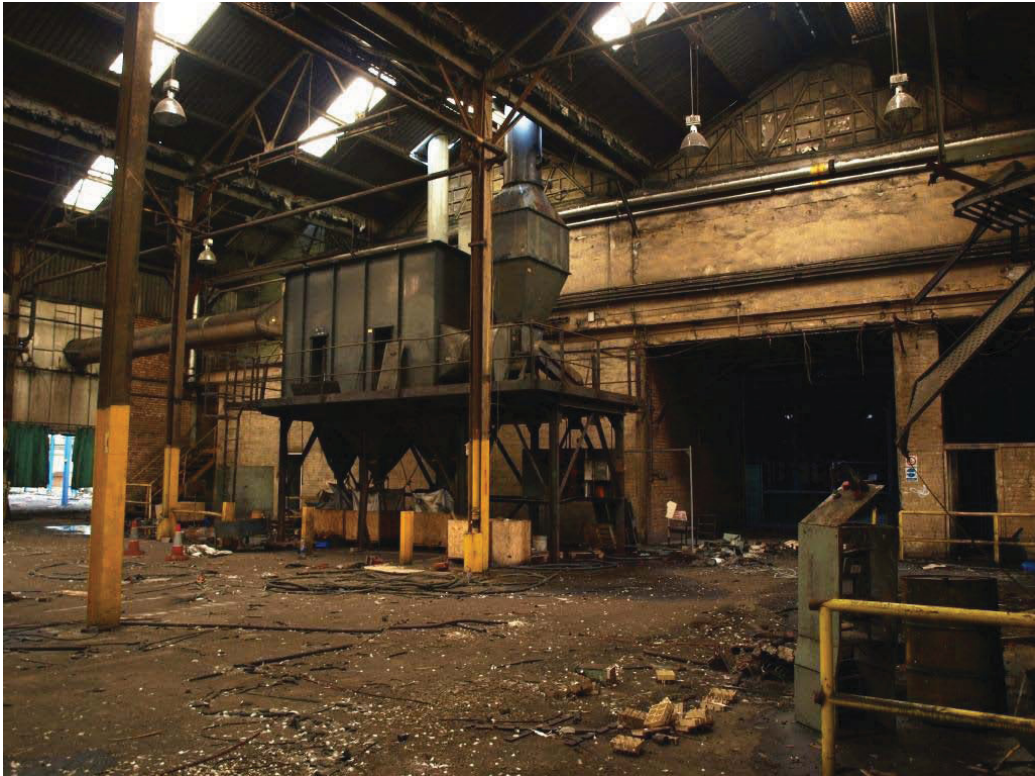
Plate 83. Interior of Building 34 looking south.
