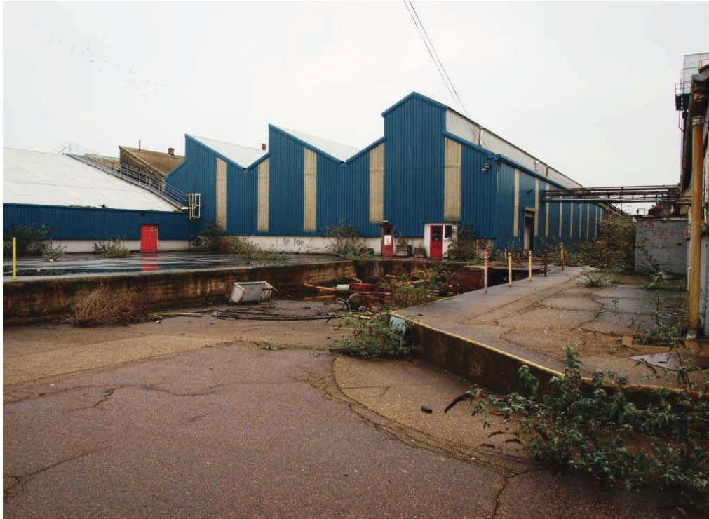
Plate 69. South and east elevation of Building 25.
