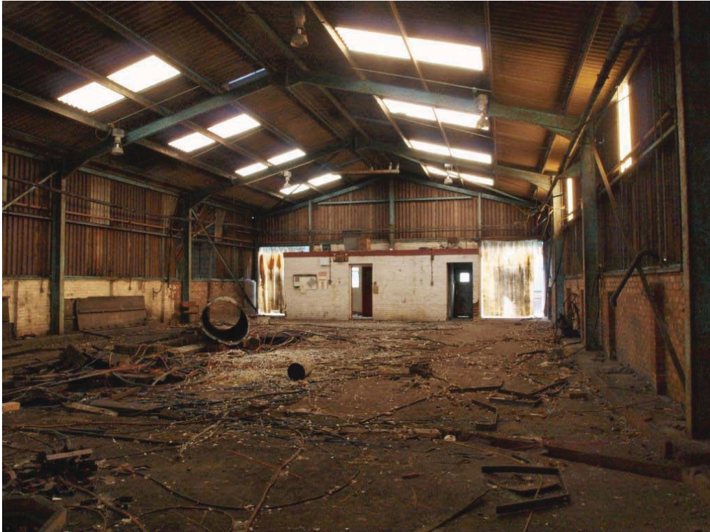
Plate 41. Interior of Ex Piddling Building (11) looking east.
