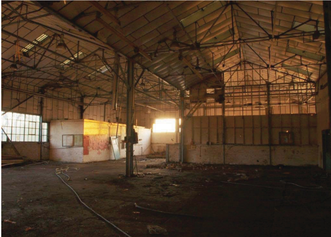
Plate 59. Interior of Building 18 looking south.
