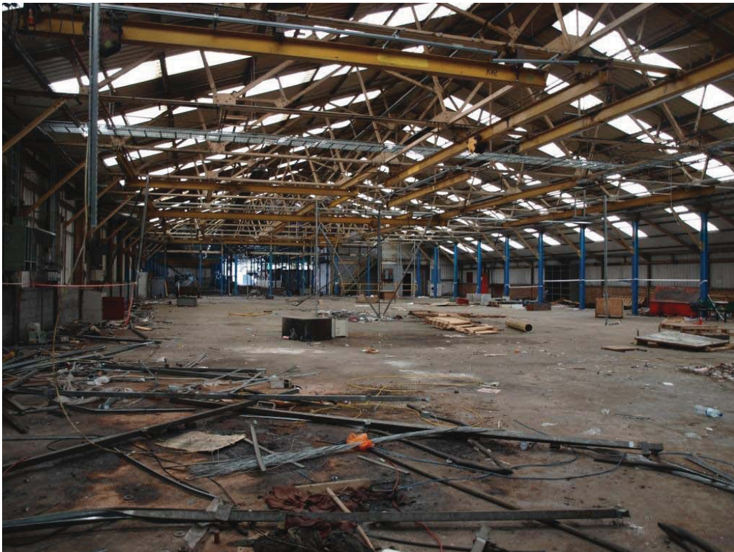
Plate 80. Interior of Building 31 looking northeast.
