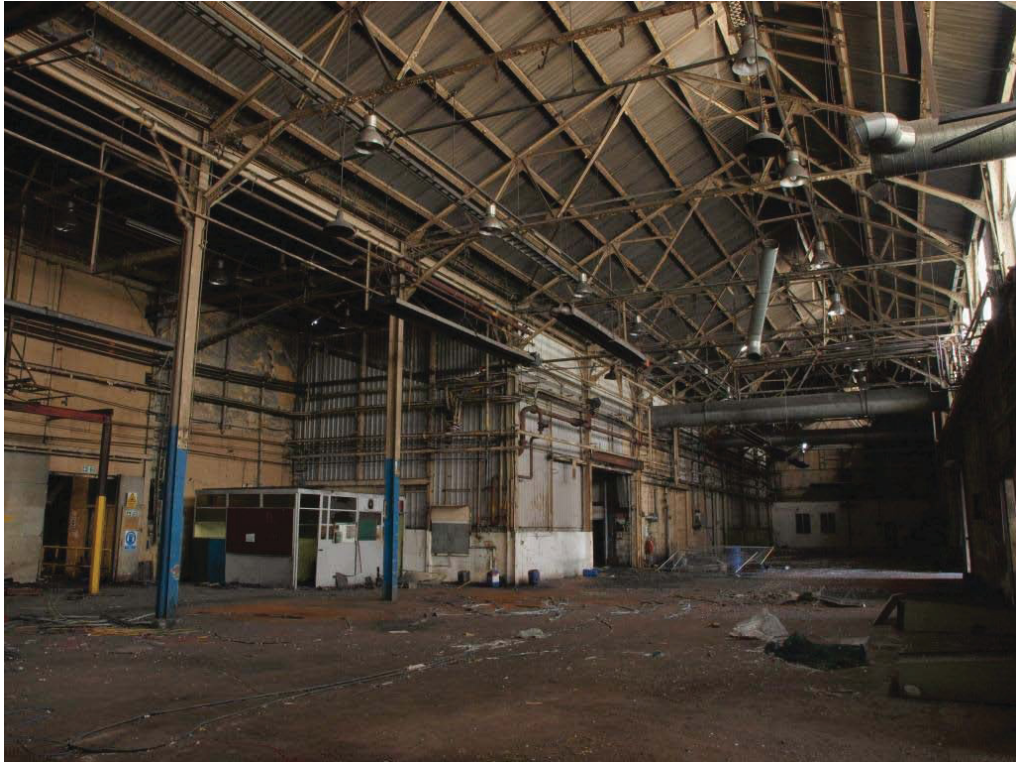
Plate 45. Interior view of Malleable Core Shop (14) looking southeast.
