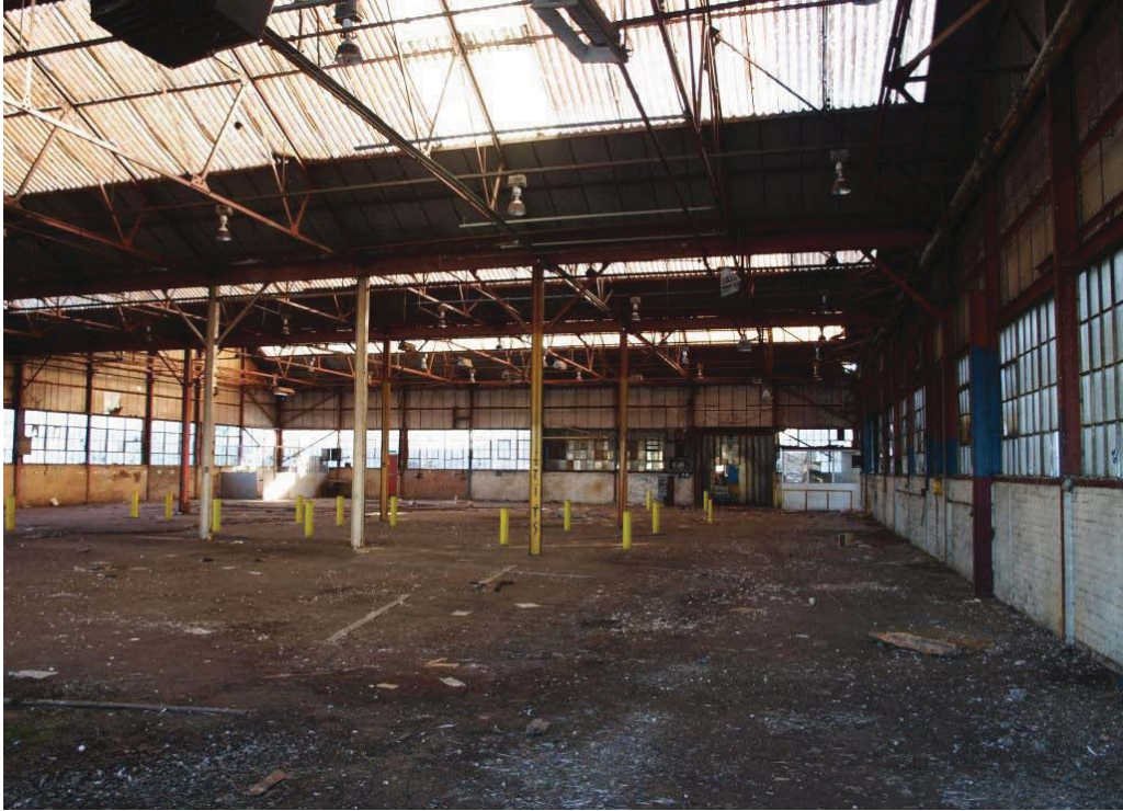
Plate 49. Interior view of Building 16 looking east.
