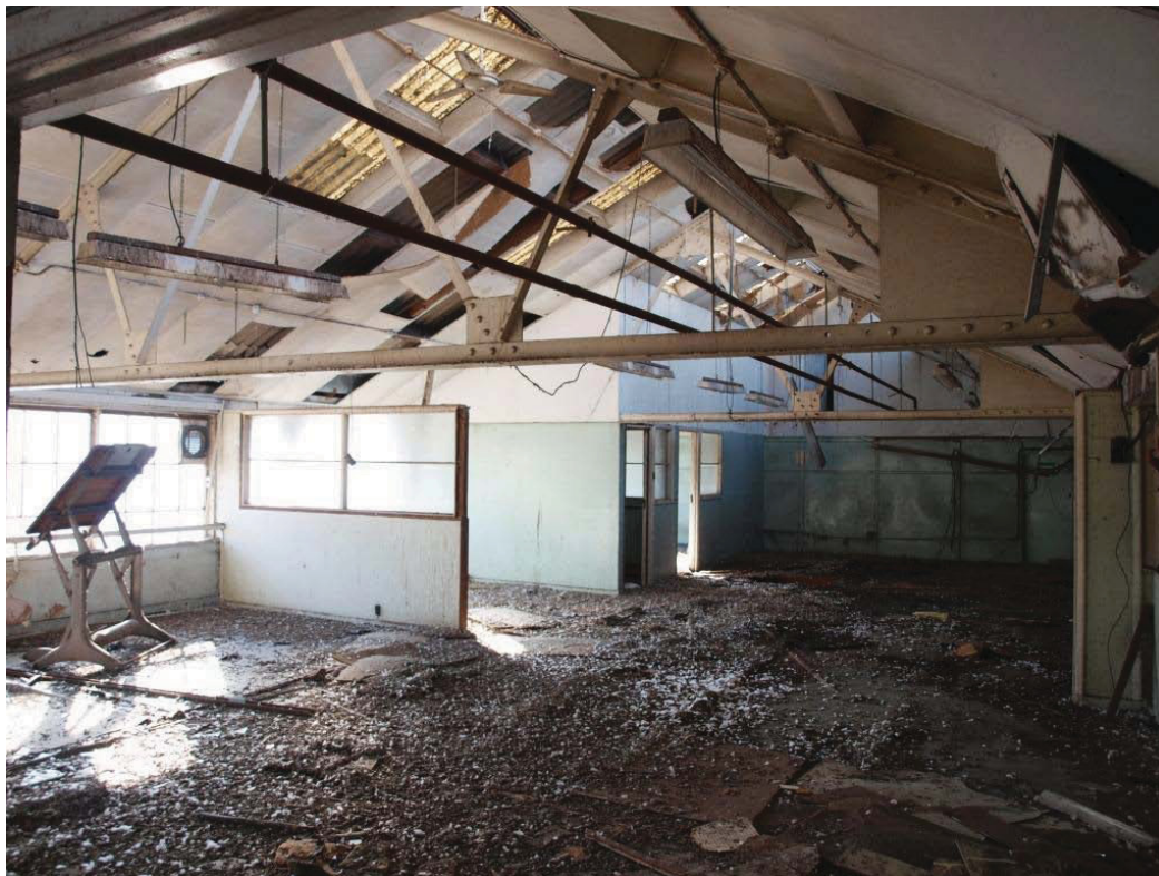
Plate 76. First floor office in Building 27 looking south.
