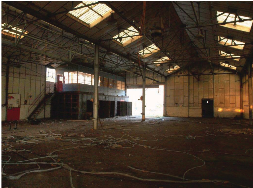
Plate 58. Interior of Building 18, looking north with storage and office.
