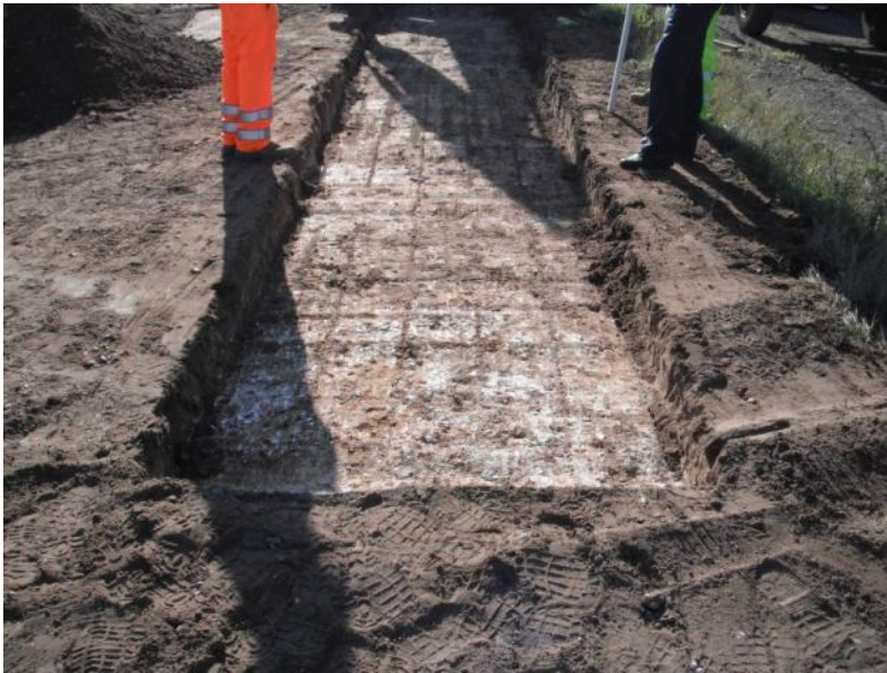
Plate 4: Western end of southern trench for cabin base
