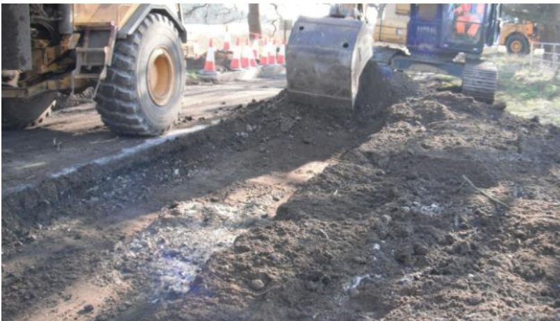
Plate 41: Widening eastern side of track
