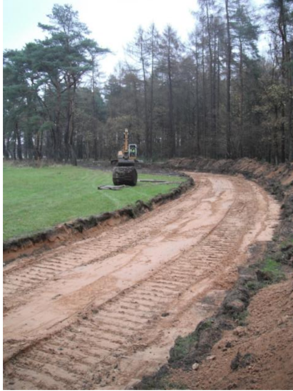
Plate 30: Final bend of New Track 3
