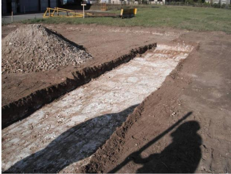
Plate 5: View southwest. Western end of northern trench for cabin base
