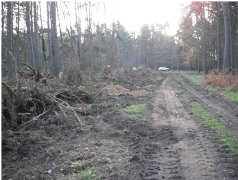
Plate 28: View South through woodland to final bend of New Track 3
