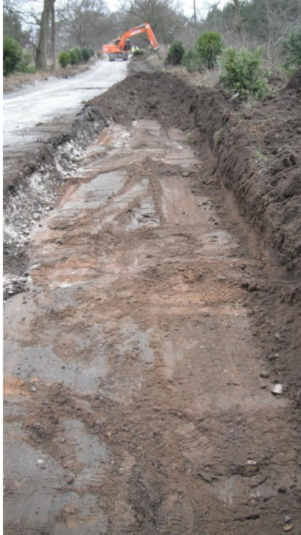
Plate 43: Widening western side of track. View south
