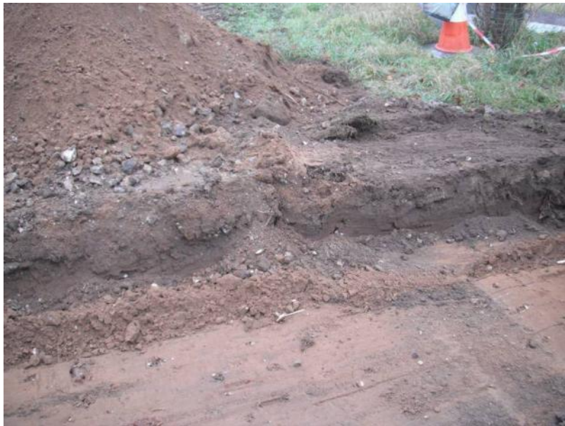
Plate 7: Topsoil removed onto silty-sand subsoil
