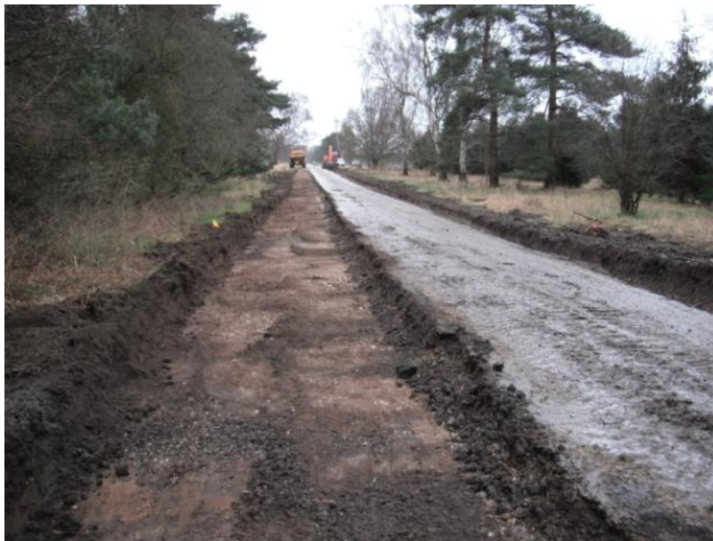
Plate 45: View North showing track widening
