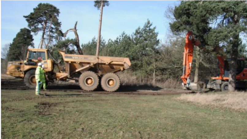
Plate 38: Work in progress: View West
