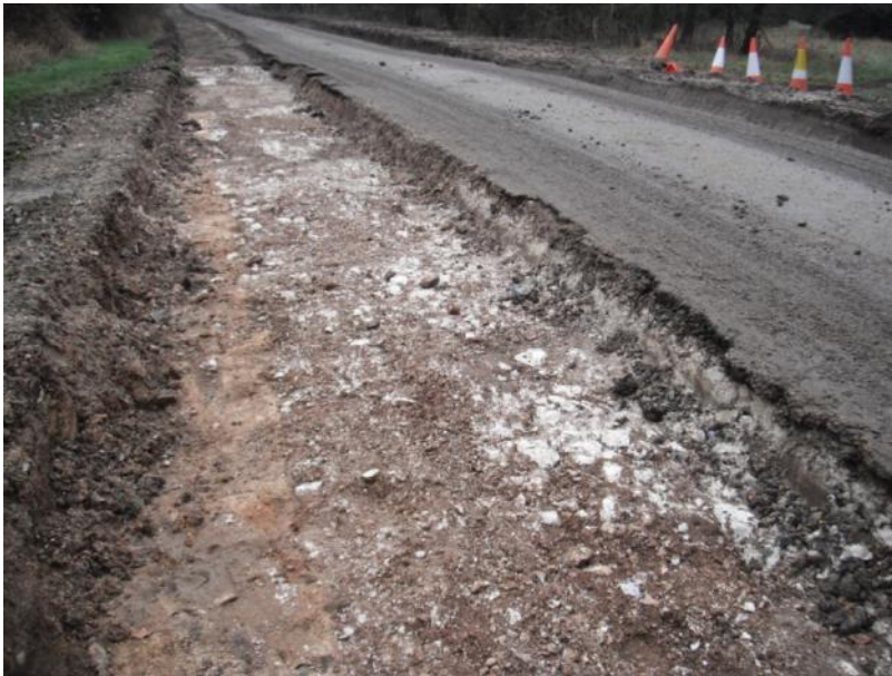
Plate 47: Chalk rubble forms part of existing track. BT service run visible to left of picture
