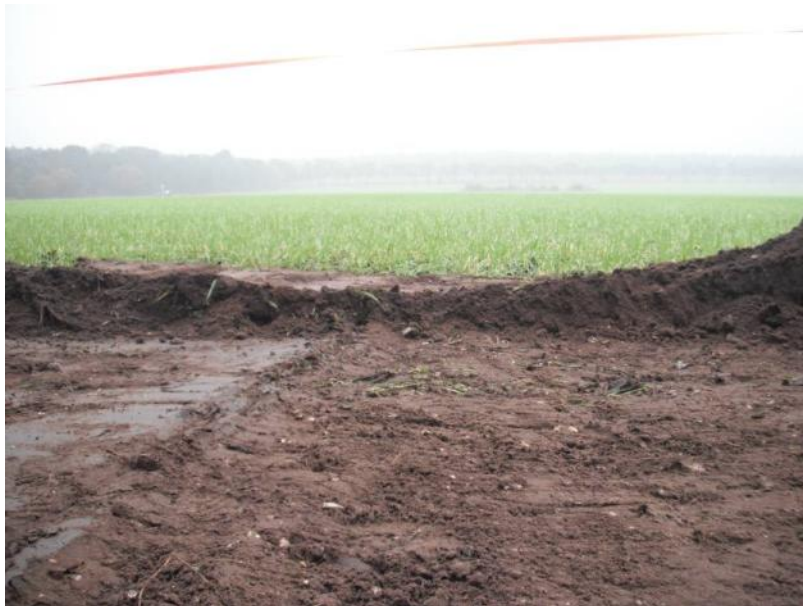
Plate 10: H18 View North – ground reduction very minimal in places. Here it is less than 0.10m
