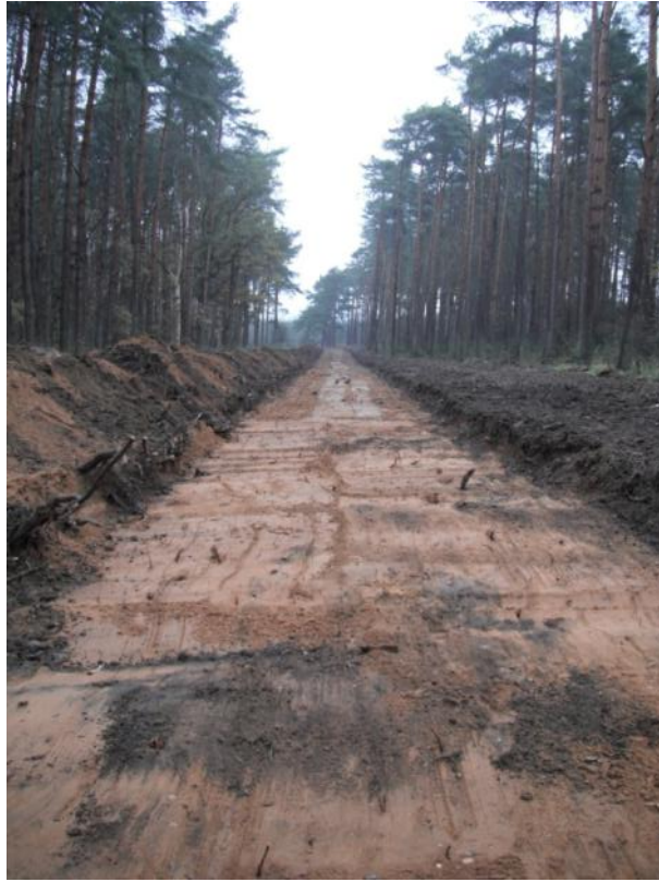
Plate 29: View South through woodland after machining
