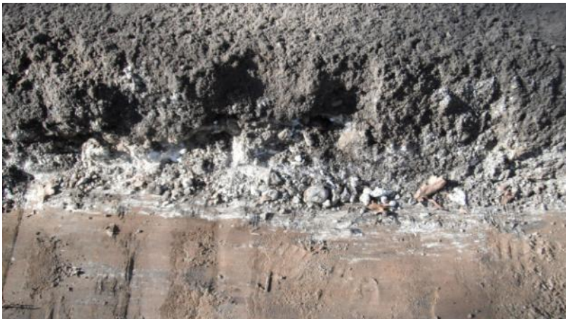
Plate 39: Section of existing track
