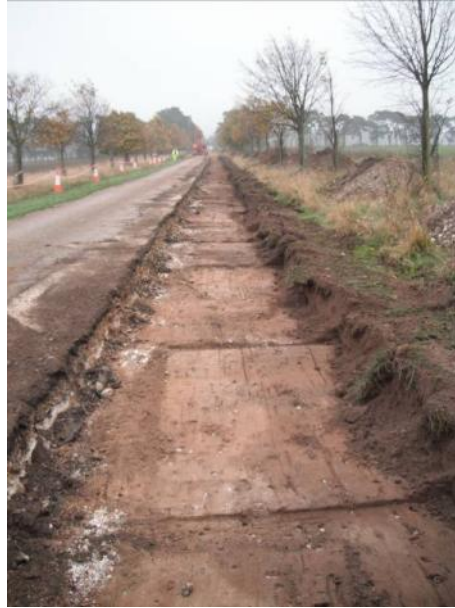
Plate 8: View east along widening trench
