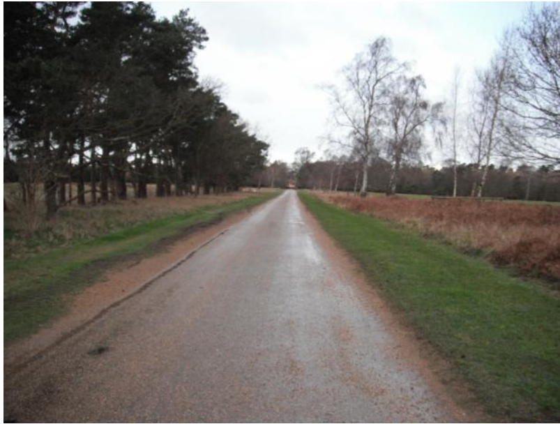
Plate 44: View South along existing track
