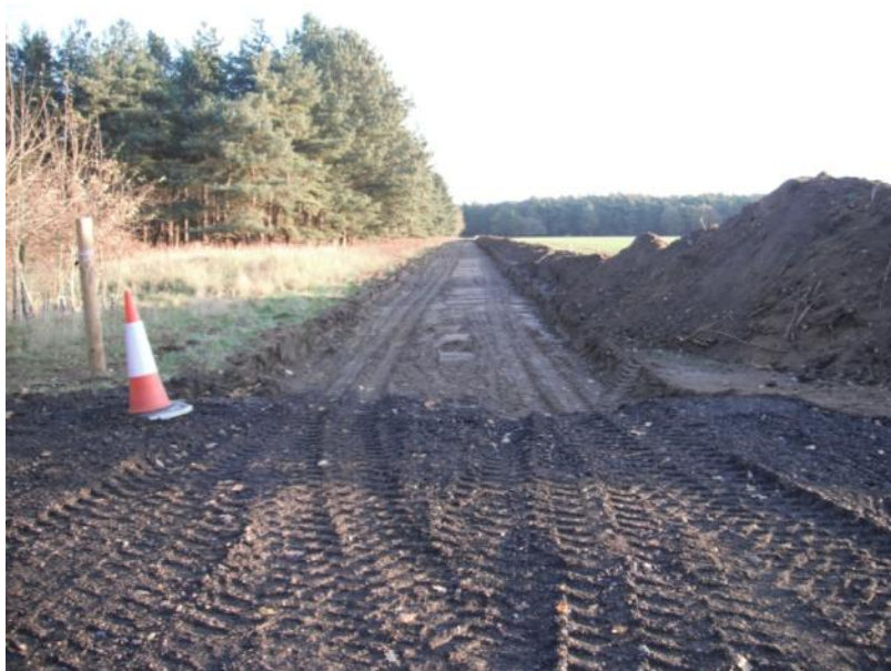
Plate 19: View North-East from start of New Track 3
