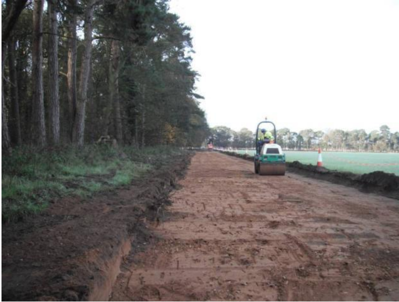
Plate 11: Middle section of T68 looking West
