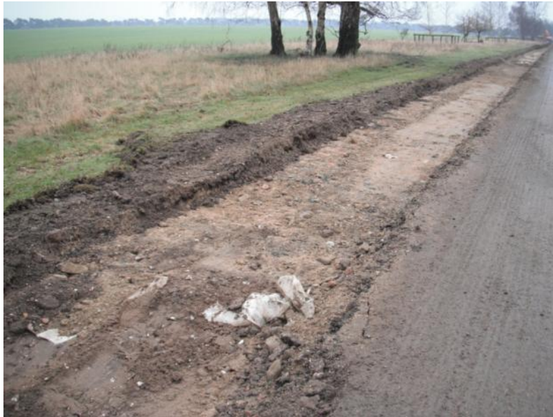
Plate 48: 100m of modern rubble each side of existing track
