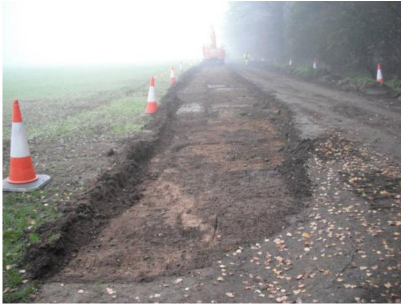
Plate 9: Removal of plough soil. H18 view East
