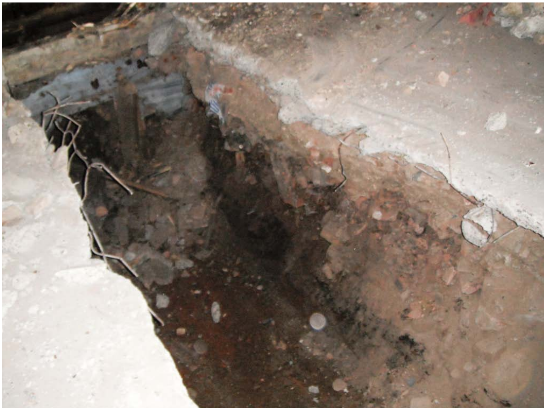
Plate 5. West side of Trench 2 looking west, showing rubble backfill and reinforced concrete cap against edge of timber deck.
