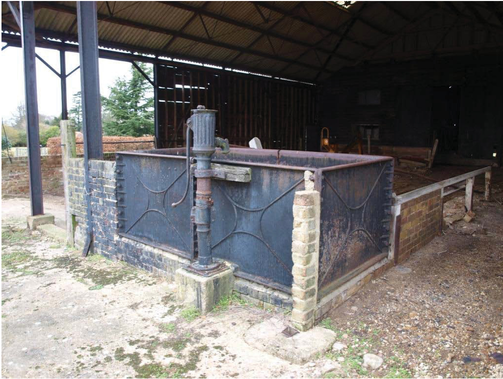
Plate 23. Water tank and hand pump found on the south-west side of Building 4.
