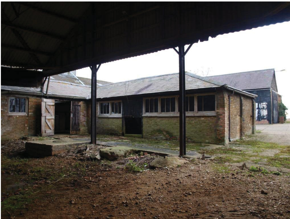
Plate 14. North elevation of south wing of Building 2.
