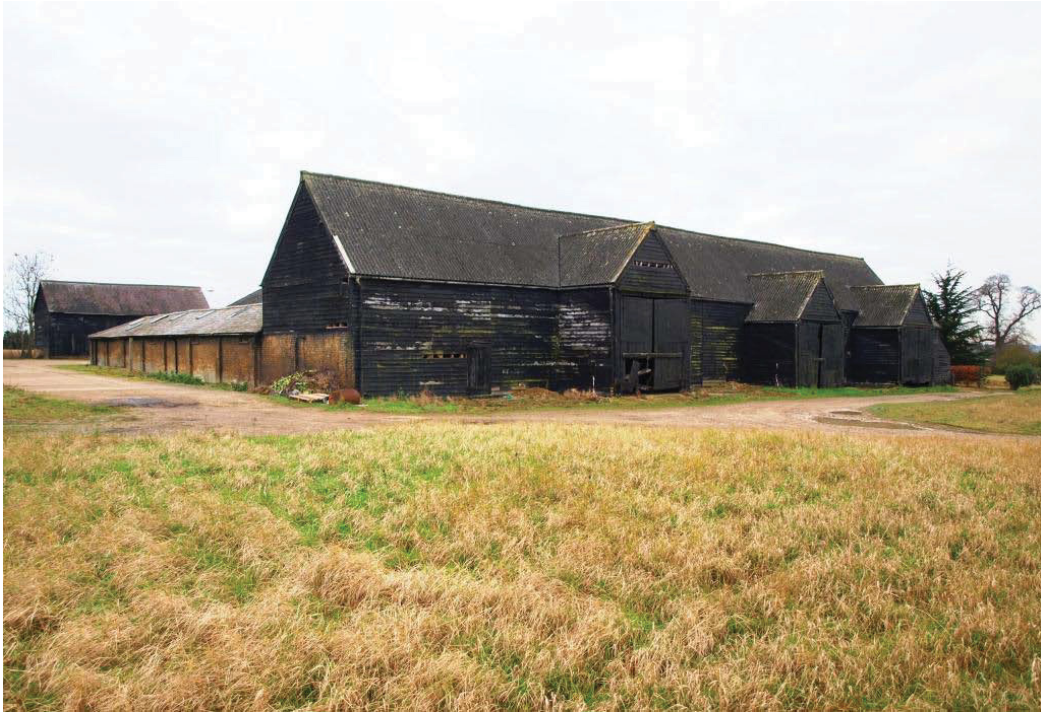
Plate 3. North and east elevations of Building 1, with the east elevation of the single storey brick Building 2 extending to the rear and beyond it Building B.
