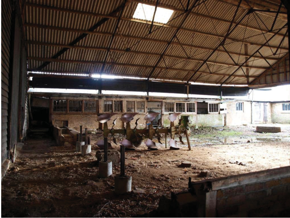
Plate 13. West elevation of Building 2 viewed from covered yard of Building 4.
