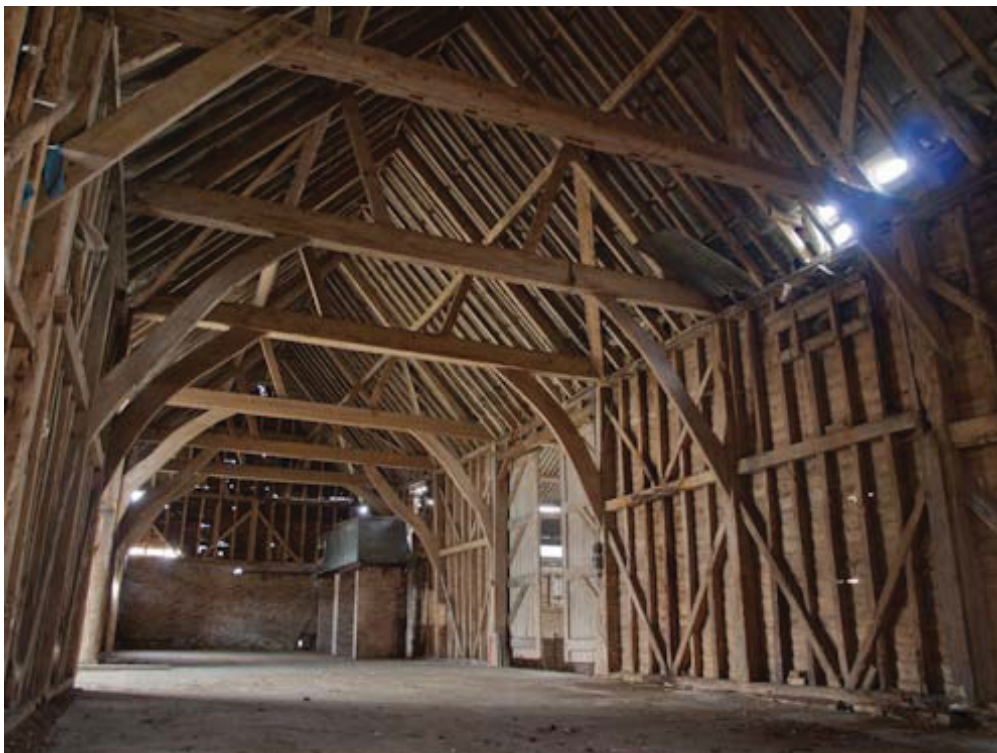
Plate 9. Interior view of east end of Building 1 looking south-east.
