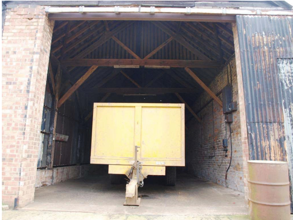
Plate 31. Interior of Building B showing timber roof trusses, braces and different methods of wall construction.
