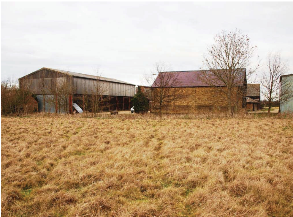
Plate 26. Buildings A (left) and B (right) viewed from the south.
