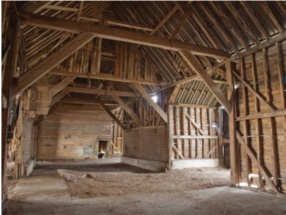
Plate 8. Interior view of west end of Building 1 looking north-west.
