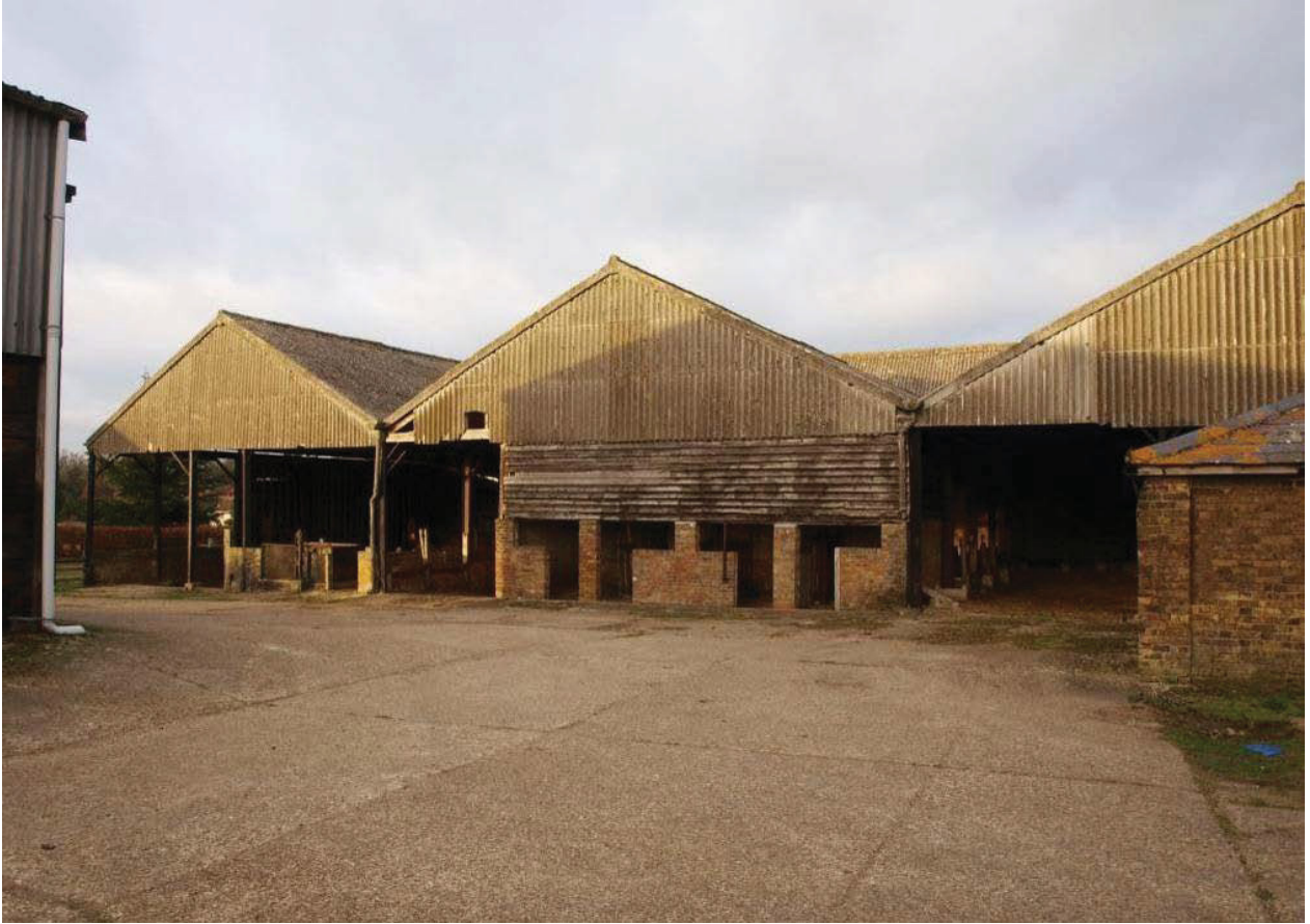
Plate 20. South elevation of Building 4 and modified brick front to the pig sties of Building 3.
