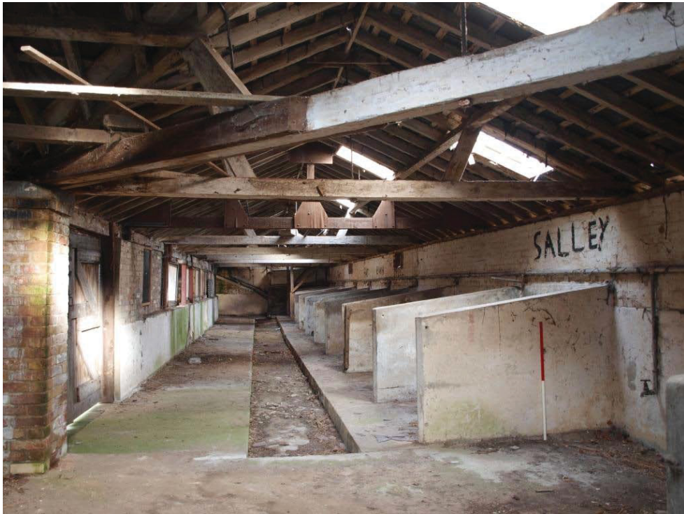
Plate 16. Interior of Building 2 looking north.
