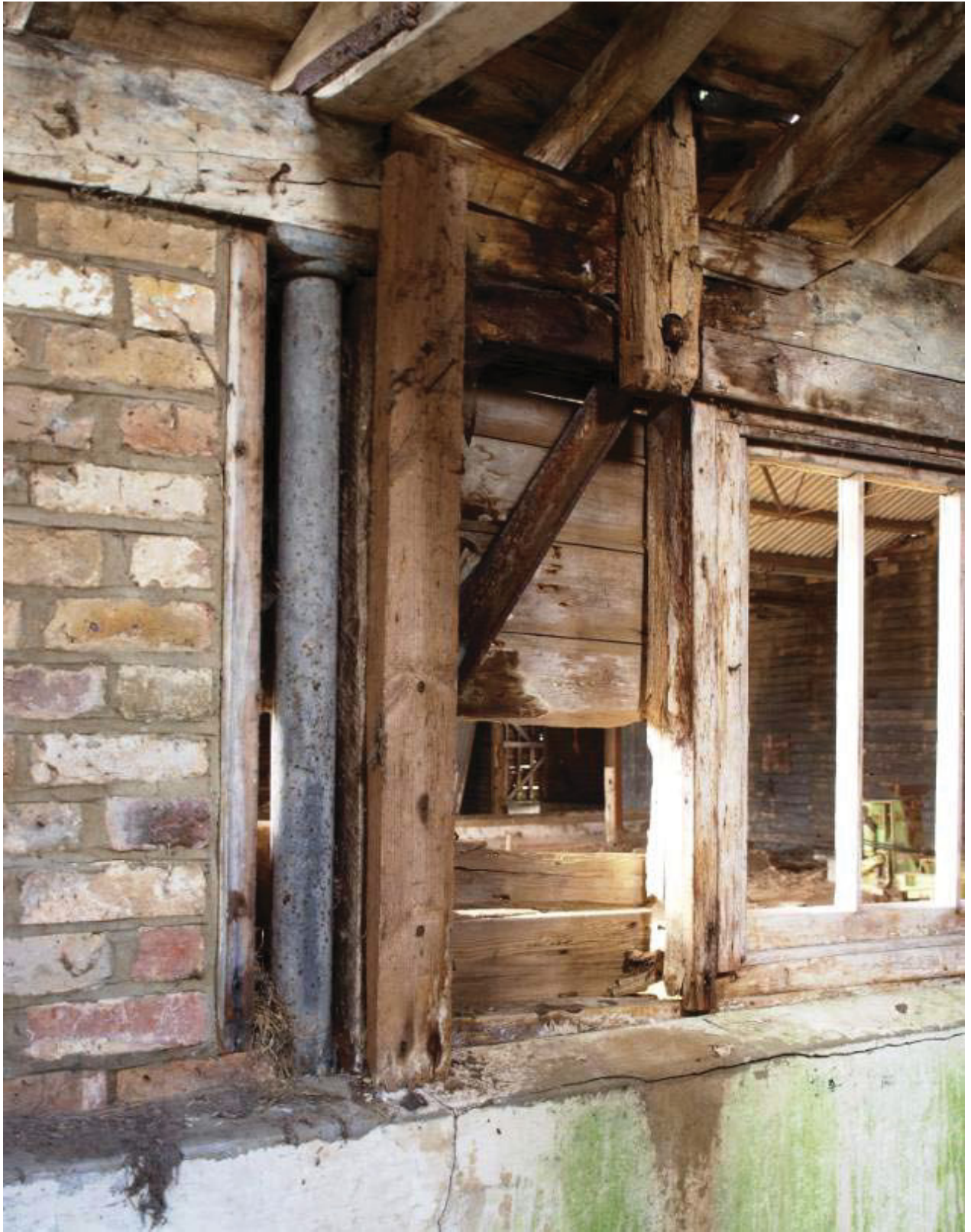
Plate 19. Cast iron column partially encased in west wall of Building 2.
