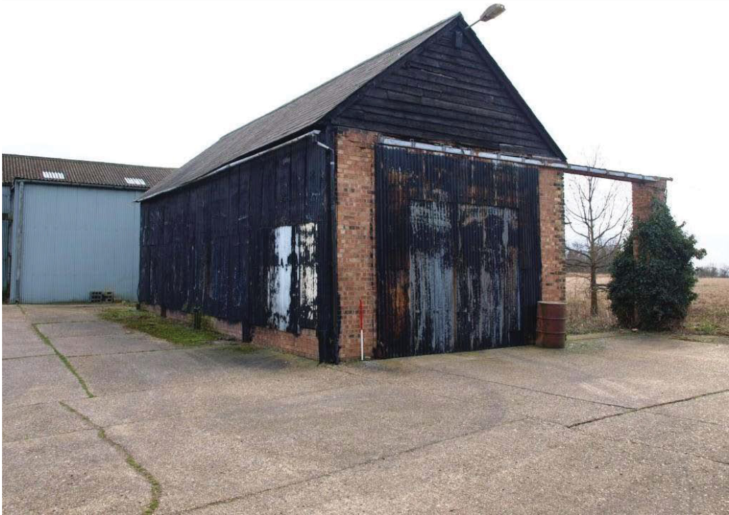
Plate 29. North and west elevations of Building B.
