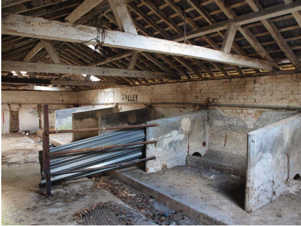
Plate 15. Interior of south wing of Building 2.
