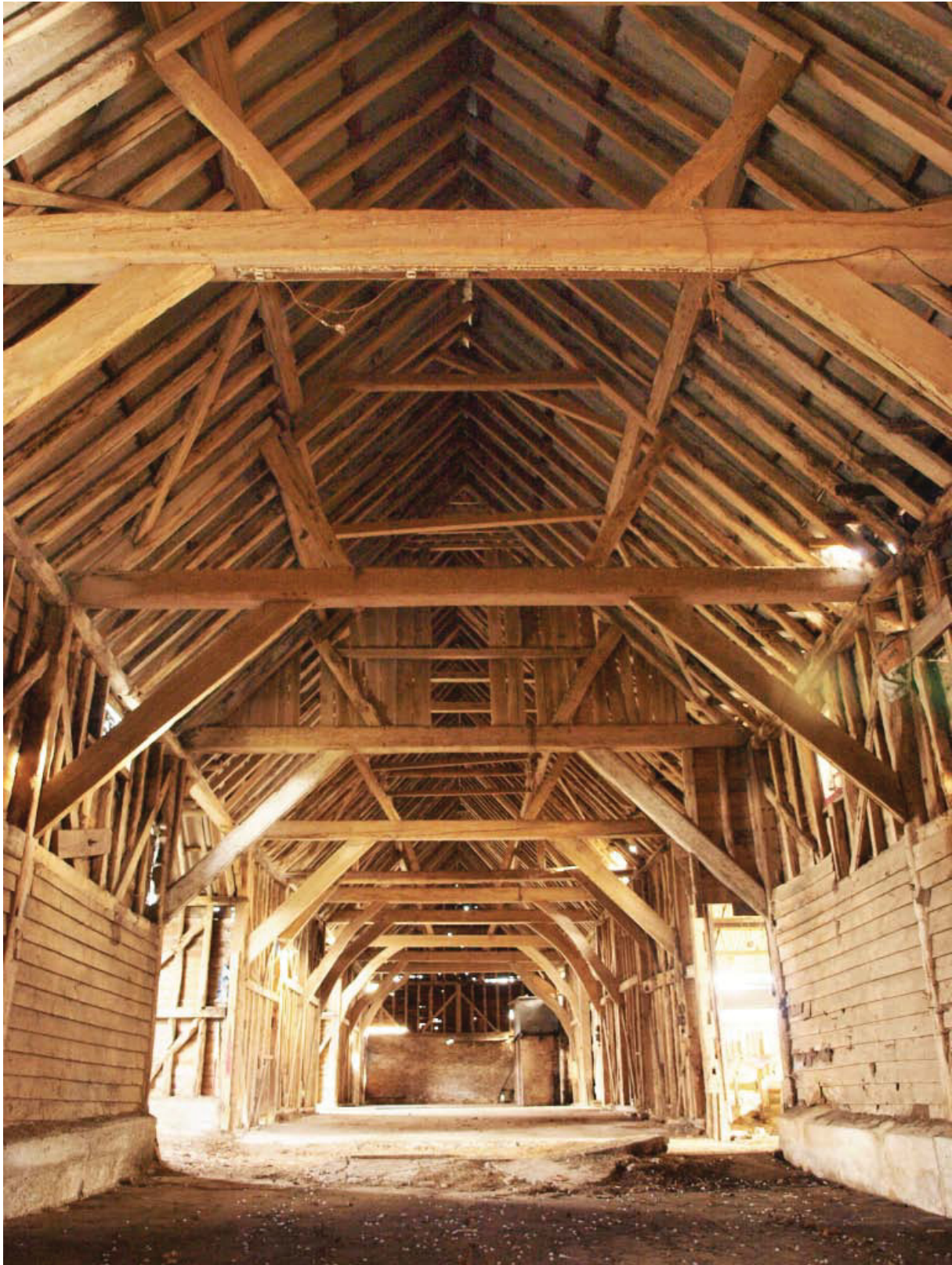
Plate 7. Interior view of Building 1 looking east from west end.
