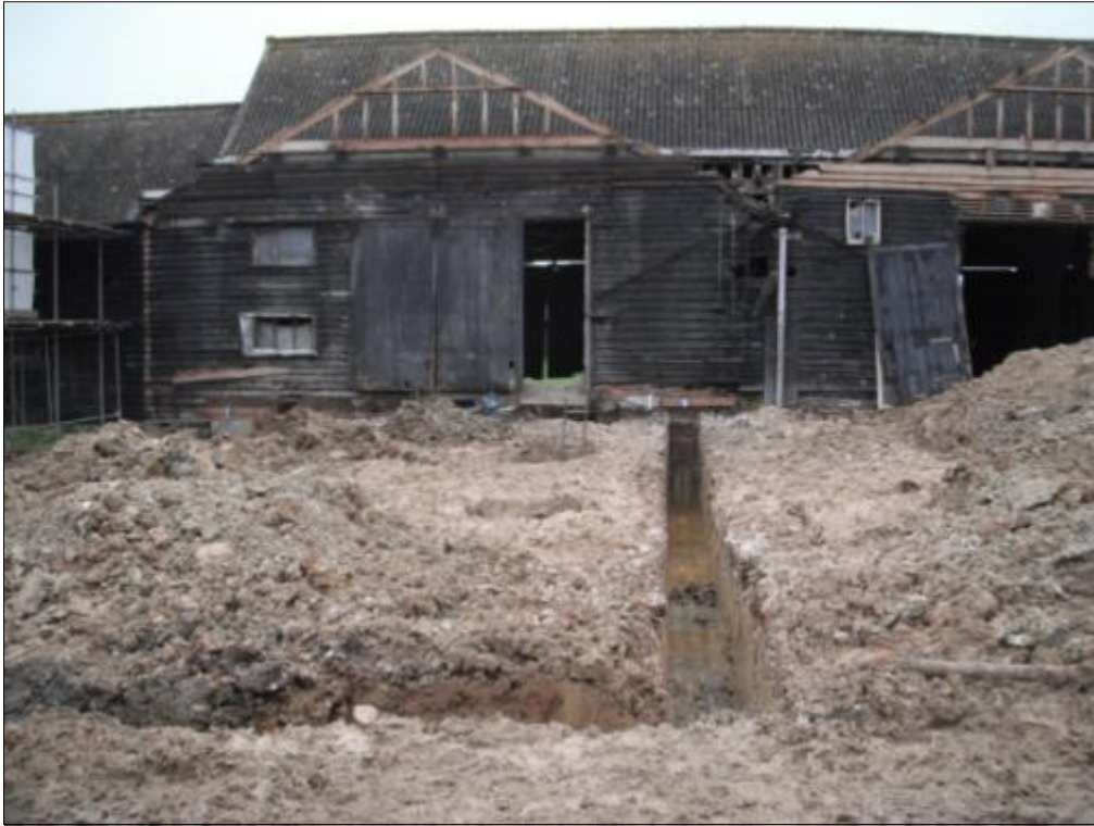
Plate 7: Eastern foundation trench and pad footings, new build extension, looking north
