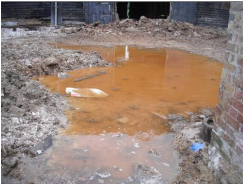
Plate 2: Farmyard following slab removal, looking north
