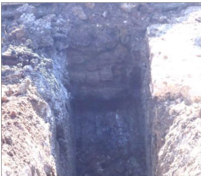
Plate 11: Wall footing [58] in courtyard building south foundation trench, looking east
