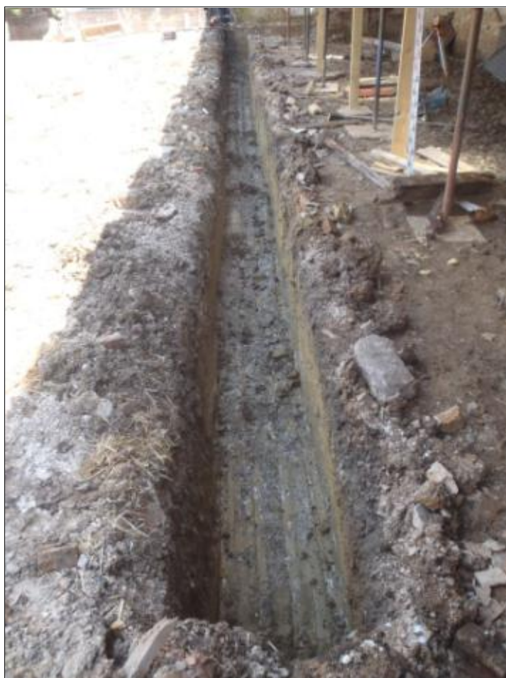
Plate 13: Piggery foundation trench, looking north
