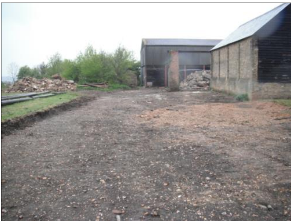
Plate 4: Topsoil stripping behind Building B, looking west
