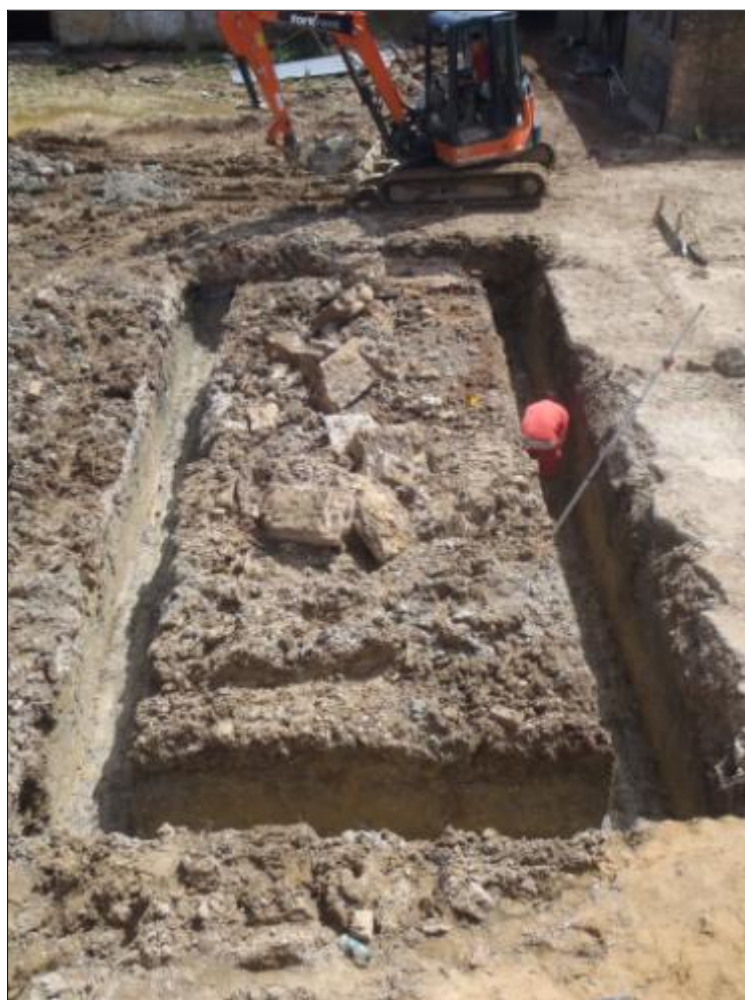
Plate 10: Courtyard building foundation trench, looking east
