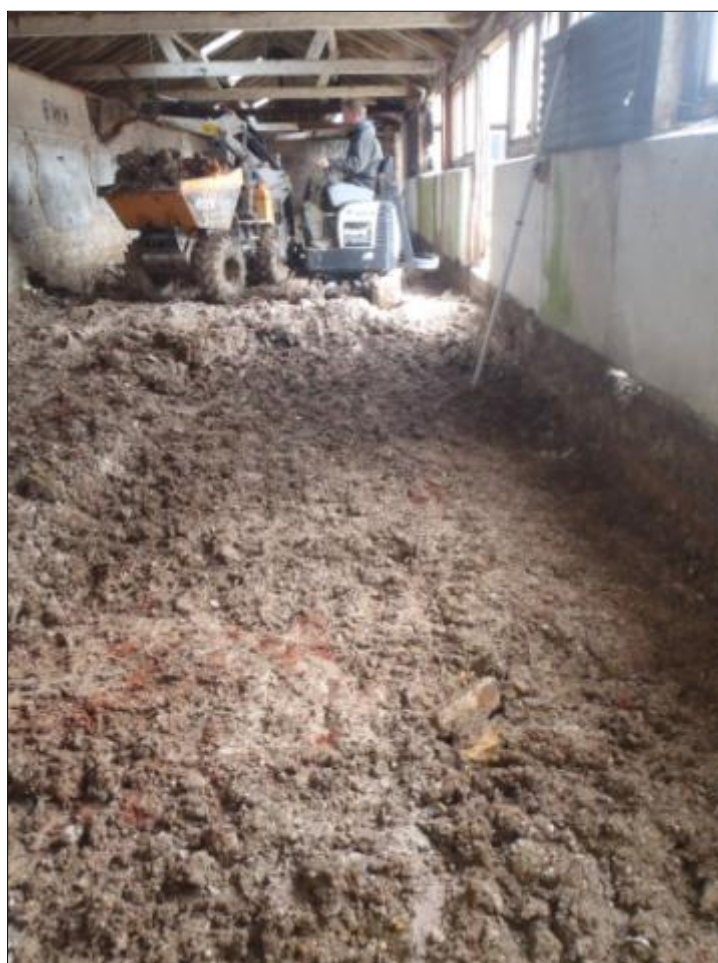
Plate 12: Ground reduction in the piggery, looking south
