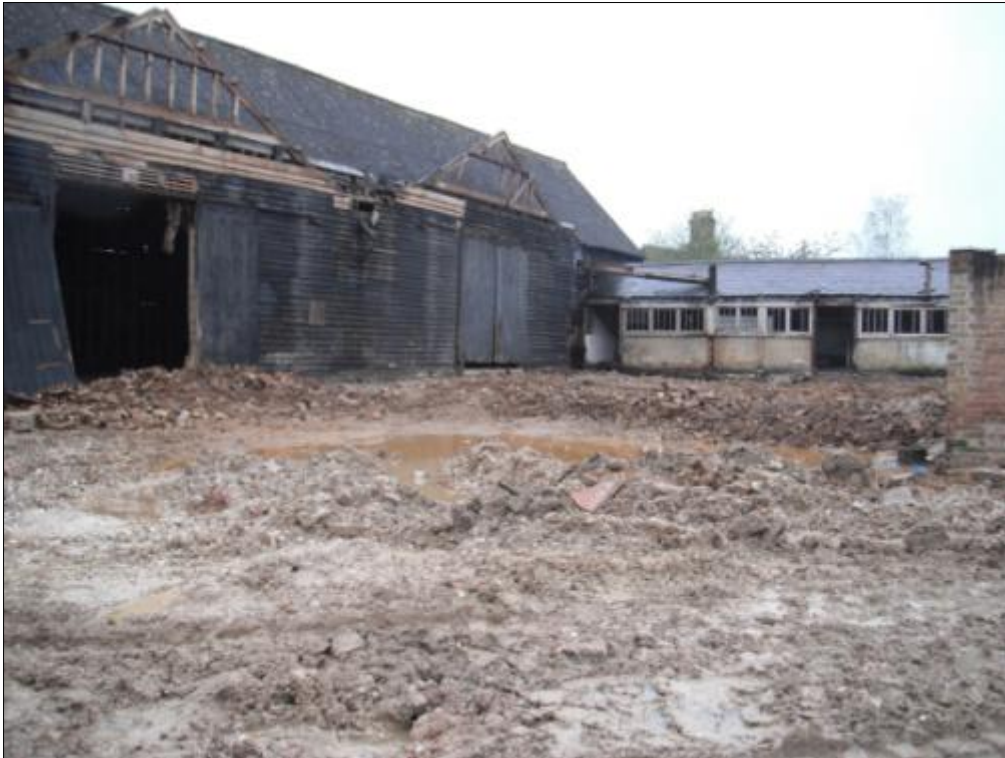
Plate 1: Farmyard following slab removal, looking north-east
