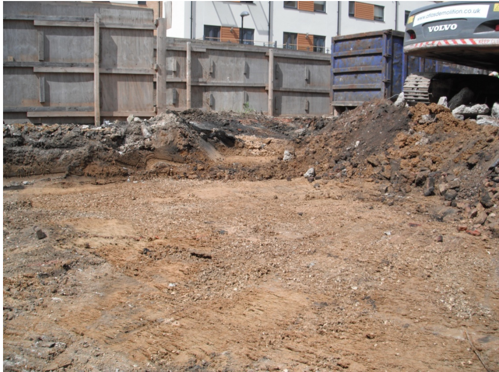
Figure 8: North Facing Shot of Phase 2 Excavation
