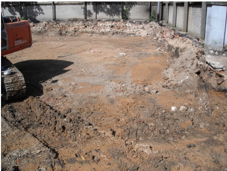
Figure 9: West Facing Shot of Phase 2 Excavation
