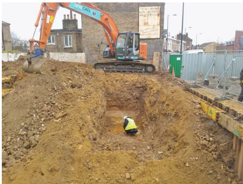
Plate 1: Investigation of natural deposits during excavation of Trench 3, looking west.
