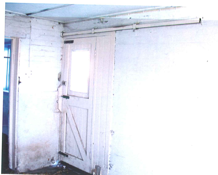
Plate 2: Interior of farmhouse showing previous double doors
