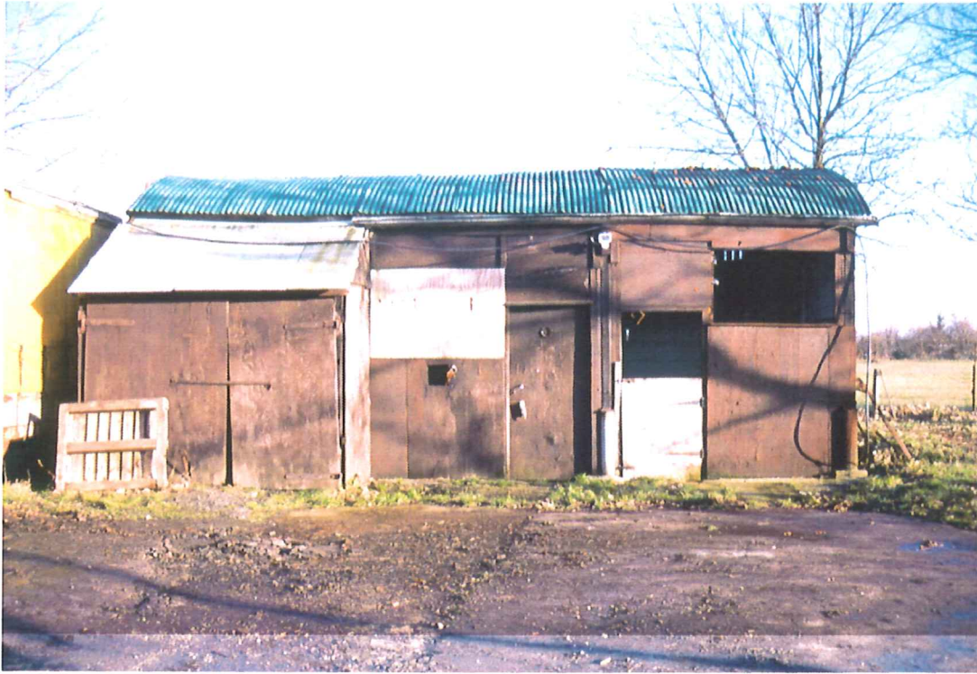
Plate 3: West facing elevation of dutch barn
