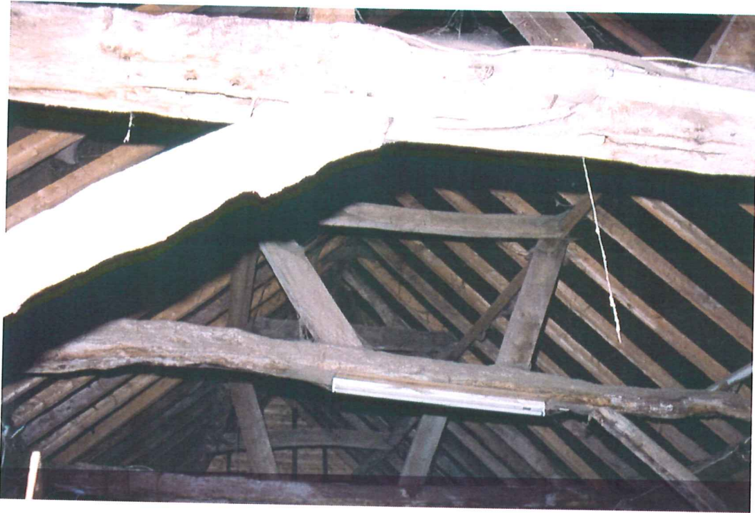
Plate 5: Roof trusses in timber barn
