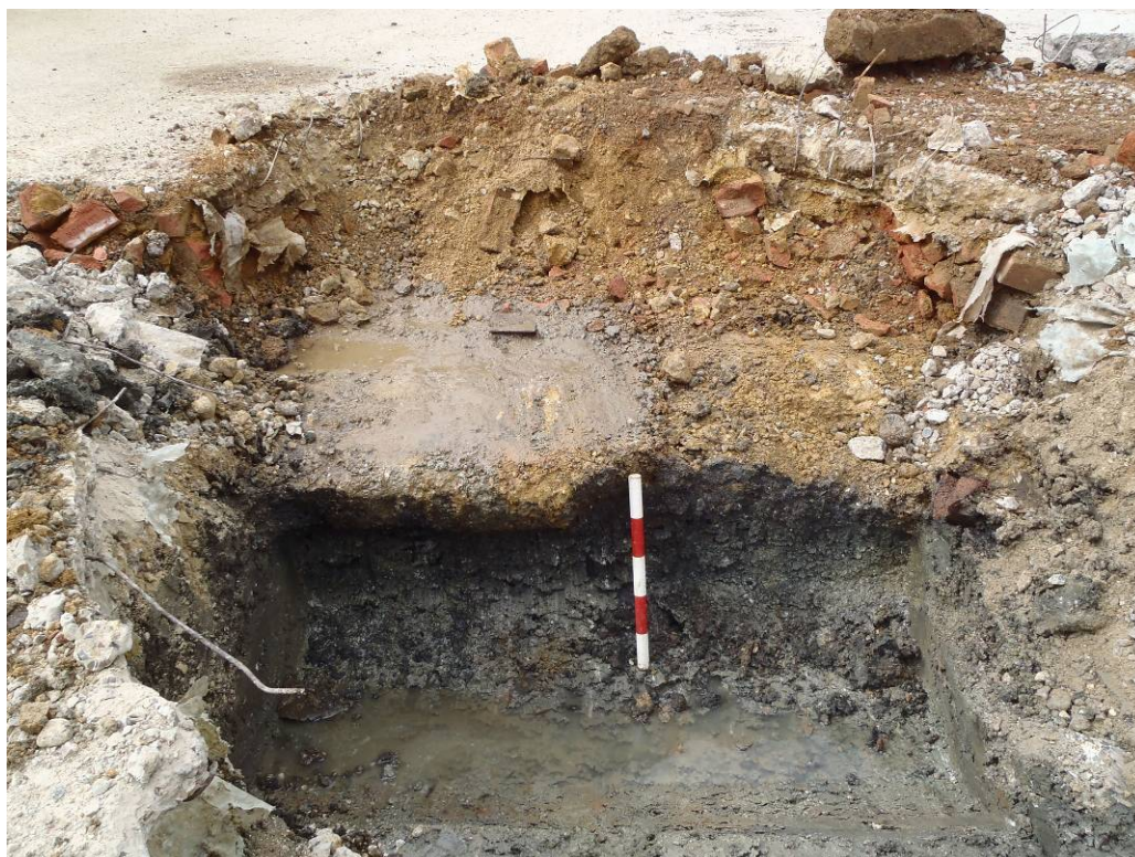
Plate 13. Trench 4 south west end. Concrete wall foundations for 20 th century factory building
