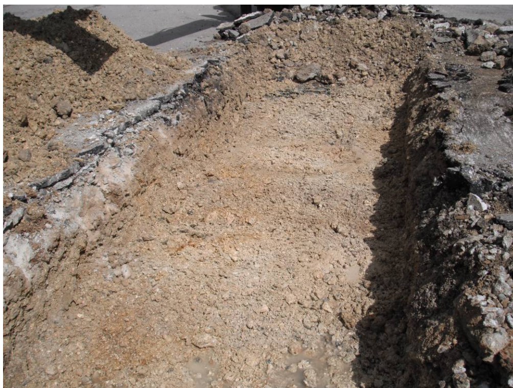
Plate 8. Trench 3 Natural gravel (12) immediately under hard-standing
