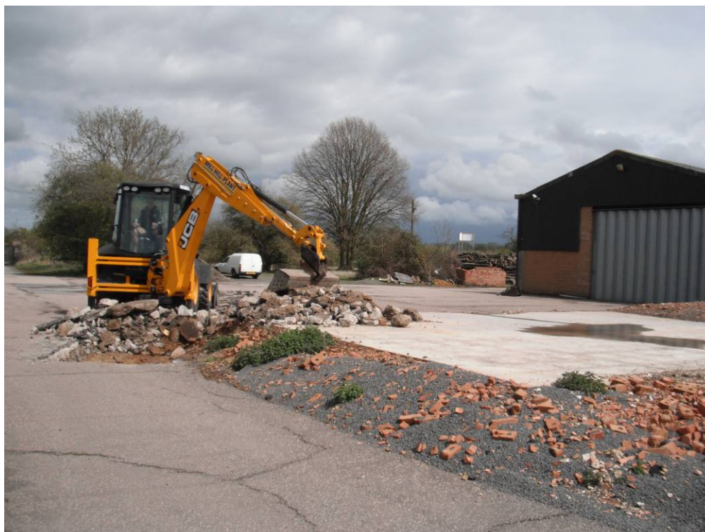
Plate 7. Removal of hard-standing Trench 3 View North-East
