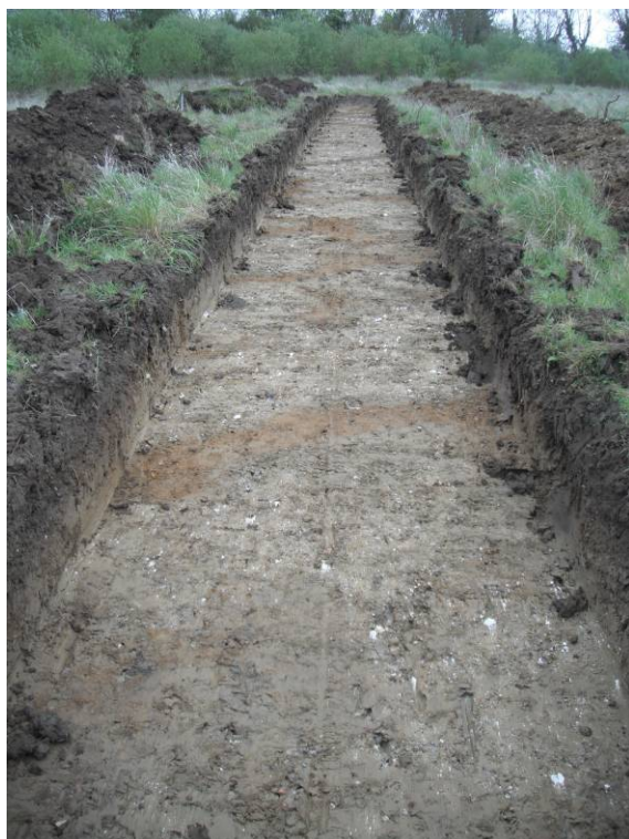
Plate 9. Trench 7. View NE.
