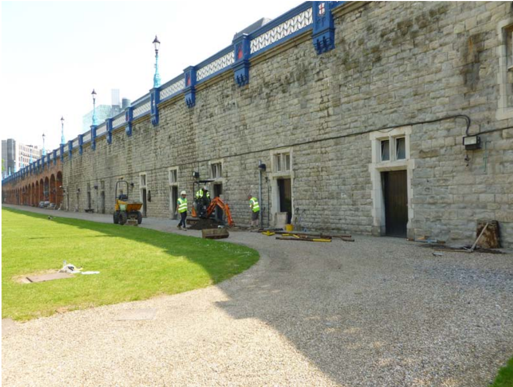
Plate 1: View NE of area of Trench 1 adjacent to Tower Bridge Approach
