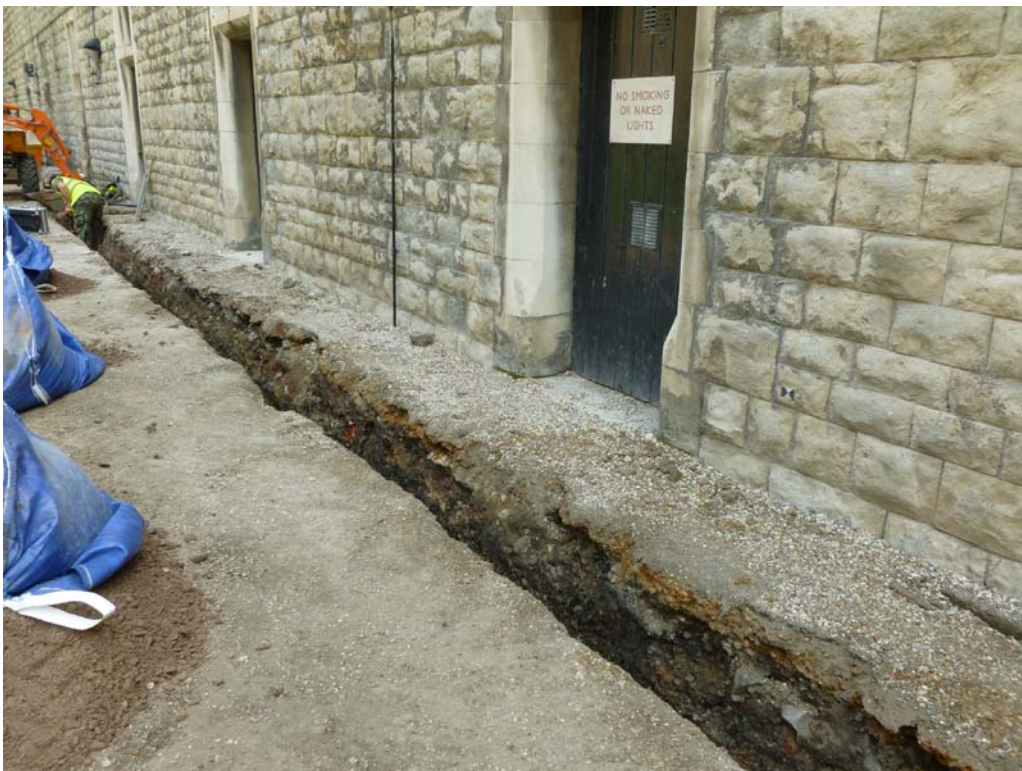
Plate 2: View NE of Trench 1 under excavation
