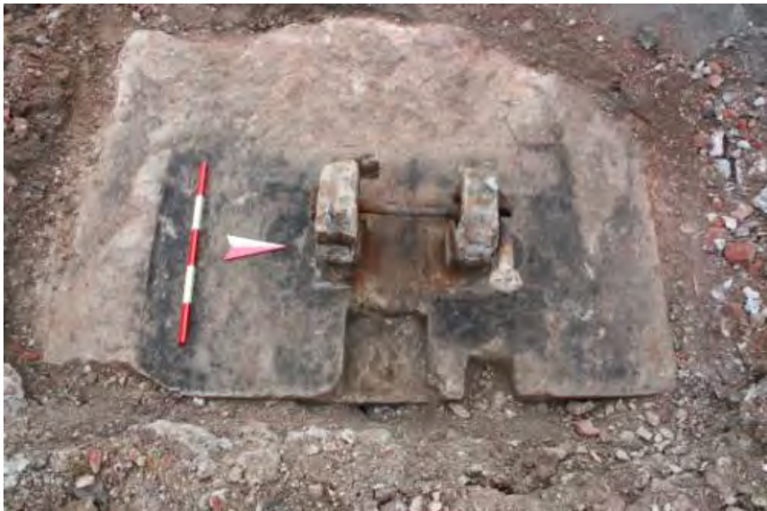
Plate 6. D.313/41. Penstock valve [137], North side Dry Dock No. 3, adjacent to Dry Dock No. 4. Scale 0.5m looking W.
