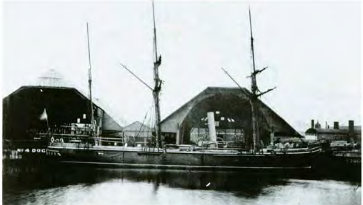
Plate 22. Photograph taken 1872. Looking E towards Dry Docks Nos. 4 and 3 (3 on the right) showing timber sheds built over the docks. [145] may be corner foundation for posts supporting this structure.
