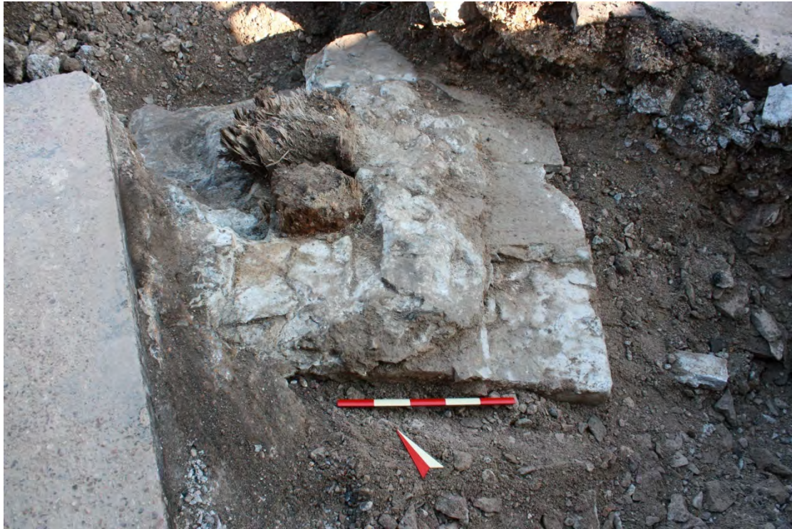
Plate 21. D317/23. Stone foundation [145] with truncated timber posts in-situ. Scale 0.5m looking NE. Believed to be the foundations of a timber framed building constructed over Dry Dock No. 3 in the 1870s. Possible that [141] (above) is a similar feature?
