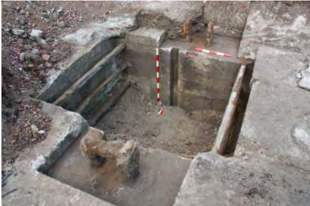
Plate 5. D.312/23. Penstock valve [132], North side Dry Dock No. 3, adjacent to Dry Dock No. 4. Scales 0.5m & 1.0m looking NNW.
