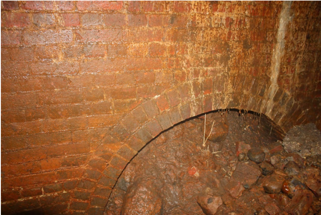
Plate 16. D316/41. [142] Sewer. Backfilled culvert in main southern wall. Looking S.
