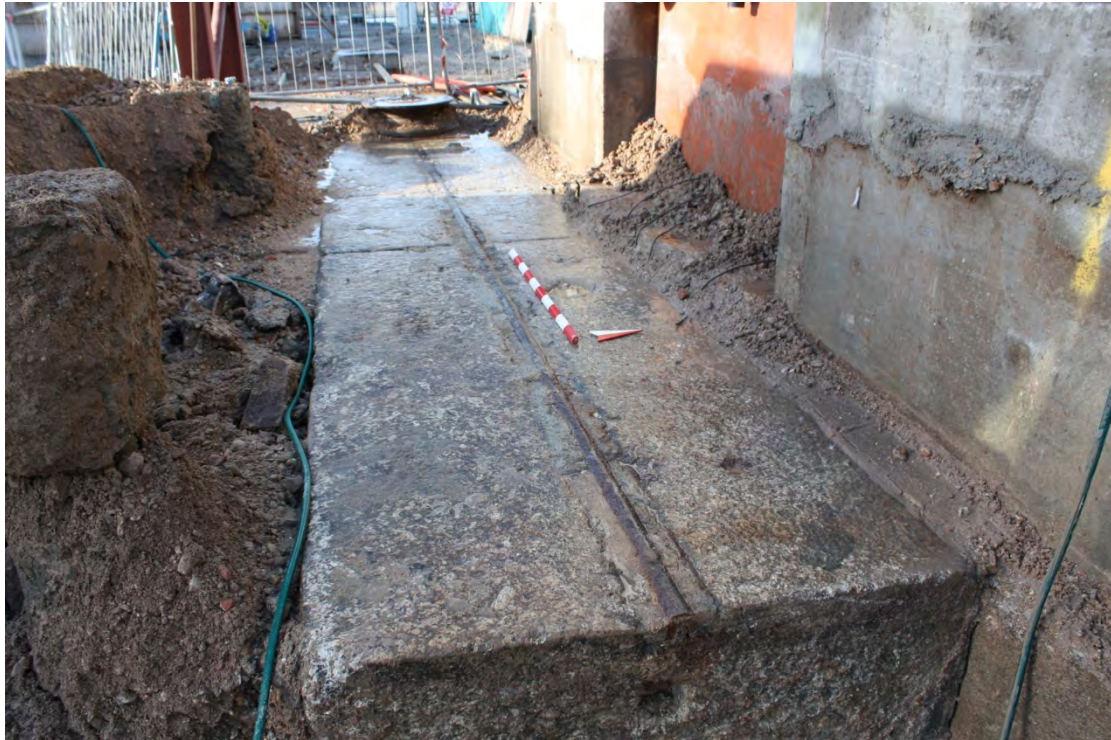
Plate 13. D300/96. 1920s outer facing dockside crane rail, south side Dry Dock No. 3. Scale 1m looking W.
