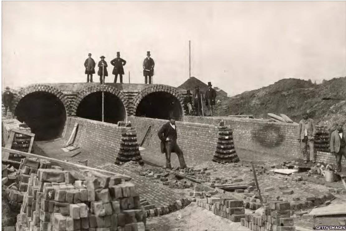
Plate 19. Joseph Bazalgette's northern outfall sewer, London, c. 1860s. Compare with Plate 17 above.
