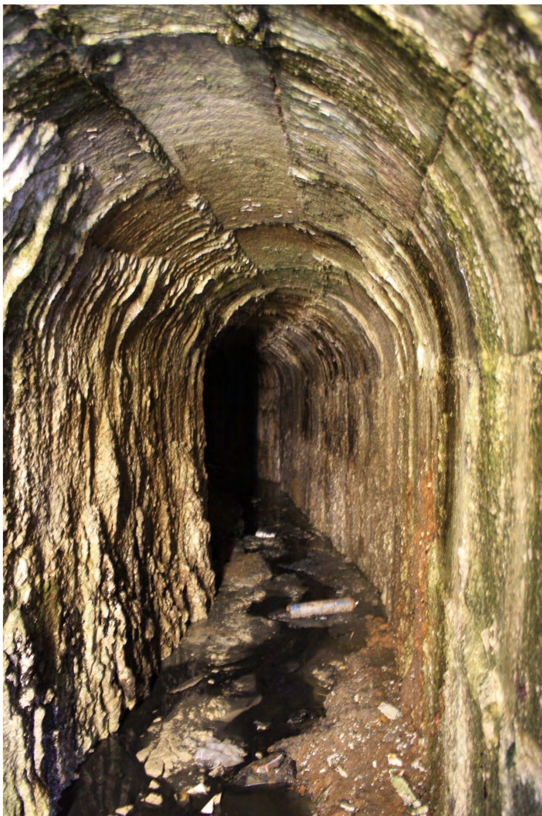
Plate 12. D305/85. Internal view of culvert [108], c. first 5m in. All of the culvert is built from Portland stone blocks as illustrated here. Looking N.
