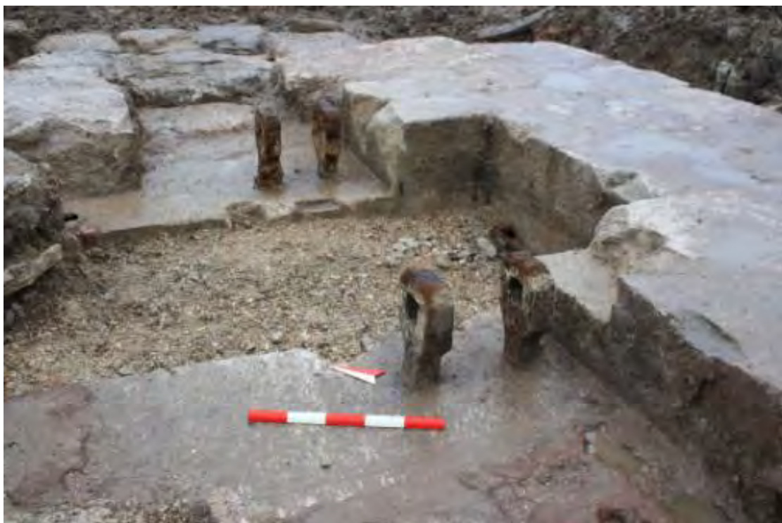
Plate 4. Penstock valve [37], North side Dry Dock No. 3 found in January 2010 (PMRP08 Phase 3). Scale 0.5m looking NE. Compare with Plates 5, 6 & 7 below.
