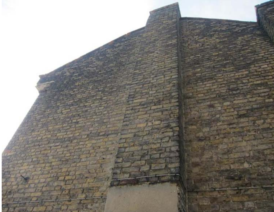
Plate 7: East elevation of 190 Warham Street, showing south chimney stack, with cement render and horizontal scar indicating former location of roof of 188 Warham Street, looking south-east
