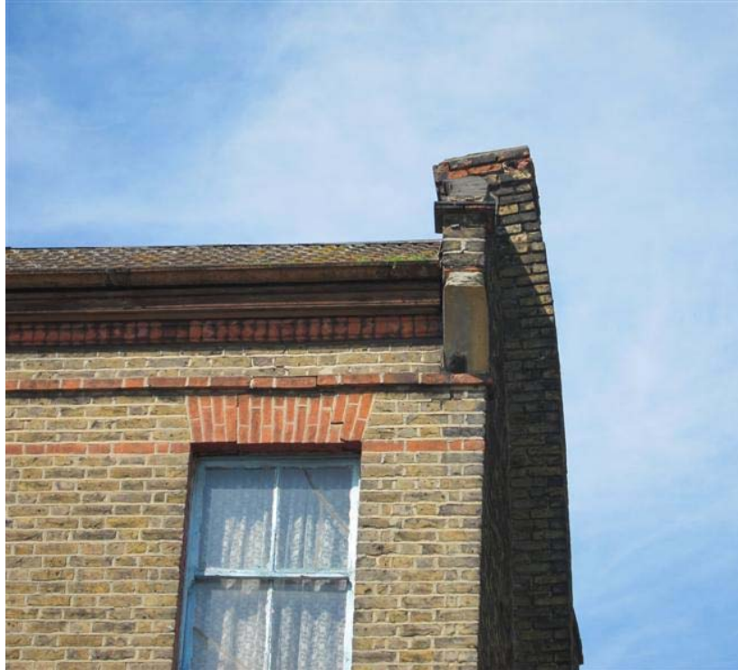
Plate 3: Second floor window of 190 Warham Street, showing decorative brickwork and bowed south chimney stack, looking north-west
