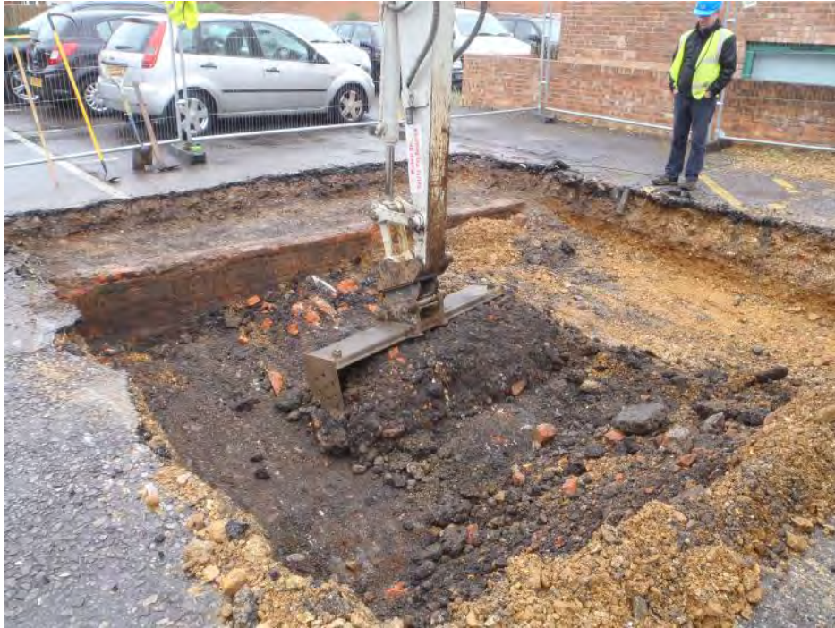
Plate 1: TP2 - looking north east during machine excavation
