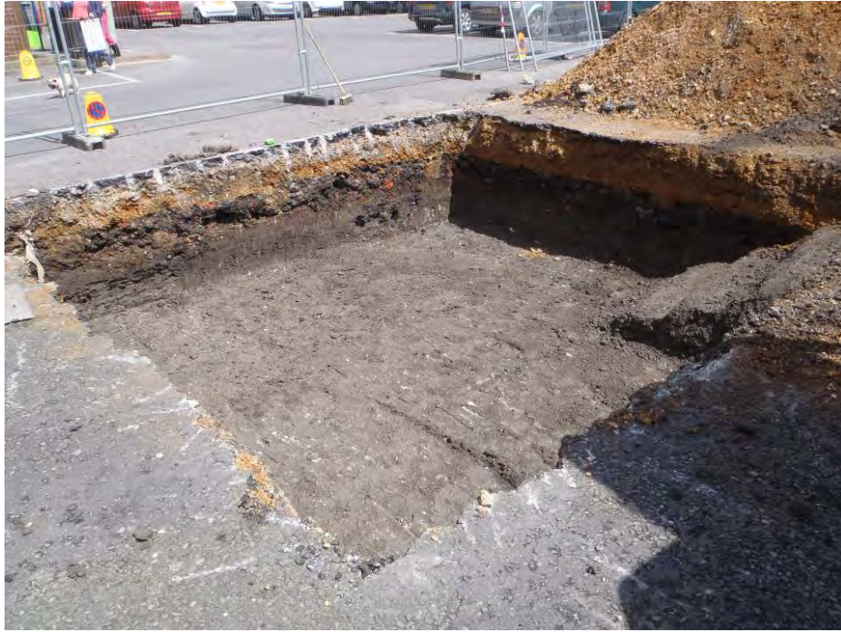
Plate 3: TP1 - View looking north east showing reduced dig to 1.2m BGL
