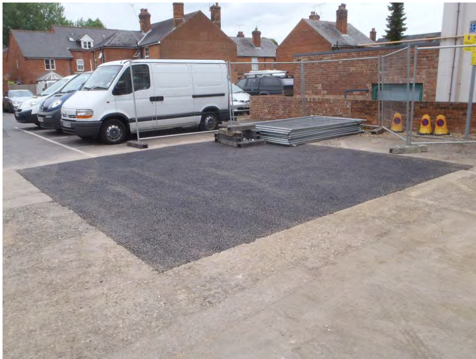
Plate 12: TP2 – View looking north east showing reinstated car park surface
