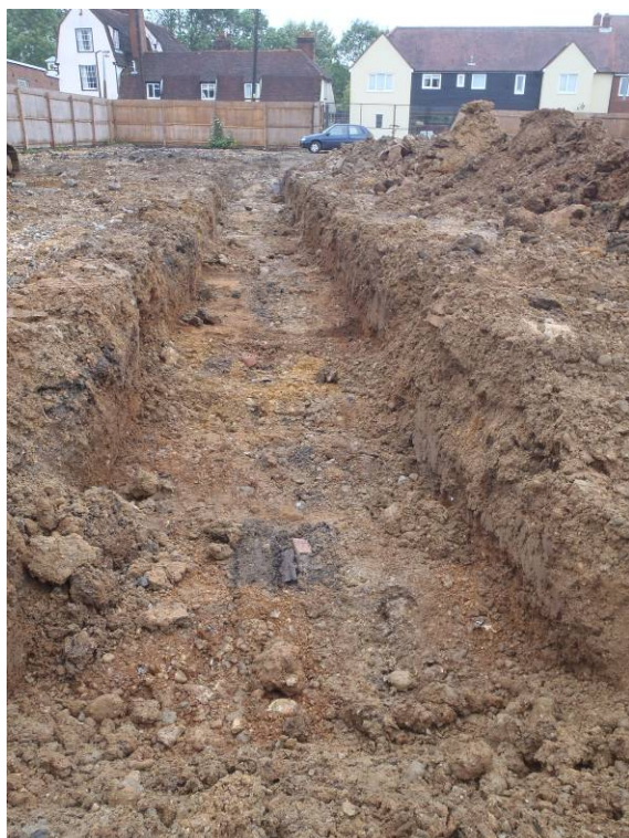
Plate 3: Trench 2 looking southwest
