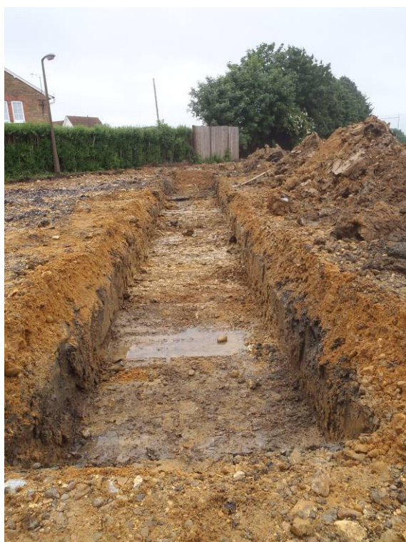
Plate 4: Trench 3 looking north
