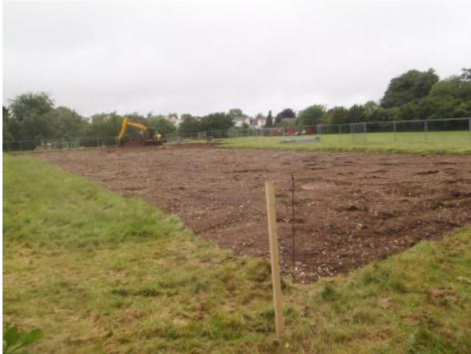
Plate 1: View of the Site looking north-west during topsoil strip
