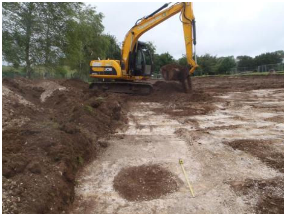
Plate 6: View looking west of Pit 5, pre-excavation
