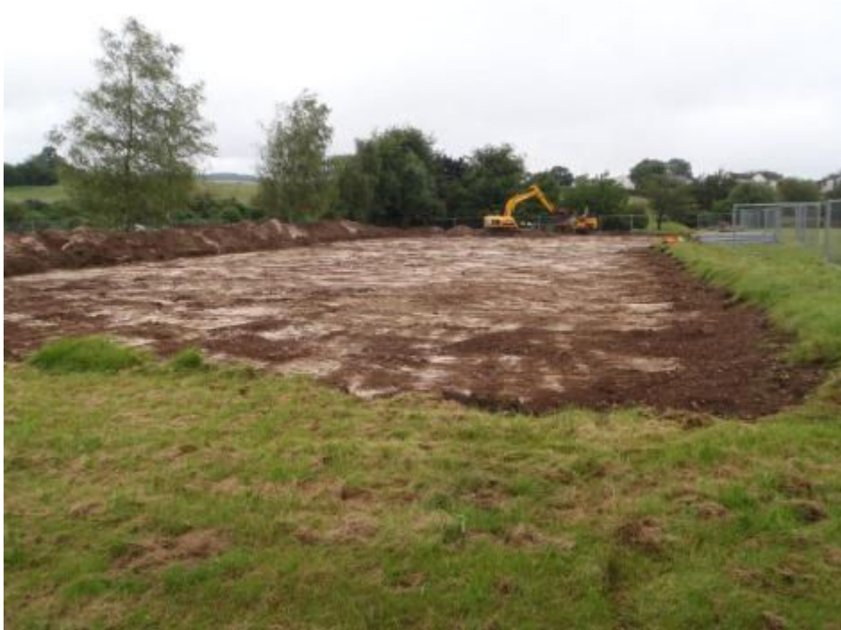
Plate 3: View looking west showing exposed natural chalk
