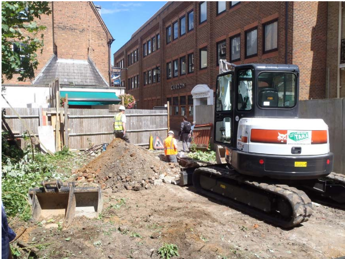
Plate 11 – General view of ET 2 under excavation facing east
