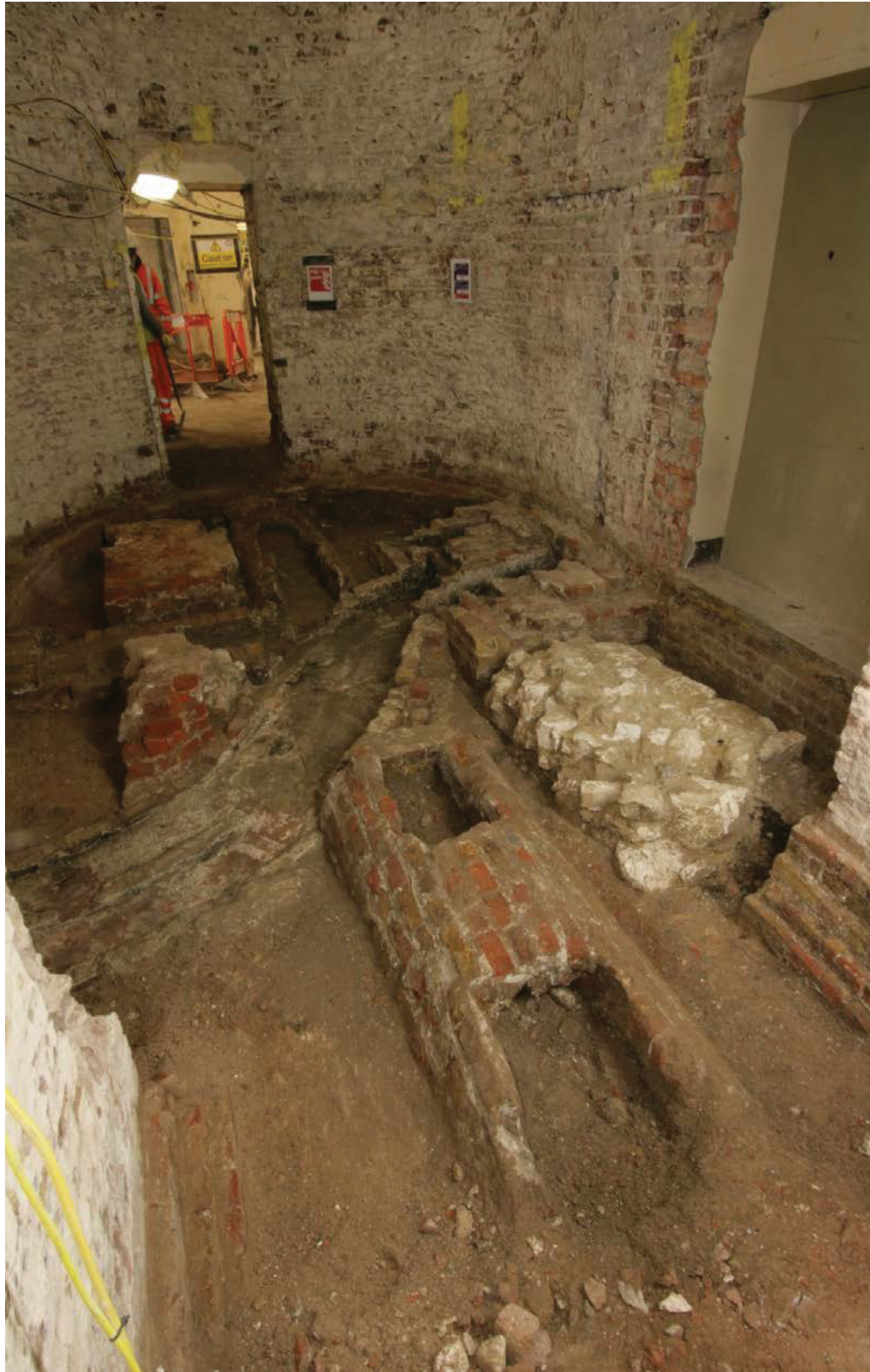
Plate 11: Multi-period activity in Lightwell 1; chalk foundation [191], Tudor brick walls [192] and [193], late 18 th -century brick drainage culverts [189] and [190] and 19 th -century brick flue structure [198], facing south
