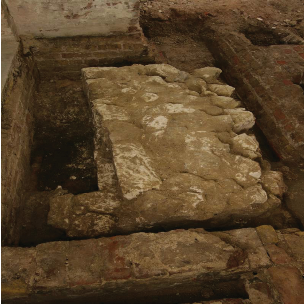
Plate 12: Chalk foundation [191] in Lightwell 1, facing northwest
