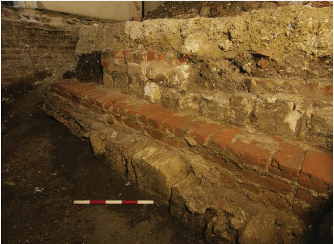
Plate 7: Brick and masonry wall [171], [172] on masonry rubble foundation [173] in Room B60, facing south
