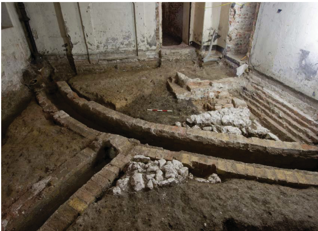
Plate 6: Chalk foundation [124]/[127] and masonry foundation [125] truncated by late 18 th -century brick drainage culvert [124] in Room B47, facing northwest
