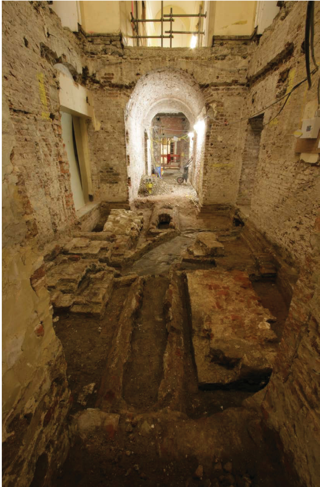
Plate 10: Multi-period activity in Lightwell 1; chalk foundation [191], Tudor brick walls [192] and [193], late 18 th -century brick drainage culverts [189] and [190] and 19 th -century brick flue structure [198], facing northwest
