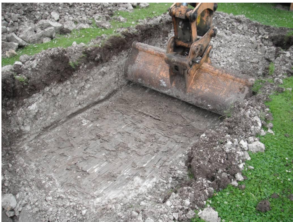
PLATE 8: Trench 3. Machining onto layer (16), buried under chalky made ground (15).
