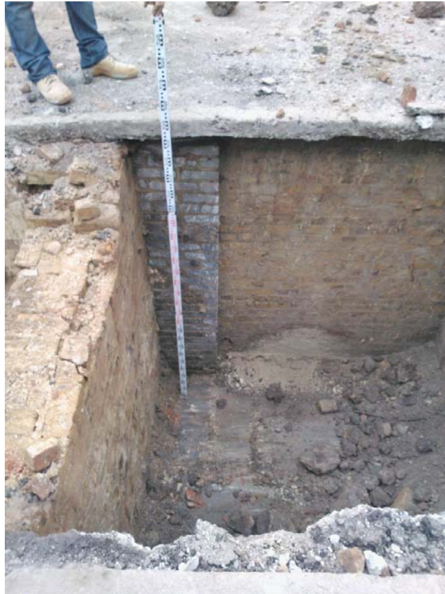
Plate 8; Sondage at east end of Trench 3 revealing basement slab.
