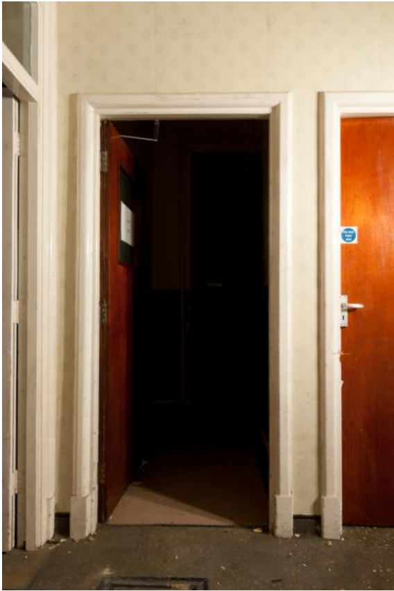
Plate 13 Original Door Architrave
