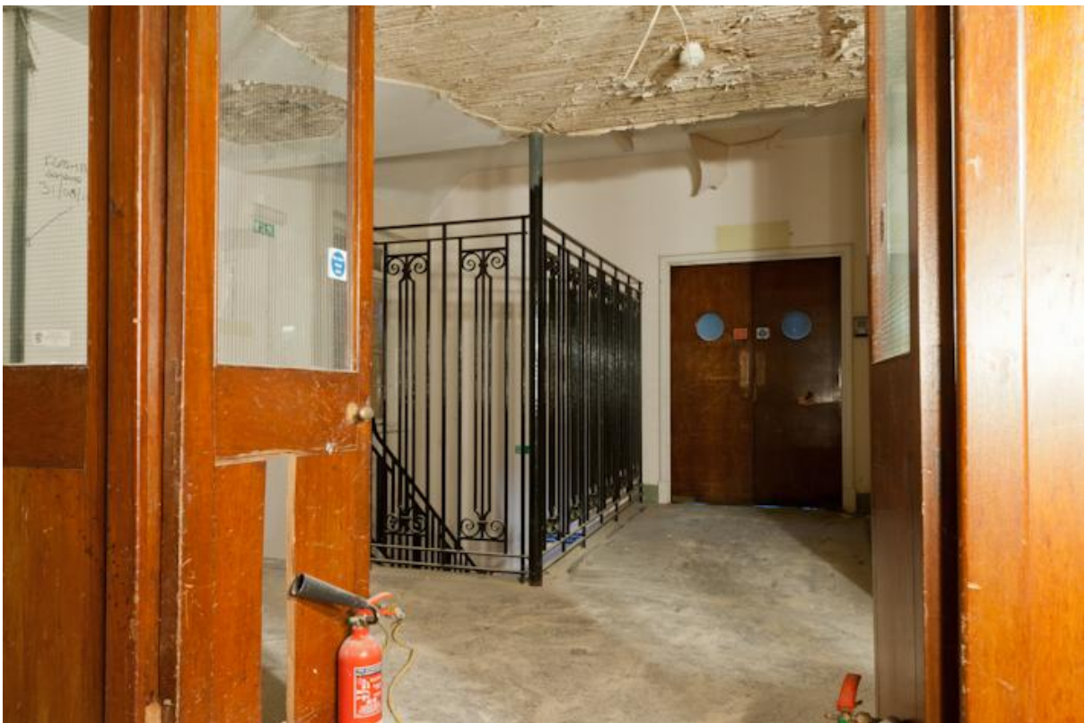
Plate 16 First Floor Landing
