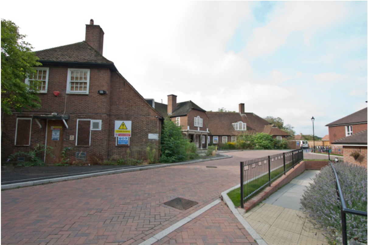
Plate 3 Northern range end bays looking south-west
