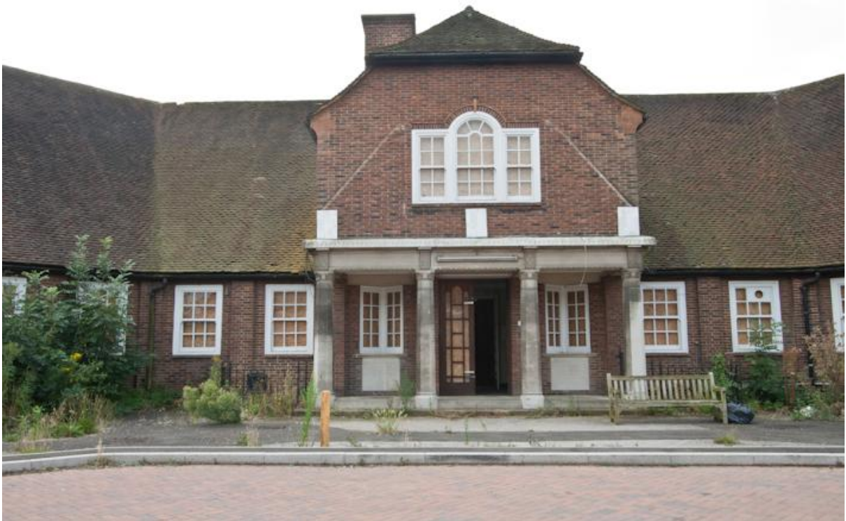
Plate 2 Central Entrance Bay, looking south
