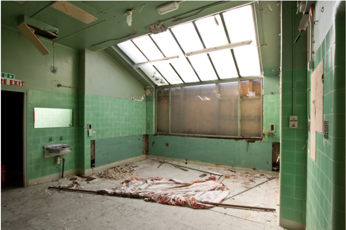
Plate 9 Theatre (G6) with north-light roof
