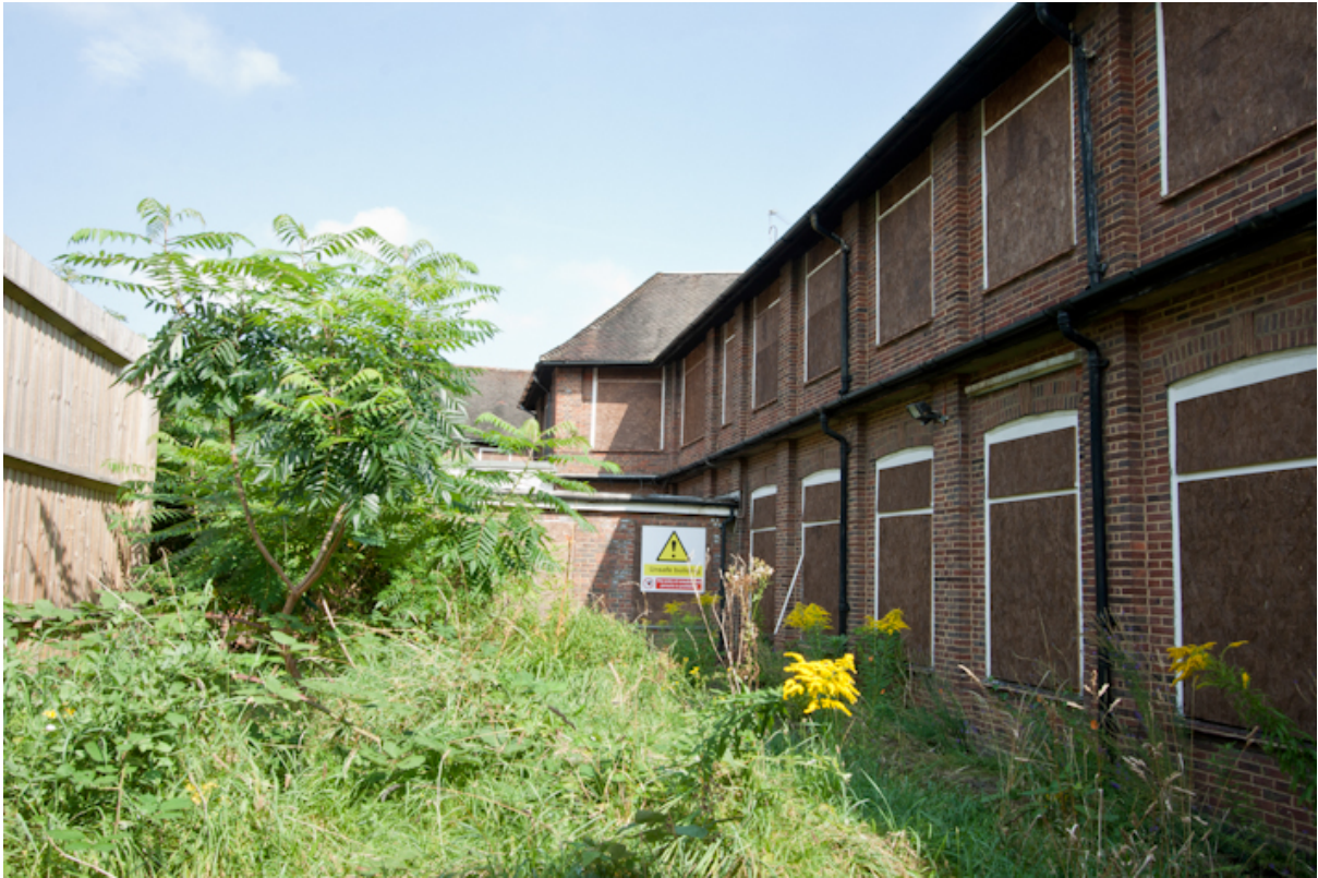
Plate 5 Central North-South Ward Wing (Mallison/Passmore) Looking north
