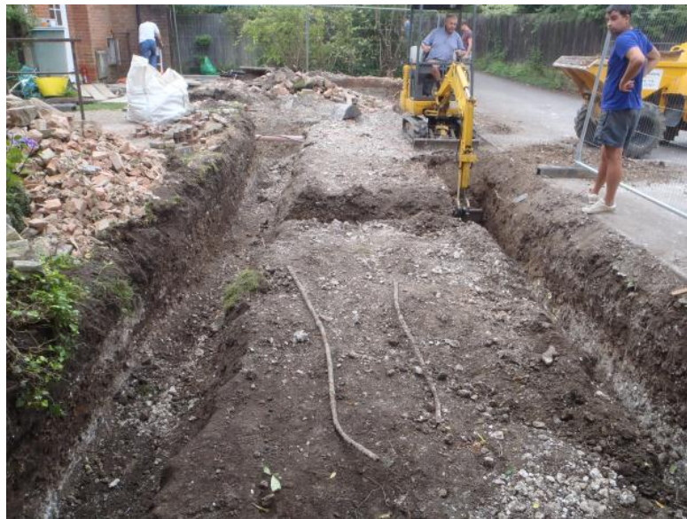
Plate 5: View looking north during excavation of foundation trenches
