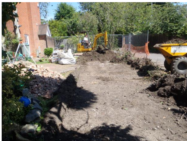
Plate 2: View looking north of reduced level excavation
