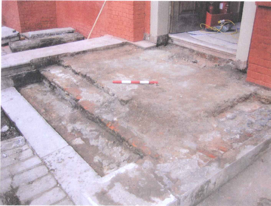
Plate 1: Floor tiles underlying stone pavoirs at the south entrance of Kew Palace
