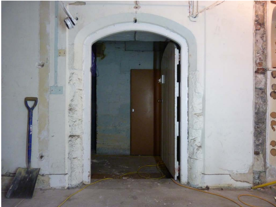
Plate 4: Door in North Wall of Room 37/38
