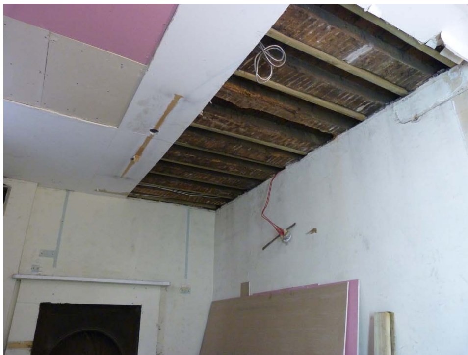
Plate 2: Exposed Joists in Northwest part of Room 38
