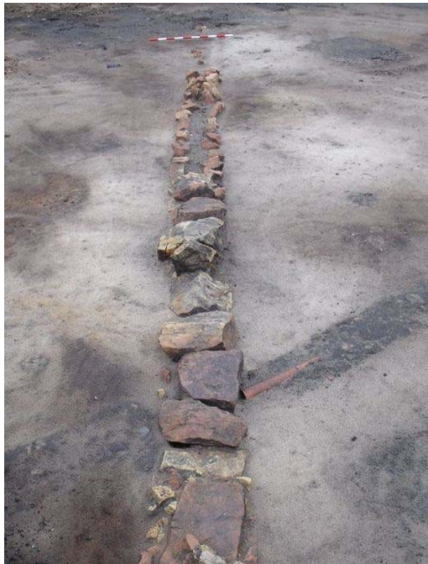
Plate 10: Trench 2, culvert [82], looking south-west (scale 1m)
