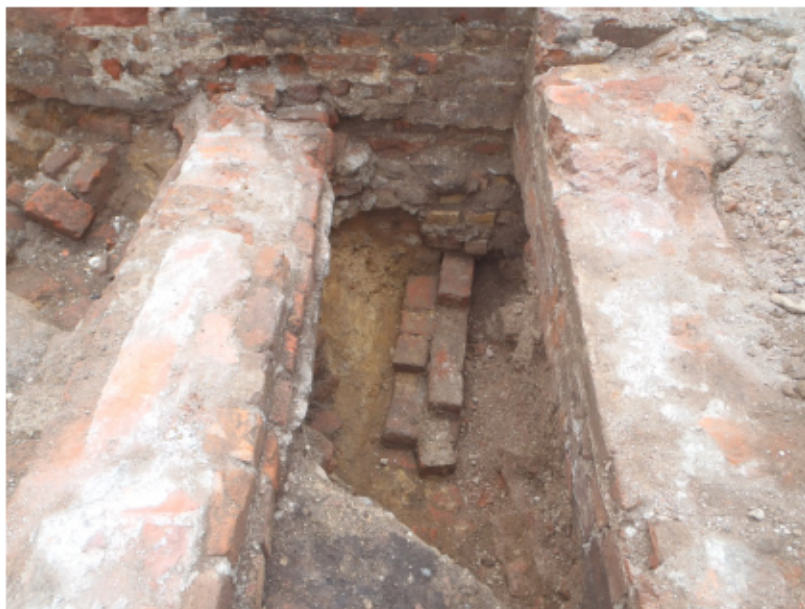
Plate 8: Wall [31] and wall [12] underpin, looking northeast
