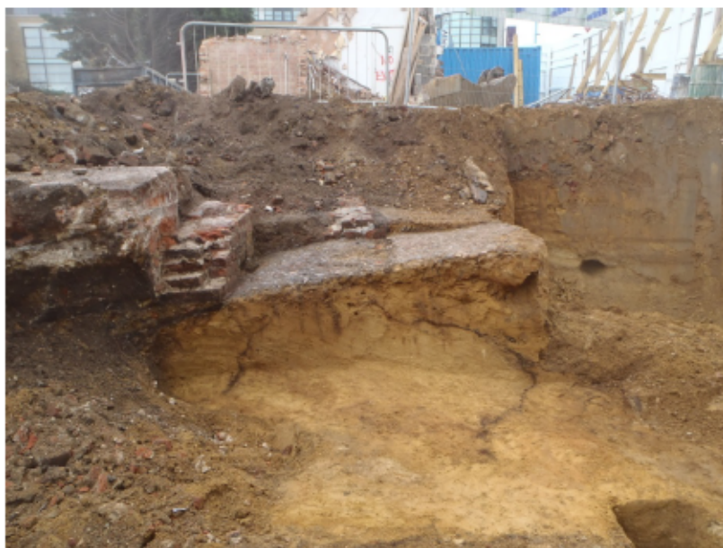
Plate 14: Section 5, showing gravel surface [17/38] and wall [29] looking west
